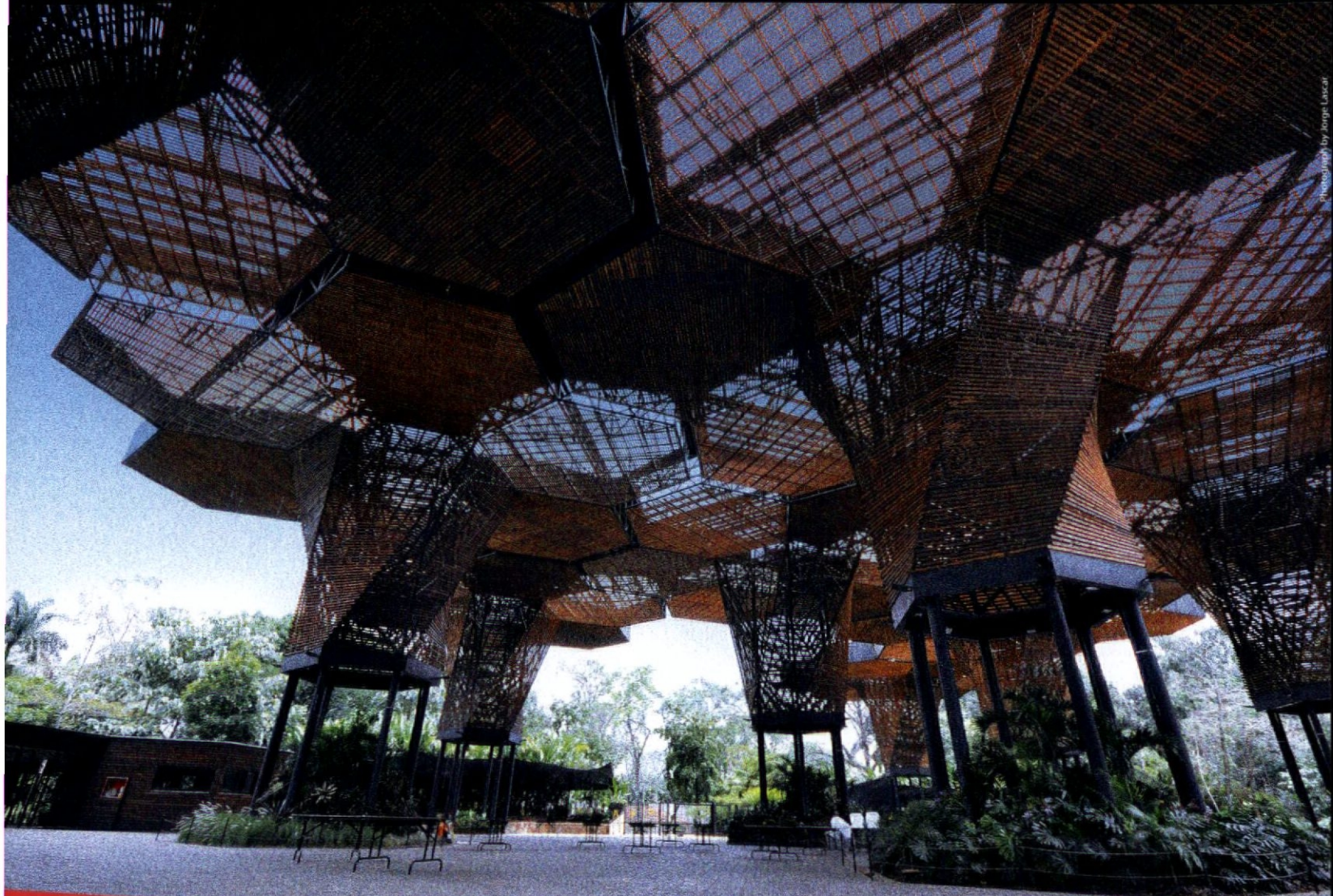
ABOVE: The Orquideorama, located in the Botanical Garden of Medellín, is a steel-framed canopy topped with glass and clad in wood strips to evoke a forest grove. Orchids grow at the base of hexagonal steel “trees,” and the space is used for events and informal gatherings.
