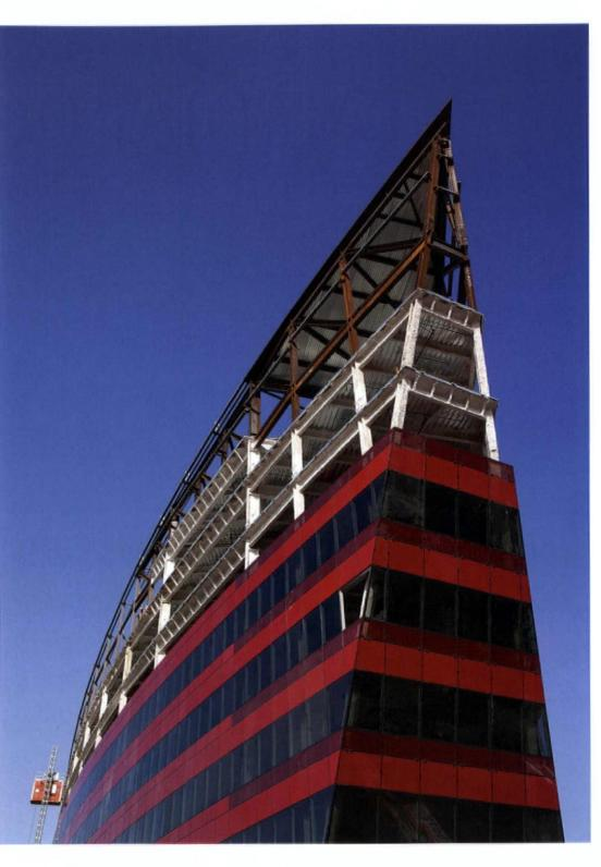
LEFT AND ABOVE: Pelli made modifications to his design but kept the red façade intact. Sheets of glass were made in China, put into aluminum panels in Thailand and positioned to suggest a curved surface.
