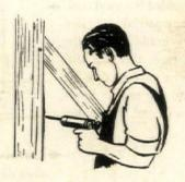
Half-timbered walls of brick or stucco suffer from shrinkage of the timbers which produces open cracks where they meet the masonry. Caulking with a fine nozzle will fill the openings. The timbers should be dressed with linseed or tung oil which will preserve them and prevent further shrinkage. Loose pieces of stucco should be cut out and replaced with new patches of cement.
