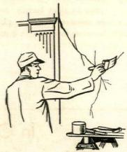
Stucco walls that show map or hairline cracks simply need a wash of neat cement. This should be brushed in so as to fill the cracks and the excess wiped off with burlap or rough cloth. Heavier cracks should be cut out, well wet and filled carefully with a mixture of two parts sand and one part of Portland cement.
