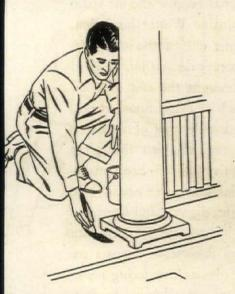
Porch columns need particular attenion at the point where the base sets on he platform. Care should be taken to see that paint is brushed in underneath
