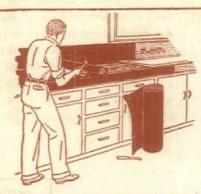
The first step is to cover the wood counter and backsplash with heavy waterproof paper as is shown above
