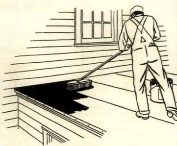
Heavy roofing paint should be brushed on at least every two years. Flat metal roofs, subject to rust, require more attention than any other painted surface of the house. The surface should be examined for small pits or rust spots
