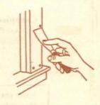
Putty all cracks and nailholes with good linseed oil putty or white lead
