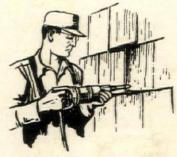
Warped shingles are the first indication of trouble in a shingled wall. If the warp is so great that there is danger of splitting the shingle by nailing it back into place, small holes should be drilled as shown in drawing and the nail passed through it and driven into place. Use only galvanized nails.
