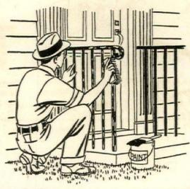
Iron work deteriorates very rapidly unless it is well protected with paint. All rust and scale should be removed with a wire brush before the new paint is applied. Paint particularly intended for metal work should be used
