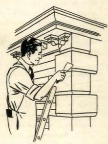
Under-eave areas don't have the chance to dry as well as surfaces exposed to the sun. Cracks in the wood-work should be filled with putty and all defects repaired
