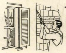
Window frames which are set into masonry walls should be caulked so that the joint is completely filled with caulking compound or mastic. Rot and disintegration progress rapidly during damp or rainy weather. A caulking gun with a fine nozzle is probably the only tool required. The joint should be struck off smooth and even with the wall that surrounds it after caulking is finished.
