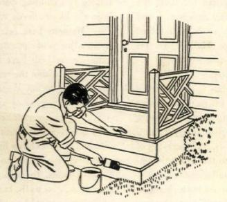
Wooden steps and platforms are subjected to severe service from both traffic and weather. Paint should be brushed in particularly well on the step nosings. Treads wear better if painted annually
