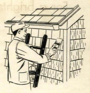
Shingled walls will absorb less moisture, and the shingles will last indefinitely if they are painted frequently. Painted, oiled or stained shingles seldom warp or split from weathering
