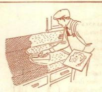
Metal lath is placed over the waterproof paper and a rough coat of cement is trowelled on
