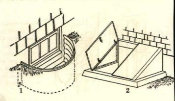
Rust-proof metal shields (1) are now designed to form a well for basement windows. Cellar entrance doors (2) in a neat assembly can be built in without fitting. They are made of rust-proof metal, the hinges are on the inside and the bolt ensures safety. This unit is entirely prefabricated and ready to install as soon as it is received on the job
