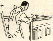
The top of a door frame is a favorite place for moisture to enter and cause wet walls and interior discoloration. The joint between the flashing or lower row of shingles or clapboard should be well filled with caulking compound. This should be carried down as well on both sides of the door frame if any cracks should exist at those points.
