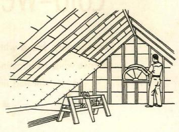
The unfinished attic may be responsible for the loss of as much as 30% of the heating energy supplied by your boiler. Insulating board properly applied to the underside of the roof rafters, or over ceiling, reduces losses to a minimum. Ventilators or attic windows should be provided to carry off both hot air and air-borne moisture
