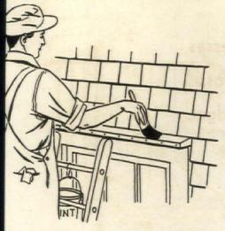
Metal flashings, unless rust-proof, should be painted annually. Even though they are made of rust-proof metal they will benefit by he paint and be less liable to corrosion
