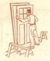
The first step in preparing the door for weather-stripping is to remove it from the frame and lay it on its side for the planing.
