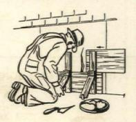
Defective clapboard can be readily cut out with a key-hole saw if the board above is wedged up on both sides of the split. The butts of the boards on both ends of the new piece should be securely nailed in place and then painted to prevent future warping.
