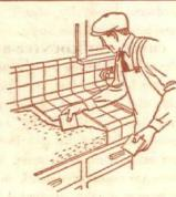
The tile is set in a second coat and each tile is squeezed securely into place in the mortar
