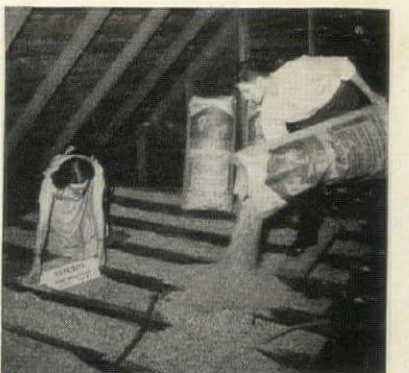
MARY SMOOTHED-OFF the Zonolite with a common board as fast as John emptied each feather-light bag between the attic joists. Time: 3 hours.
