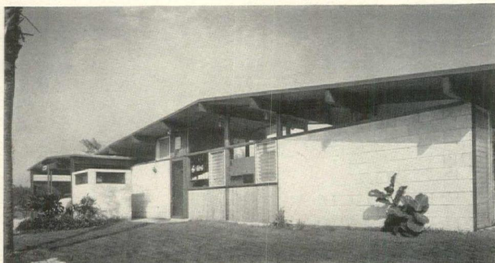
**The service side of this small house** shows you a close-up of the lime-block walls. Since this material is porous and hollow, air can circulate through it and keep the house cool. Notice the glass jalousies and glass panels above which give the kitchen light, air, and a view of outdoors.
