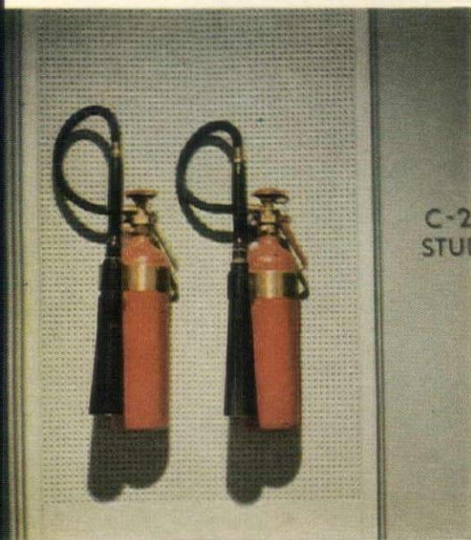
**FIRE EXTINGUISHERS** are near fan rooms, sound, and recording booths, have red metal and brass cylinders, black discharging horns attached to rubber tubes.
