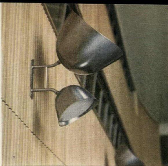
**LIGHTING FIXTURES** in Trusteeship Council Chamber are set in wall of ashwood slats backed by Fiberglas matting to absorb sound. Larger unit throws light on unusual pattern of ceiling shown on the right.
