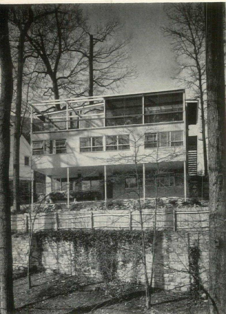
You enter the ground floor from the back garden, where the children have a fenced play area. Because site slopes so steeply, the center (bedroom) floor rests on a series of steel columns.
