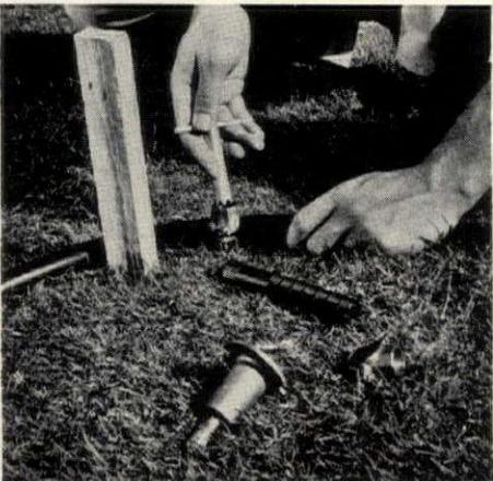
5. Once pipe lines are laid out on the surface, taps are quickly made at required locations to receive branch T's of sprinkler heads.
