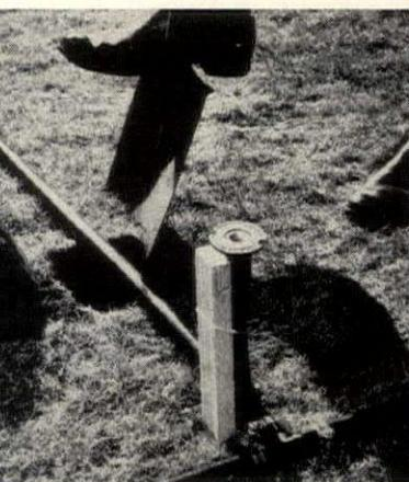
When pipe is laid, all lines connected, and heads properly attached, the setup should be tested before trenches are opened.
