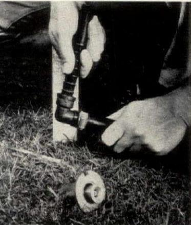
Plastic pipe is easily cut with a strong pipe cutter and special angles and connectors can be placed and replaced as required.
