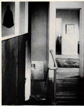
Gallery-effect stair landing was made by removing old bearing partition and replacing it with posts and parapet wall.
