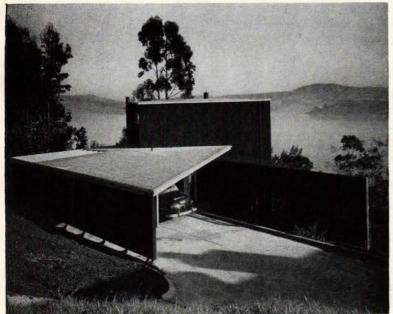
Driveway from street, left, descends to angular carport which has storage cabinets for equipment, partly louvered roof for laundry drying yard at rear.
