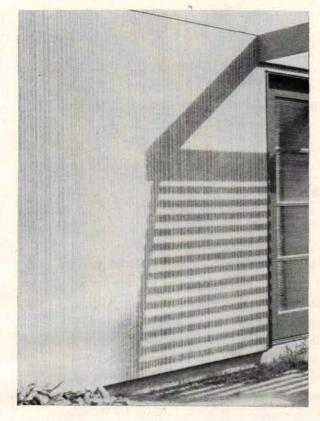
No feature of the new houses interests other builders more than the \(^1\ge\)'s" sheets of asbestos cement that form exteriors. Eight feet high x 32" wide, they butt together with an almost invisible crack. Produced in seven colors, vertical lines seem to be striations. At gable ends, top panels lap over bottom panels. Prepunched nail holes speed installation, let carpenters nail through into studs.
