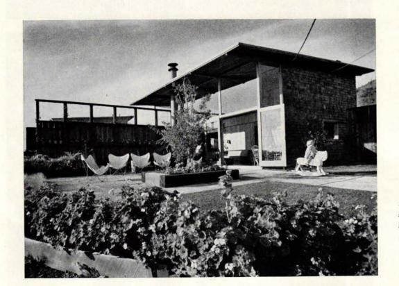
Full-height plate glass wall with simplest possible framing provides light, view and ventilation for the entire interior:
