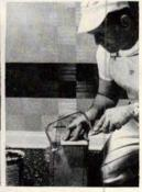
square is dabbed with mastic and pressed into place so none of the binder oozes through the seams. (Not a waterproof system, it is not recommended for use in baths or kitchens.) Retail price, not installed, is about 60¢ per sq. ft. The finished wall may be washed clean, dusted with a brush or vacuumed. Colors, which go beyond the familiar pastels to include a deep blue green and coral, are permanent, and the material is said not to chip, peel, or crack.
