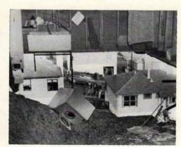
IN SOUTH SAN FRANCISCO, a landslide undermined \$9,450 postwar home built by Sterling Building Co., let slab floor collapse, leaving a clothes washer dangling by its rubber hoses.
