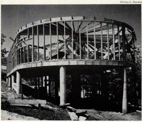
Though rafters are easily cut and set for wheel shape, some special cutting and fitting had to be done on peripheral framing members.
