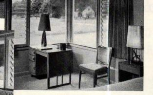
With louvres of glass or wood, these efficient modern windows provide not only a functional but a decorative unit for architectural design. They are used as standard window openings, as side vents for large areas of fixed glass, as porch and breezeway enclosures and as door panels.
