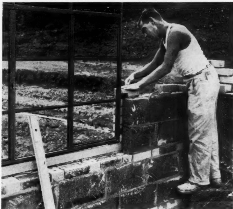
TWO CLIPS on side of frame help hold window firm while mason sets brick. Steel windows are so easy to handle, this workman couldn't spoil the job if he tried.
