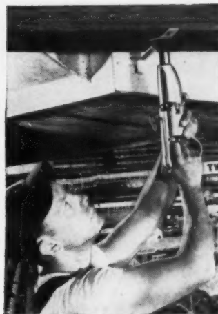
Hanging ventilating duct from concrete ceiling
