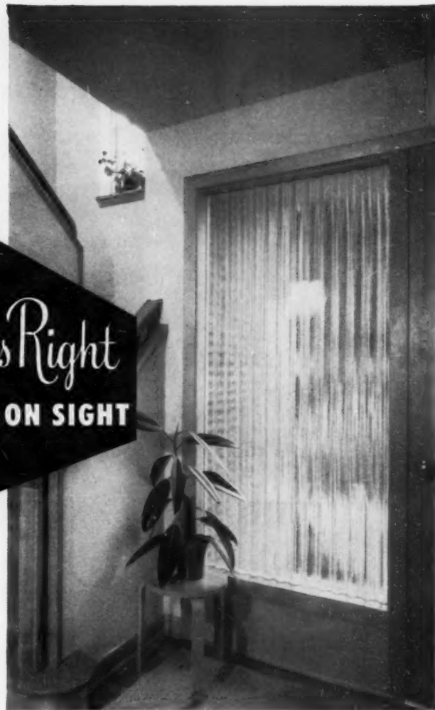
Structural Corrugated glass installation at main entrance of L. M. residence in Seattle, Washington. Architect, Gerhard E. Karplus, New York City.
