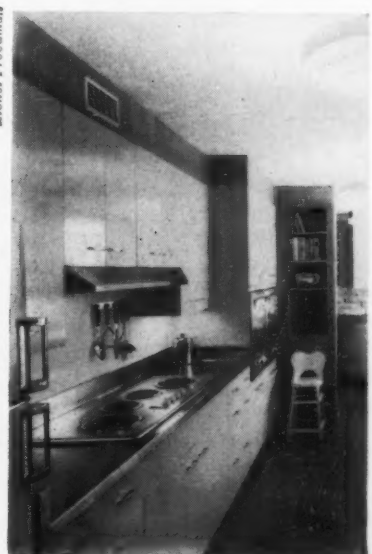
The ventilation problem, more urgent in open kitchens, can be solved by a hood and fan directly over burners, secondary intake near ceiling. Architect: A. L. Aydelott.
