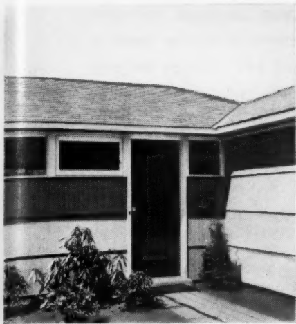
Ready-cut \frac{3}{8} " Weldtex siding like this in strips 48" by 15 \frac{7}{8} " can be used where a dramatic horizontal effect is desired. It is easy to install in shingle style, but goes up faster than shingle-size pieces.
