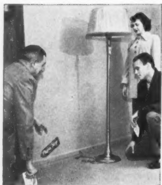
Plug-in strips are economical, permit free furniture placement. Lamps may be turned on or off directly or from central wall switch.
