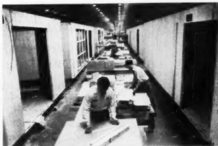
UTILITY CORE , one of three units that make up the house, carries all plumbing and appliances. Ductwork for blower furnace extends into all sections. Roof is designed for 30 lb. snow load.
