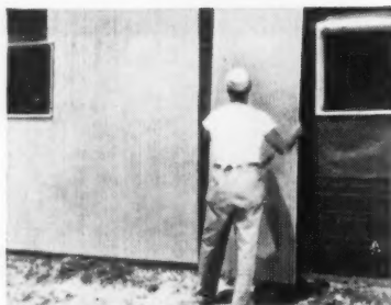
One man can handle and place with ease a full-size sheet of Colorbestos. Nail holes are pre-punched.
