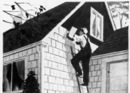
• Nova Insulated Roofs and Sidewalls. Sheathe, shingle and insulate in one operation. Give double-coursed effect.
