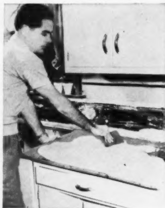
PLASTIC COUNTER TOPPING applied with glue and rolling pin
