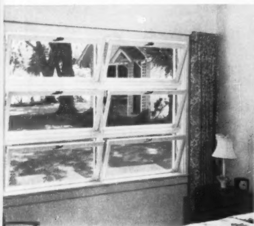
1. HOPPER-VENT —Sash swing inward with Flexivent in this position. Screen on outside means easiest operation. Note ample ventilation, yet no interference with drapes. Good protection during rains. Use hopper position for very low or very high ventilating windows.
