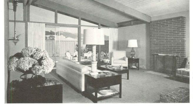
Heavy beams of dor  $2'' \times 12''s$  with plank:  $T\&G 2'' \times 6''s$  are charteristic of all Terra Li houses. Over the cei is 1/2'' of glass fiber, the built-up roof topped volight-colored gravel.
