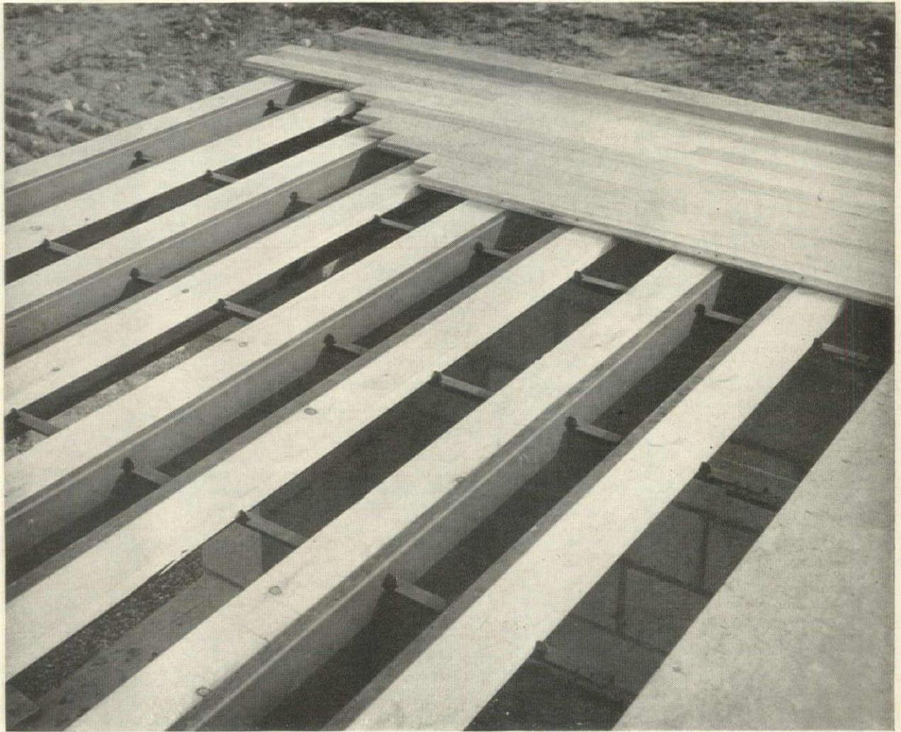
**STEEL FRAMING** system by Webcore (Cessna Homes) is a series of grid sections formed from four 16 ga. steel joists locked together by traverse support angles. Wood
