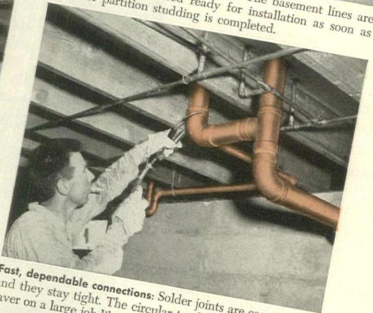
**Fast, dependable connections:** Solder joints are easy to make and they stay tight. The circular torch shown is a big time saver on a large job like this. (Water lines are also copper.)
