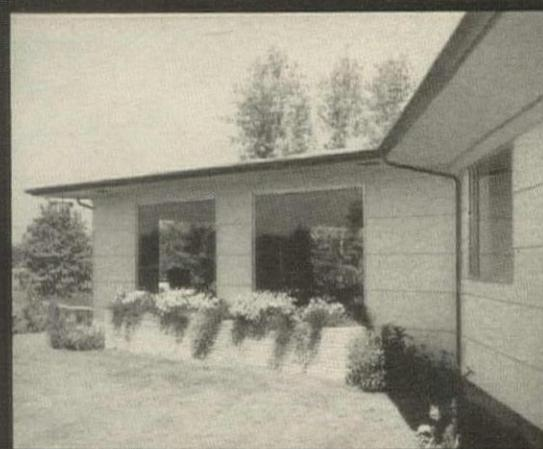
**PLYALOY OVERLAID PLYWOOD** provides the finest and most durable paint base of any siding on the market today. It takes paint easily, evenly. Eliminates grain raise and checking. The smooth, durable overlay is a medium-density resin-impregnated fiber permanently fused to Exterior fir plywood in modern hot-plate presses. Pre-cut to standard 12", 16" and 24" widths; 8' long; lower edge beveled for drip. Comes packaged by the square, complete with wedges and shadow-line furring strips.
