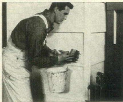
for lamination with the individual wood plies. The resulting surface takes paint better than wood and holds it longer, yet can be worked, glued or fastened like any ordinary plywood. In interior use, the plywood can be used in kitchens, bathrooms or laundries, because the plastic surface cannot be delaminated by moisture or heat.
