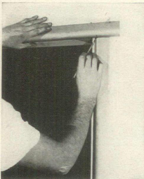
**STEEL CASING** for window and door openings (Scholz) snaps into a saw kerf in the jamb, needs no nailing. Bullnose shape prevents damage to pre-applied trim. Manufacturer: US Gypsum Co.
