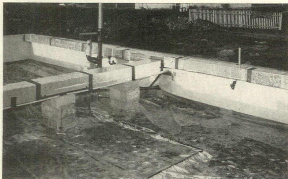
**GLASS FIBER DUCTS** are integrally insulated, and have good sound deadening properties, especially important in forced air systems (Scholz). Perimeter ducts are strapped to the foundation wall just below the plate line. *Fiberglas* sheets are shipped flat, folded into rectangular ducts on the job, and joints are sealed with pressure-sensitive tape. Manufacturer: Owens-Corning Fiberglas Corp.
