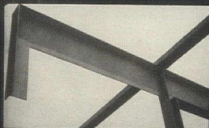
**Steel sunshade** can be suspended from cantilevered girder and faced with standard steel decking, as in this detail from Quincy Jones' own house. Note another kind of integral roof gutter, in this case a simple steel channel laid on its side. Architects: Jones & Emmons.
