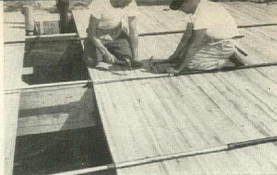
Installed planks eliminate subflooring
