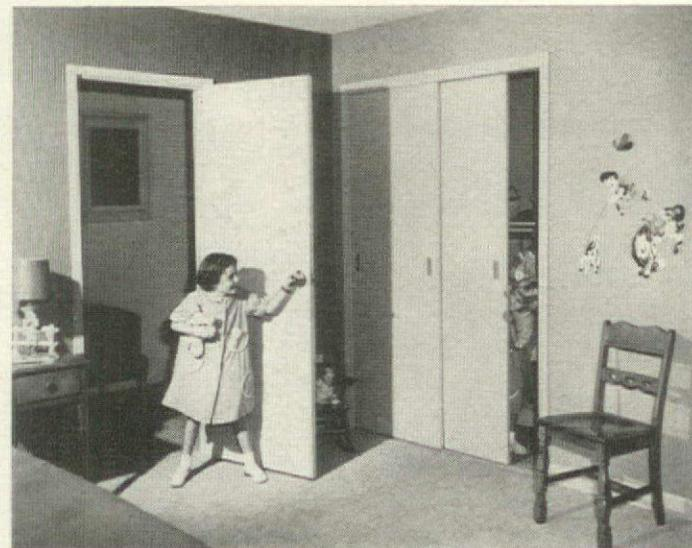
**STEEL DOORS**, mounted in steel frames (US Steel Homes), are mortised for hardware at the factory. Swinging and sliding doors used are pre-primed, and sound deadening and reinforcing eliminates any "tinny" resonance. Manufacturers: United Steel Fabricators & Steelcraft, Inc.
