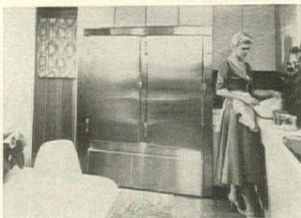
**m. REFRIGERATORS and FREEZERS can be built in, with compressor in a remote location**
