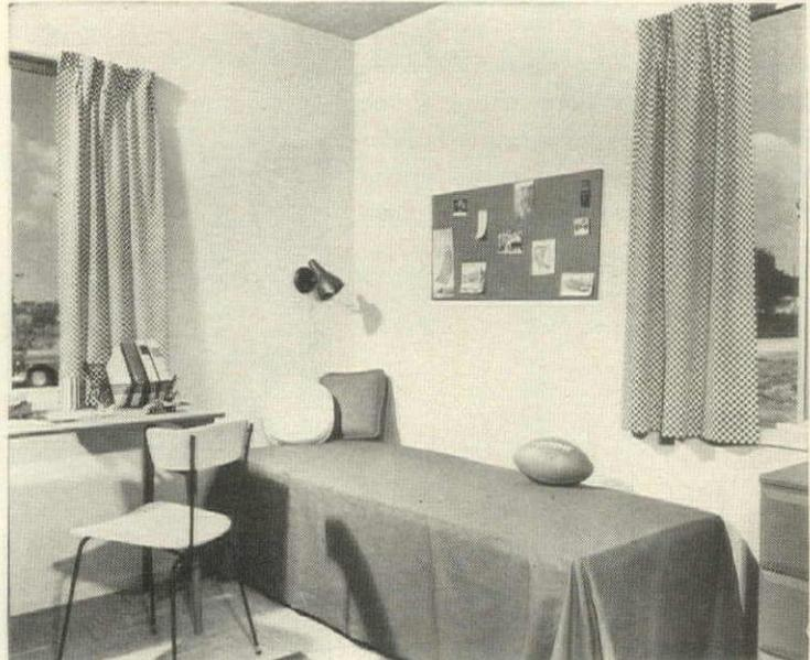
**Flat, smooth** wall surface is result of tape over gypsum
