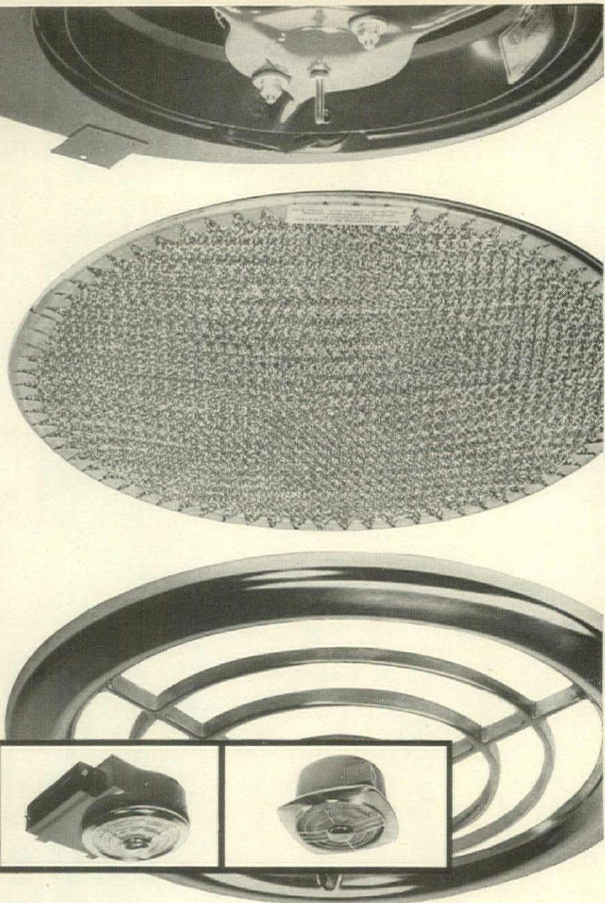
Multiple-mesh filters now make Pryne Blo-Fans and Aerofans even easier to clean — more popular than ever before! Simply snapping in behind the grill, the washable filter keeps blade and motor cleaner... guards against hazardous accumulations of grease in the flue!
