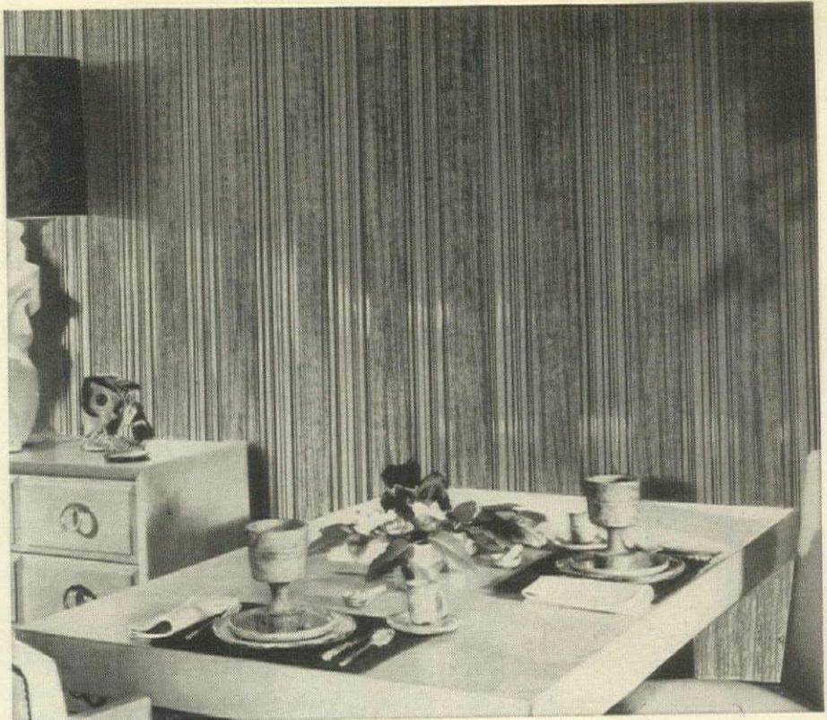
**PLANKTEX®** alternates bands of striations that contrast with the smooth pattern of the wood grain. Made of pre-finished Philippine Mahogany, Planktex comes in 4' x 8' panels, 5/16" thick. Fine for a dining area wall, over the fireplace, or in an entrance hall. Panel a 12' x 8' wall for about \$47—less if you choose unfinished Planktex.
