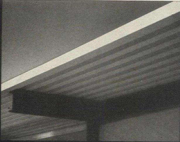
**Steel framing combined with fluted steel decking** makes 2-way cantilevers simple, thus permits roof overhangs on all four sides of house. Neatly integrated roof gutter makes usual fascia and gravel stop unnecessary. Architect: Raphael Soriano.
