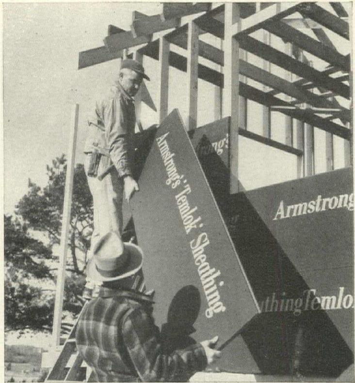
**Less waste** because Temlok Sheathing fits accurately over framework of studding 16" on centers. Temlok waste is only 5%, compared to an average of 20% with wood. There's no dimensional loss with Temlok—2' x 8' Temlok is full 24" wide, while 6" wood sheathing is only 5 3/4" wide.
