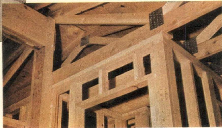
All structural lumber is No.1 and better, kiln-dried fir and hemlock. Structural strength is so great that all weight is supported on the outer walls, allowing freedom for interior changes without affecting building code requirements. Only proven, nationally famous products are used, including redwood prime-dipped siding on traditional models.
