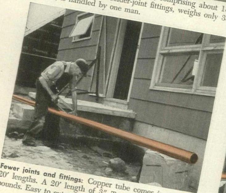
**Fewer joints and fittings:** Copper tube comes in standard 20' lengths. A 20' length of 3" Type M weighs only 53 pounds. Easy to cut, too.
