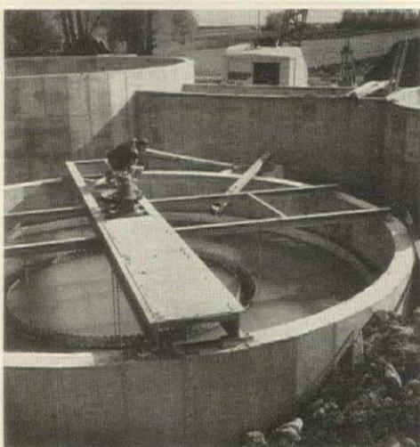
The agitator tank, shown in lower photo at left, is being used temporarily as a settling tank in this bio-filtration system until the whole plant is completed. Then sewage will go from the agitator to the two larger settling tanks shown at the rear. Part of the plant, in operation, is shown in the upper photo (left). Plant can now handle a population of 5,000, will later be expanded to take care of 54,000. Bonds will be retired through a \$100 tap-on charge for both old and new houses.
