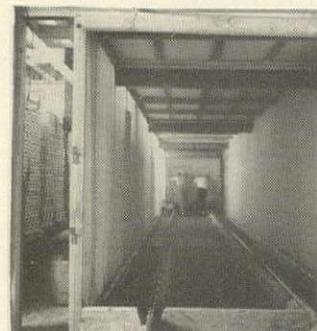
Doors pass through a complete conditioning cycle in special kilns.
