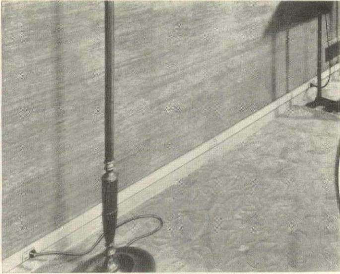
**CONTINUOUS ELECTRICAL STRIP** has outlets every 30", and can be installed last, so as not to delay other trades (Scholz). Wood baseboards can be routed out at the factory so that steel raceway is partly recessed. Couplings for interior or exterior corners permit the use of this raceway even in irregular rooms. Manufacturer: The Wiremold Co.
