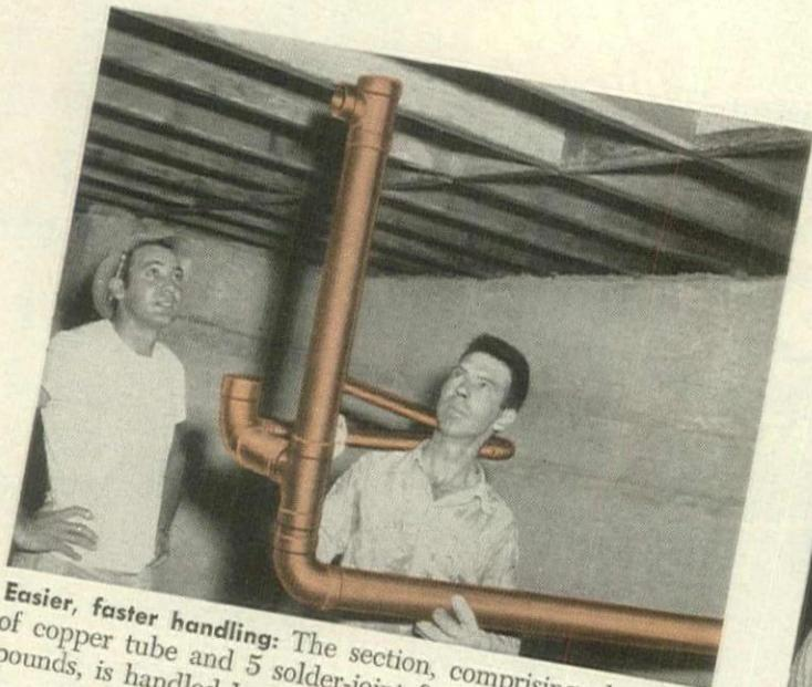
**Easier, faster handling:** The section, comprising about 13' of copper tube and 5 solder-joint fittings, weighs only 35 pounds, is handled by one man.
