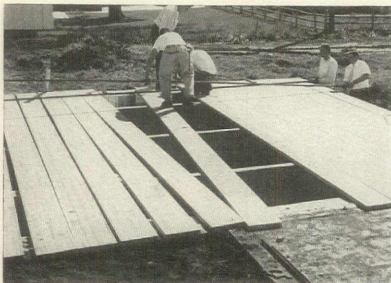
**LAMINATED PLANK FLOORING** serves as structure, rough and finish flooring (Scholz Homes). Planks are 1' wide and 1½" thick, built up from strips of kiln-dried oak. Spiral steel dowels bind the strips. Only 43 planks need be handled in an average 1,000 sq. ft. house. Manufacturer: Edge Grain Timber Products, Inc.
