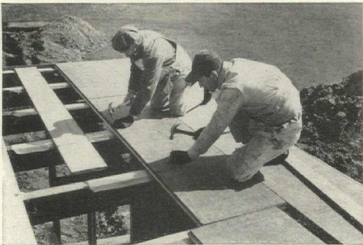
**Big savings in roofing waste** because Temlok Roof Deck with its standard 2' x 8' size can be installed on beams, 24", 32", or 48" on centers. This means less cutting and scrap material—a saving in labor time and material cost for you on each house. Armstrong Temlok Roof Deck cuts cleanly and, as with Temlok Sheathing, there's no dimensional loss.
