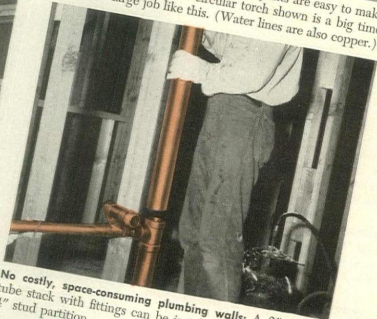
**No costly, space-consuming plumbing walls:** A 3" copper tube stack with fittings can be installed within a standard 4" stud partition.
