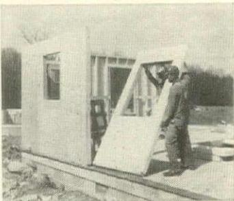
**Closest** to conventional construction is 2x4 panel (Scholz, Lu-Re-Co) which doubles up studs at panel joints. Most panels are shipped with exterior sheathing applied, sometimes with siding materials already on. Tendency now is to ship panels with interior gypsum ready for taping on site, insulation in and provision made for wiring.
