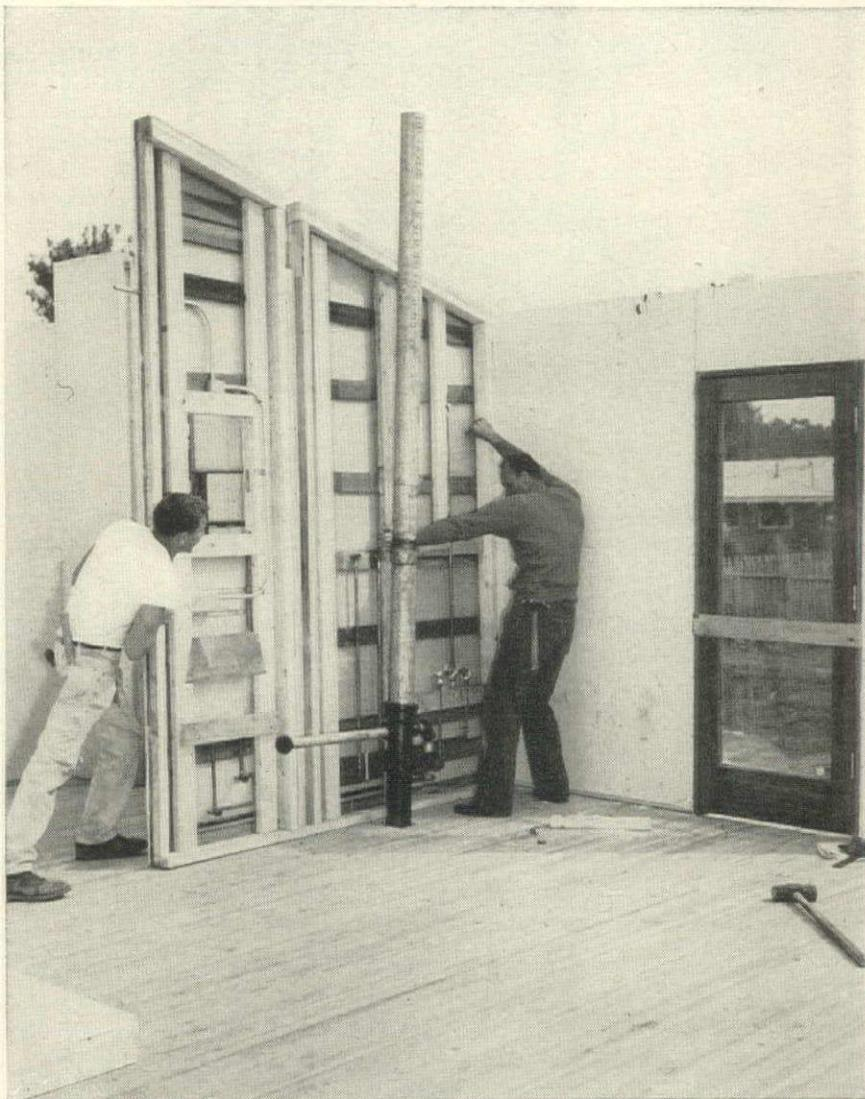
**One 6" plumbing wall** used by Allen Industries contains not only all hot, cold water pipes but also has 4" soil stack. Like most prefabbers, Allen lets his dealers order plumbing at their option. But unlike other prefabbers shown on this page, Allen does not make up his own plumbing package; he orders the assembly (right) from large Indiana plumbing supplier who mass produces similar units for many buyers.
