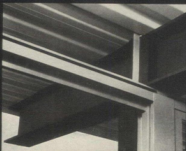
**Steel-framed sliding glass doors** were erected just inside of column line, are thus quite free from structure. Note how welded steel house does away with many flashing problems—a weld being about as tight a joint as you can get. Architect: Raphael Soriano.
