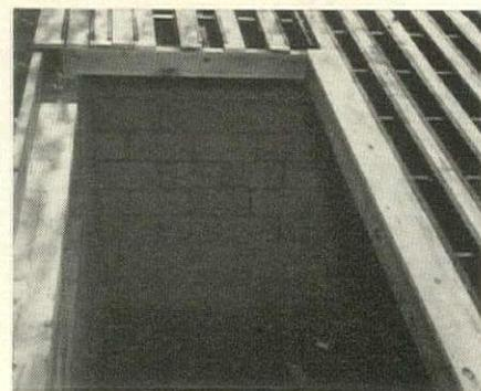
stairwell. Load tests indicate that live load capacities will not make the floor deflect more than the 1/360 of the span recommended for optimum comfort. Joist spans available range from 8' to 16', with 1' increments.
