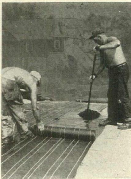
and bond into a solid mass, eliminating one common cause of blistering—felt touching felt. The reinforcing reduces cracking or "alligating" of the actual weatherproofing agent, the bitumen. Because the glass fibers are inorganic, they do not rot or deteriorate.
