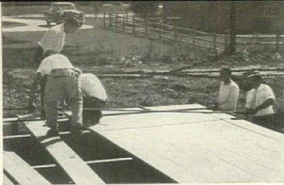
Plank flooring is pulled taut by pipe vises
