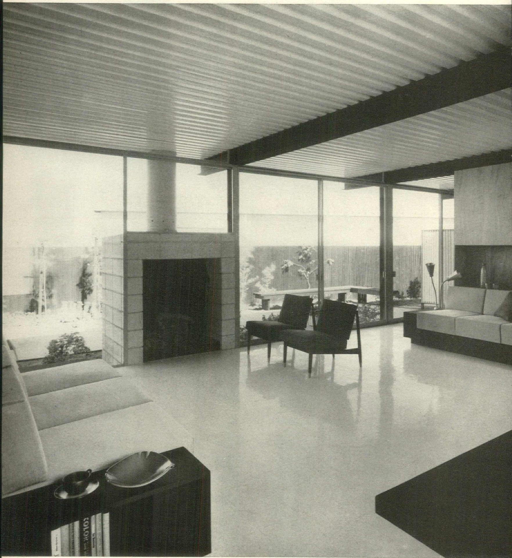
**Wall units** are 8' high, reach up to underside of dropped steel girders. 8" deep space between girders is filled with glass
