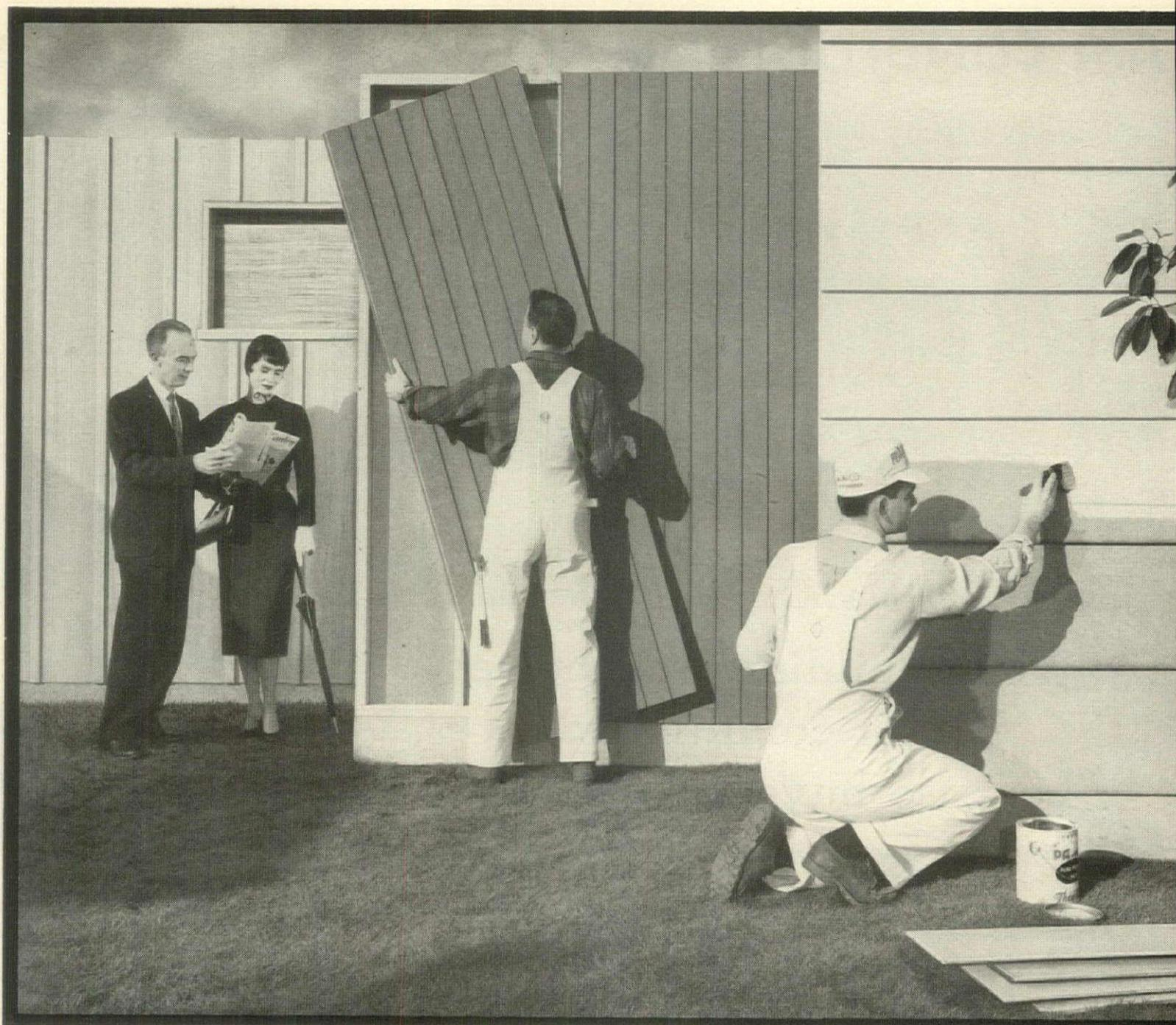
SHOWN ABOVE—(left to right): Rough sawn hemlock board and batten; Tree Life Texture One-Eleven (4" groove spacing); PlyAloy Overlaid Siding.
