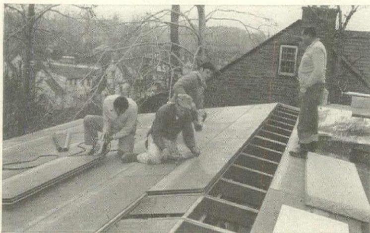
**Labor time is cut 50%** with Temlok Roof Deck. This new building material does the work of several old-style materials. It saves construction time and cost by providing a strong roof deck, complete insulation, excellent vapor barrier, and an attractive finished ceiling—in one material. After your men nail Armstrong Temlok Roof Deck to ceiling beams, only the application of built-up roofing is required to complete the entire roof.
