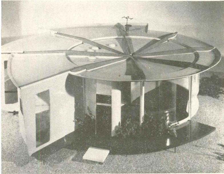
Scale model shows eight pie shapes that make up the basic structure
