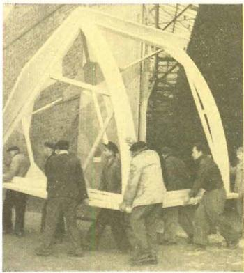
Wooden forms were used to mold the structural plastics skeleton. Here the biggest form is carried into shop.
