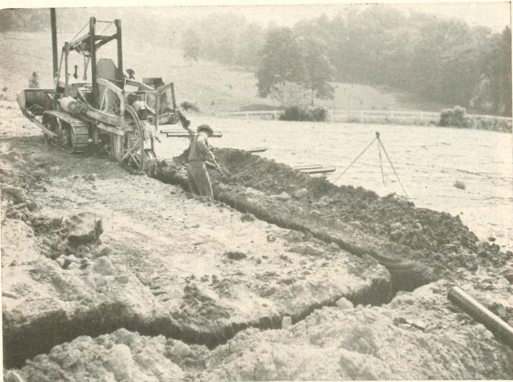
A land-drainage installation of perforated Perma-Line pipe on the J. L. Shannon estate near Detroit. Photo Courtesy Superior Tank Company.
