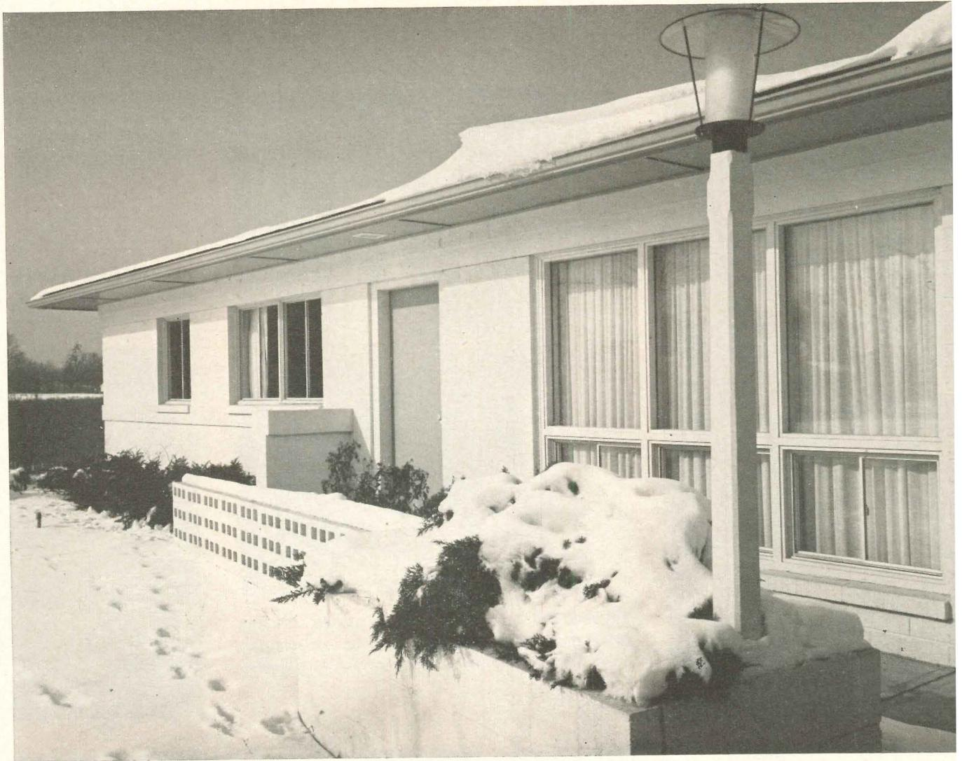
Masonry wall, protecting and outlining entry, is made from standard blocks laid up on their sides to expose cores
