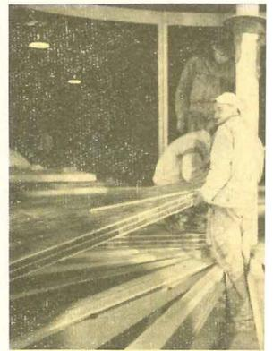
Floor panels fit into pie-shaped skeleton, have honeycomb core with a central layer of insulation.
