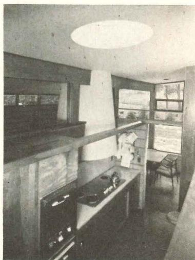
**Central kitchen** controls all areas of the house. Funnel-shaped exhaust stack serves both fan and flue (right).
