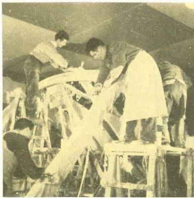
Glass fiber reinforcement strengthens the structural frame. Altogether 13 different plastics were used.
