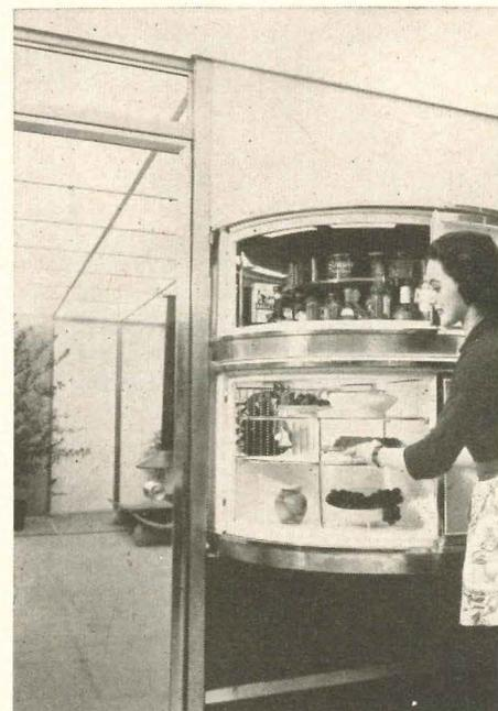
**Refrigerator** rises to waist level, lowers to come counter top extension. Sections rotate loading. Top holds dry foods.
