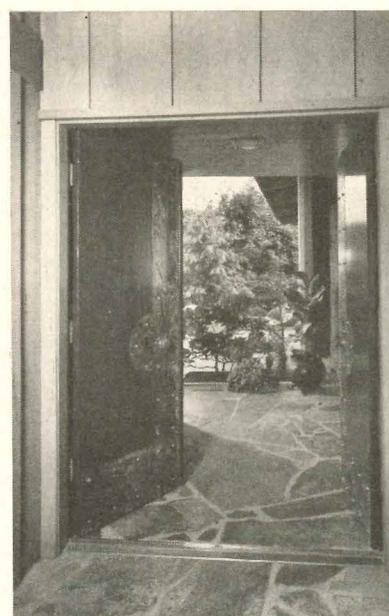
**Elegant front door, lacquered red, has vertegris copper edging made by fast-aging regular plate with acid for an antiqued effect.**
