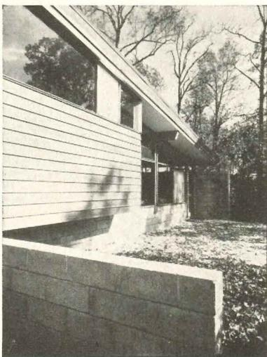
**Shed roof** bridges change in level gracefully, thus unifies the house. Retaining walls simplify grading.
