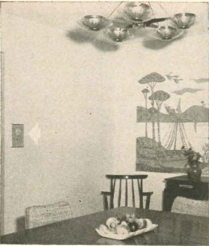
Dimmer switch on dining area lighting fixture works like rheostat, permits wide range of light intensity.
