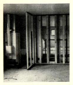
28 Furnace, left, is located near outside wall to save costly runs of fuel and water pipes to center of house. This location reduces height of roof stack and keeps furnace noise away from living-sleeping rooms.
