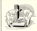
In usual installation, the R⊕M-Hunter Fan (package unit) is placed on attic floor with automatic shutter in hallway ceiling.
