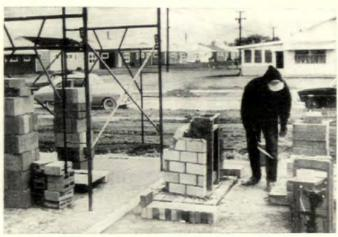
**6** Fireplace jig has sloping back and is marked for spacing and plumb. Jig is pulled out only after the firebrick is laid. Scaffold is used to build chimney before the house is framed in.
