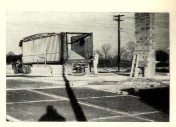
**T** Lumber yard truck is backed against finished slab so panels and trusses can be unloaded quickly on clear, smooth area. Panels are laid flat in the place where they are to be erected.
