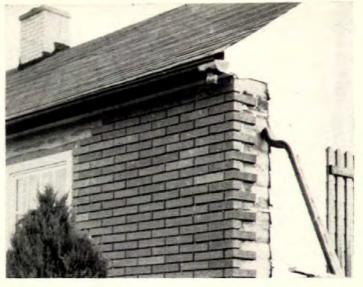
RE-NU-VENEER is a 3/4" thick slab of hard-burned Norman size brick which is attached to exterior or interior walls by placing each unit in a metal clip which is nailed to the existing wall. Brick courses are marked with chalk lines on house walls, and separate Re-
