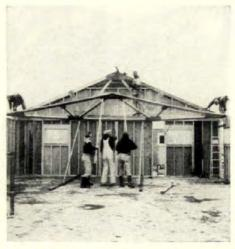
Three men on top put trusses in place as fast as three ground men can tip them up. Two men, on side walls, nail one truss in place every four minutes.
