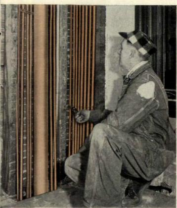
TWO STUD SPACES serve as the chase for the copper tube risers. The large tube is the soil stack; smaller tubes are water supply and heating lines. No space was lost for built-out plumbing walls.
