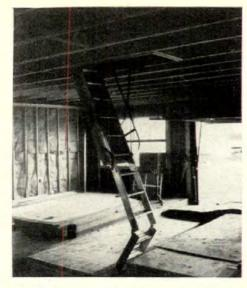
24 Disappearing stairway goes in garage after walls are insulated. Men can then carry ceiling insulation, plywood to attic. House is drywalled as one room.
