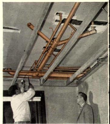
COPPER TUBE made light, fast work of an otherwise tough, slow job of roughing in for two new baths on the second floor. The lightweight assembly is supported by hanger straps fastened to the original floor joists.
