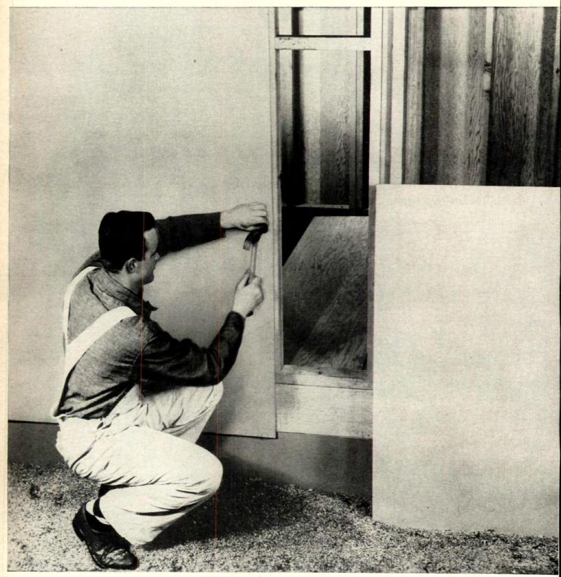
WHAT COULD BE SIMPLER? Duraply can be nailed right to the studs with no sheathing, no building paper. Big size of panels means you can close in a house in a day . . . save extra material and cost of installing them.
