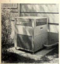
The American-Standard outdoor, air-cooled condensing unit (above) works in conjunction with an evaporator on top of the American-Standard blower-equipped furnace pictured at the right,
