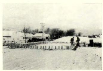
**2** Block is placed on end around the perimeter of the foundation by laborers. This saves mason's time: he lays block, steadily never waits for material or stops to get it himself.
