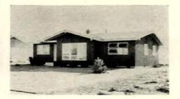
Smallest of three homes has 1,418 sq. ft., no basement, was built of component parts to demonstrate lumber dealers' Lu-Re-Co system.
