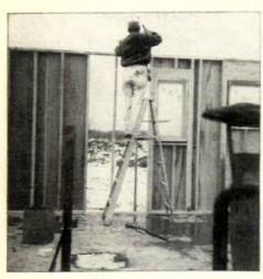
**14** One section of each side is framed conventionally to take up slack in tolerances of foundation and slab. Says Schmitt: "Complete paneling is too inflexible."
