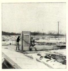
**9** First panel erected includes pre-hung front door and combination storm and screen door. The screen insert for the storm door is stored between the two doors.
