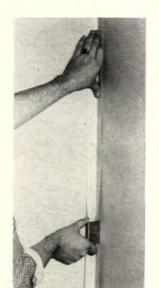
SPECIAL HARBORITE for use as siding, soffits, gable ends, outside storage, interior paneling and partitions is a medium density overlaid plywood. A resin impregnated overlay is permanently fused to a core of "C" grade veneers for resistance to wear, weather
