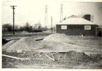
3 Slag for slab bed is dumped in three piles out of the way of heat duct runs which will be laid next. Truck that dumps slag enters the area over a footing purposely left unblocked.
