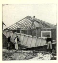
20 Second gable end is put in place. Extra 2x6" on bottom chord becomes nailer board for flooring of 500 sq. ft. unfinished attic under high part of 5:12 roof.
