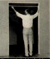
Kenna-pak steel header takes minimum headroom. Eliminates fascia and cutting of doors—standfascia and cutting of doors—stand-ardizes all door opening heights.
