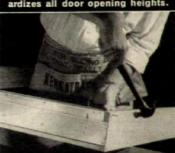
Adjustable Kenna-pak is nailed flush with side jambs.
