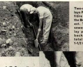
Two-man crew lays Permaline fibre pipe on the Bracy project. They dig sewer trench, lay pipe, and backfill in a total time of 1-1/2 hours.
