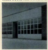
Sliding Doors of aluminum tubes and aluminum sheets roll sideways into compact pockets to allow maximum unrestricted indoor-outdoor space use.
