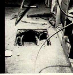
broken (photo) through the thinly cemented top. A workman shatters pipe, removes sand and plasters smooth box-shaped cube to form heat plenum over which floor furnace fits.
