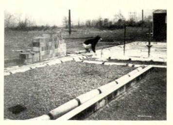
5 Slag is leveled by small bulldozer after heat pipe, plumbing stack are placed. Hand labor completes smoothing. Meanwhile mason finishes laying block, crew lays vapor barrier.
