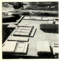
All exterior wall, door and window panels for the house lie on the slab which serves as a roofless assembly plant for Schmitt's four-man panel erecting crew.
