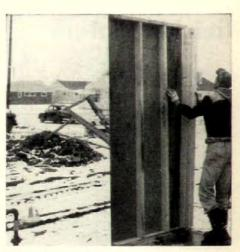
Corner panel, without studs on either side, gets support from preassembled corner post. Same type of panel turns corner, gets support from same post.
