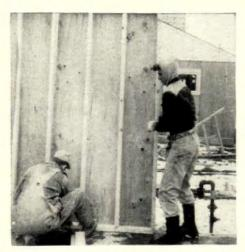
Solid panel is supported by the 2x4" stud on the adjoining panel. Only door and window panels have two end studs preassembled. Studs are 16" o.c.
