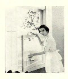
I. MODULAR WOOD WINDOW with double-hung removable sash fits between studs on 48" centers or into Lu-Re-Co panels. Meeting Round Table standards on window sizes (see page 158) the window frame fits a stud opening 46-3%" wide (three stud spaces) with a 40" glass width. Another size fits the 44" Lu-Re-Co panel with a 37-34" glass. Frame has inside trim attached. Carr, Adams & Collier Co., Dubuque, Iowa.
