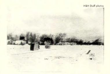
1 Trenches are dug and footings poured for slab on same day. Modular 4" x 8" x 16" block, used in place of forms to retain slab, is stacked at marked position near foundation.
