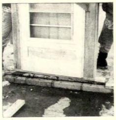
**10** Bottom 2x4" member ties both sides of door panel together, prevents prehung doors from getting out of fit and becomes part of subplate (right of photo).
