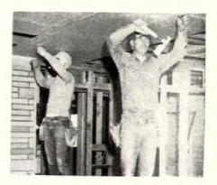
6 Drywall nailers wear helmets to hold wallboard against the ceiling joists while they are nailing it in place. When ceiling has been installed they move to the partitions, which are also covered with wallboard. Hammers used in nailing are rounded on striking face to dimple the board slightly around nail-head.
