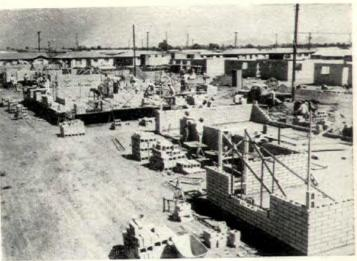
Masons work from conveniently stacked blocks brought to site by unskilled labor using forklifts. The masons lay the 8" x 4" x 16" lightweight blocks fast, as many as 1,000 per day. (They have laid up an entire house in 2 hours, 12 minutes.) Long provides both high and low scaffolding to keep masons from tiring by bending over.
