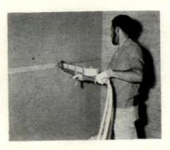
7 Tapers move in with power equipment as the nailing crew leaves. Long is sold on the taping machine, says "one man can do the work of three or four" with it. The machine lays a bed of cement for the joint tape, which feeds from a roll on the cement gun, and then spreads a film of cement over the top of the tape.
