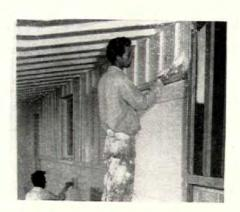
Painters work entirely with brushes. Flat finish paint is used everywhere except in baths and kitchens (and on soffits of flat-top house), which get high gloss enamel. Block walls are painted inside and out except in the kitchen, where the outside walls are furred and lined with hardboard, before being painted.
