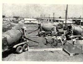
1 Concrete crew places transitmix for slabs and driveways, returns few hours later to finish it. Foundations were poured the day before by the same crew. Concrete crews also pour curbs along streets. (Earlier, Long's excavation crews prepared the site and dug footing trenches with power equipment.) Plant-mixed asphalt road is also laid by Long's own crews.
