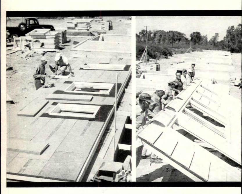
First Step in Dietrich's speedy system is completion of finished shingled sidewall sections lying flat. With strong, rigid Bildrite Sheathing applied to frame, carpenters can safely kneel, walk and work anywhere on surface. Insulite Shingle-Backer and cedar shakes are quickly applied, and wall section is ready to go into place.
