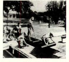
A new shingling method for low pitch roofs can be used either for new houses or for re-roofing with 2/12 to 4/12 roof pitch. Shingles are cemented and nailed over courses of 36" asphalt-saturated felt.
