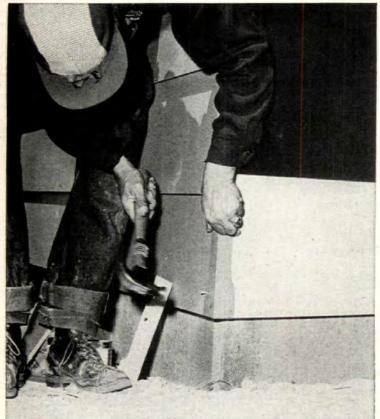
Neat, trouble-free corner construction is easy with Duraply lap siding. Special aluminum corners are a snap to install quickly, correctly . . . cost only pennies extra. Duraply superiority is seen in the number of "repeat" orders builders have made.
