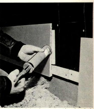
Duraply is caulked at each seam to give a tight weatherproof seal.
