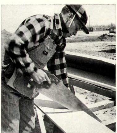
Duraply is easy to work... can be sawed with any hand or power saw used to cut plywood. Special tough overlay holds wood fibers tight—reduces edge-splintering. Ten pieces of Duraply—pre-cut for lap siding—come in each carton (in back of workman)... make stocking easy.
