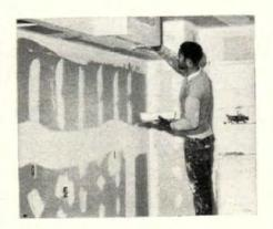
B Joint coaters follow tapers in three hours (time needed for the tape cement to set). Coaters apply broad band of cement to taped joints, smooth it out to a feather edge that completely hides joint in wallboard They also cover nail heads the same way. Coating crew is large enough to provide one man for each room.
