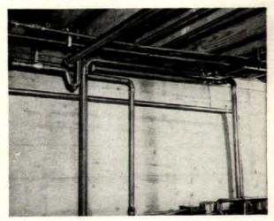
No wrench-room worries here. Easy-to-solder Revere Copper Water Tube can be fitted into the tightest corner. Vertical lines shown come from the water chiller. G&H PLUMBING & HEATING COMPANY, Paducah, was the Contractor who installed the 1,740' of non-rusting Revere Copper Water Tube in sizes from 3/8" to 2". Tube was furnished by the HOE SUPPLY COMPANY, Paducah, Revere Distributor.
