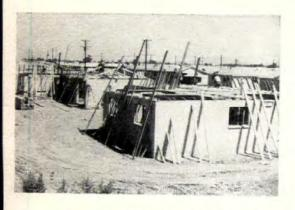
Garpenters install precut partition and roof framing, then the roof sheathing. Lumber is stacked against building within easy reach. Because he uses so many hip roofs, and because his shop-cutting is so efficient, Long feels that rafters are a better bargain in his roof construction than roof trusses would be.
