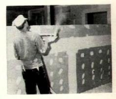
9 Spackle sprayers shoot thin layer of "mud" on wall and ceiling drywall. Unlike most systems, Long's sprayguns have hoses long enough to reach a hydraulic pumping rig outside the house. This lets operator move freely through the house without dragging heavy rig after him. Original pump was developed, built for Long.
