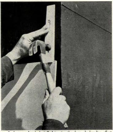
3 Back-up wedge is installed to give the deep, shadow-line effect.
