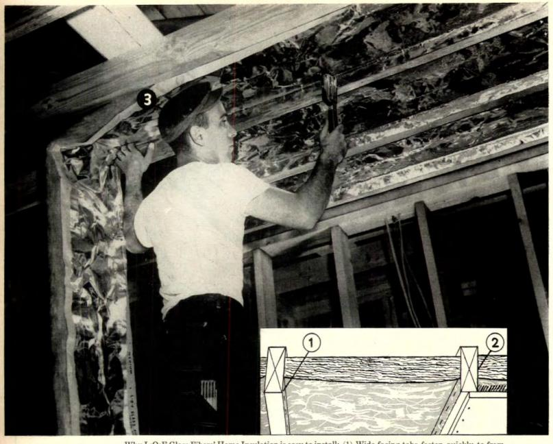
Why L·O·F Glass Fibers' Home Insulation is easy to install: (1) Wide facing tabs fasten quickly to framing, form dead air space; (2) Resilient blanket retains snug fit, prevents heat leakage; (3) Weighs as little as 1 oz. per sq. ft.—is easy and pleasant to handle, stays put for fast, one-man installation.
