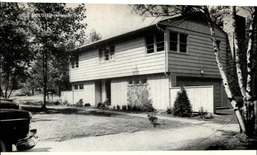
Board-and-batten on front of split-level is actually plywood sheets with batten strips. Big chimney hides middle level at rear.
