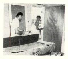
11 & 12 Finish carpenters like the man above follow the texturing crews, hang doors and preassembled cabinets, install trim throughout the house. Note the extensive use of power tools, which are plugged into outlet box on the workbench. (Twelfth step—not shown here—is glazing steel sash, a subcontract.)
