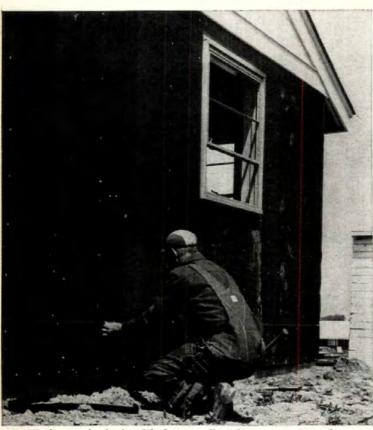
Workman checks level before installing first course. Duraply is exterior grade Weldwood Plywood with a permanent "CreZon" overlay bonded to its surface. "CreZon" (phenolic resins and cellulose fibers) is tough, weatherproof, supersmooth.
