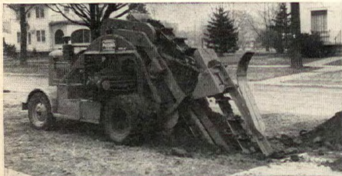
TRENCHING will all be done with this Parsons machine which cuts the 8" trenches at 5 mph and which cost Lively nearly $9,000.
