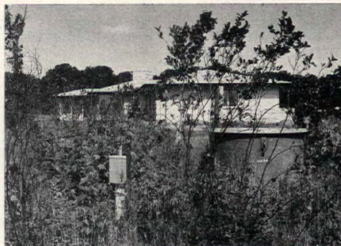
PEDESTAL POST (left) and transformer housing are kept above ground to ease maintenance. They are less conspicuous than pole and wire, can quickly be concealed by plantings./END
