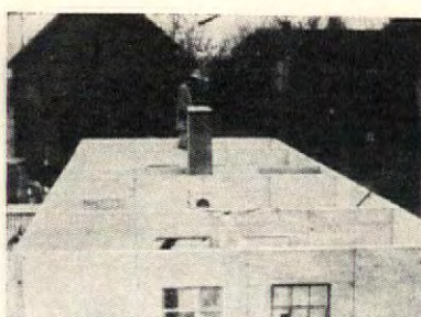
"Stressed covering" panel house was put up in Indianapolis at cost of $1,239 in 1936.
