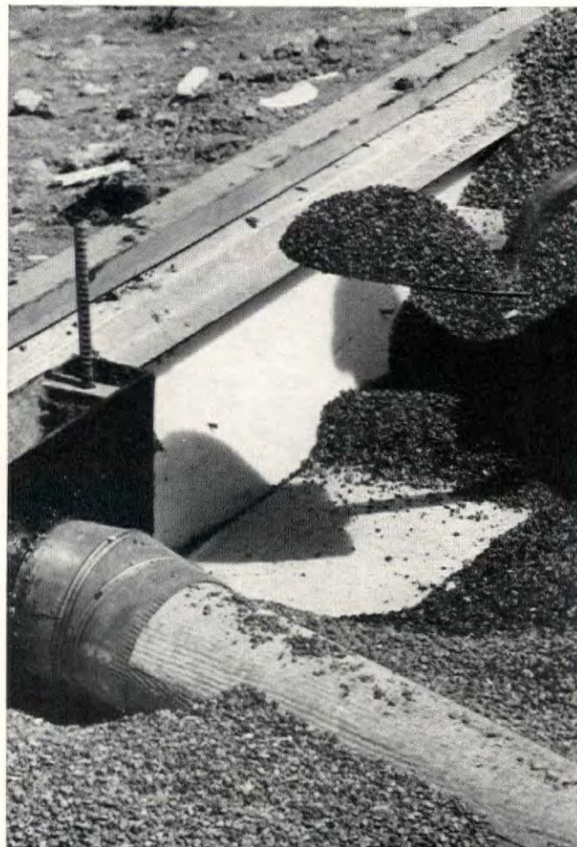
2. Styrofoam insulation 1" thick is then placed at an angle 12" high against the poured foundation wall.
