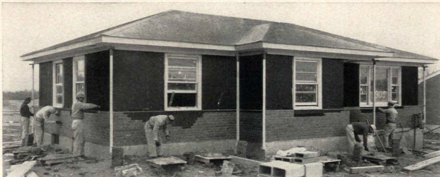
FASTER CREWS can work independently of slower workmen on adjoining walls, as line holders move separately up masonry guides at corners.
