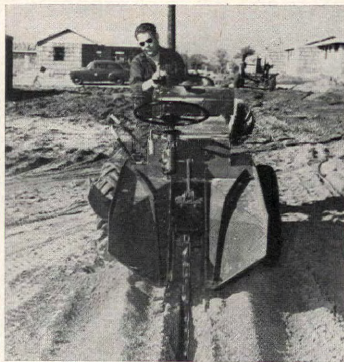
NEW TRENCHING MACHINE , built by Barber Green Co., for use in builder tracts digs a slot 3" wide, 40" deep at a rate of 5' a minute. Small unit does not disturb grade. Cost: $3,200.
