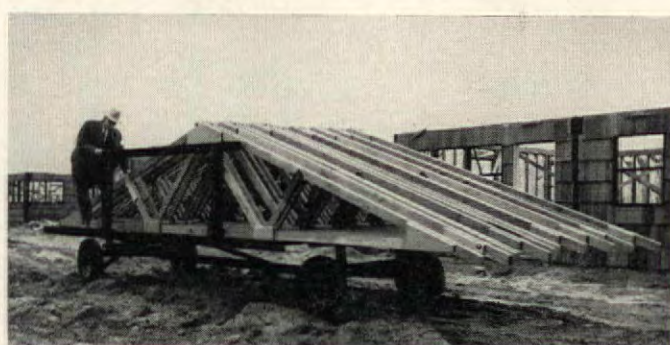
CONVERTED FARM WAGON makes a fine trailer for hauling big, heavy trusses to the site. Boom rig (opposite) hoists them in place.
