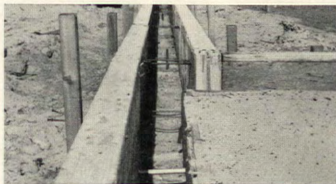
RE-USABLE FORMS for beams help save $130 a house. Labor and materials for block would cost $3.60 a foot; concrete, $2.80.
