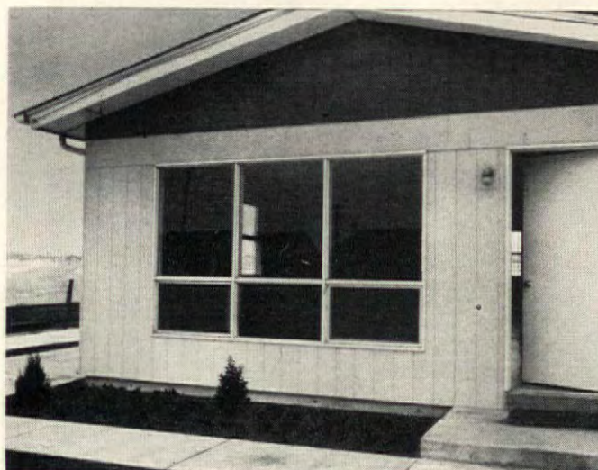
FINISHED PANELS in place have clean uncluttered lines. Gable ends are made in shop in one piece with overhang and soffit.
