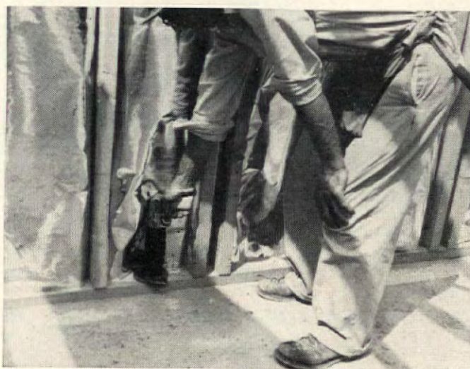
RAMSETTING wall panel plate to grade beam, with a sill sealer between, is a lot faster and easier than setting bolts in beam.
