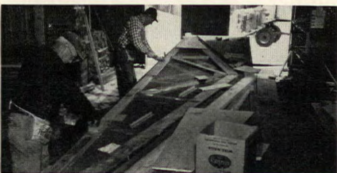
TRUSSES ARE SHOP-MADE with glued and nailed plywood gussets on a simple jig, a bench on which angle irons align truss members.
