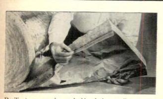
Resilient, compression-packed insulation unrolls to proper thickness. Retains snug fit, minimizes heat losses between framing members and edge of blanket. Reflective facing acts as vapor barrier, turns back radiant heat, extends to form handy fastening tabs.
