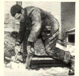
Joints are quickly and easily made by simply tapping together-no cement, no calking.
