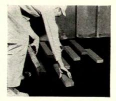
**3** For screeds, use flat, dry 2x4s in random lengths from 18" to 30". Screeds should be preservative treated to prevent rot or termite damage.
