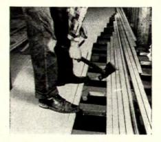
6 Use only tongue-and-groove and end-matched strip oak flooring. Blind nail to each screed. Stagger end joints for strength and appearance.
