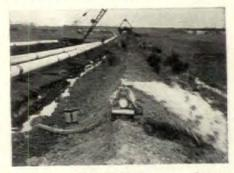
Self-Priming Centrifugal Pumps ... Carry these lightweight, dependable pumps anywhere. Non-clogging design ... 28 foot suction lift ... capacities up to 15,000 g.p.h. ... sizes from 1½" to 3". Diaphragm pump also available.
