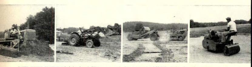
EARTH MOVING EQUIPMENT includes three bulldozers, two pay-loaders, a scraper and \$2,000 unit that digs and seeds lawn at mowing speed.
