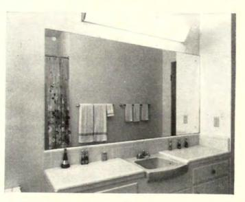
18 "Put some extras in your bath." Holden puts a 7'-long plate glass mirror over the lavatory counters. The lavatory is set in a tile countertop, with drawers and shelves built in below. The lighting fixture over the mirror hides six incandescent bulbs behind its obscure glass. The bath's floor is coved too (see 17). Mirrors and tile counters with built-ins are standard features for all bathrooms in all of Holden's houses.
