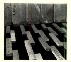
4 Lay screeds flat side down in staggered pattern on 12" centers at right angles to proposed direction of finished floor. Lap joints at least 4".
