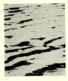
CRACKING occurs with a poorly formulated paint coupled with siding which has moisture in it, or through which moisture can come because of poor wall design.
