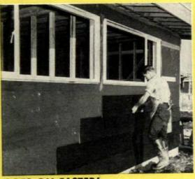
GOES ON FASTER! Costly man-hours saved! One man easily applies lightweight panels. After setting first course, exclusive rabbeted lap provides automatic alignment...eliminates further chalk-lining and measuring.
