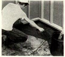
2 With moisture barrier in place, apply mastic to secure screeds over entire slab surface or in "rivers" along lines where screeds will be positioned.
