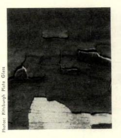
BLISTERING results from moisture, either in the siding or coming through it. The water destroys paint bond and blows up the paint film which flakes off eventually.
