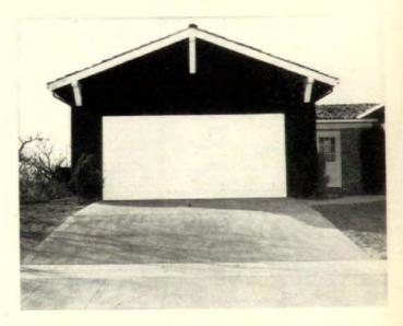
23 "Rough up the surface of sloping driveways." So cars will have better traction in wet, slippery driving weather, the steep part of the concrete drive is given a very rough finish. Most of the driveways in Holden's development have a steep enough rise (though 14% is tops) to make this small point important.
