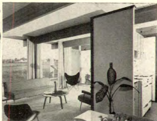
Roof deck also serves as finished ceiling eliminating purlins, joists, bridging, sheathing, lath and plaster.
