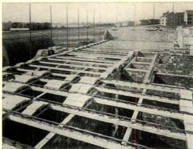
TYPICAL OMNIA PLANK ASSEMBLY
