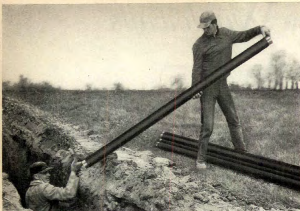
Ten-foot lengths of Permaline Fibre Pipe—pioneered by L-M—are light enough for easy handling. Fewer joints cut handling time, cut costs.
