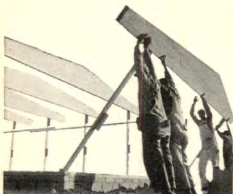
Contractors R. A. Koplow and I. W. Konigsberg erected these twelve Rilco post and beam frames in one hour. Pitched beams spaced 6' o.c. have a clear span of 21' 6" with a 3' 6" overhang.
