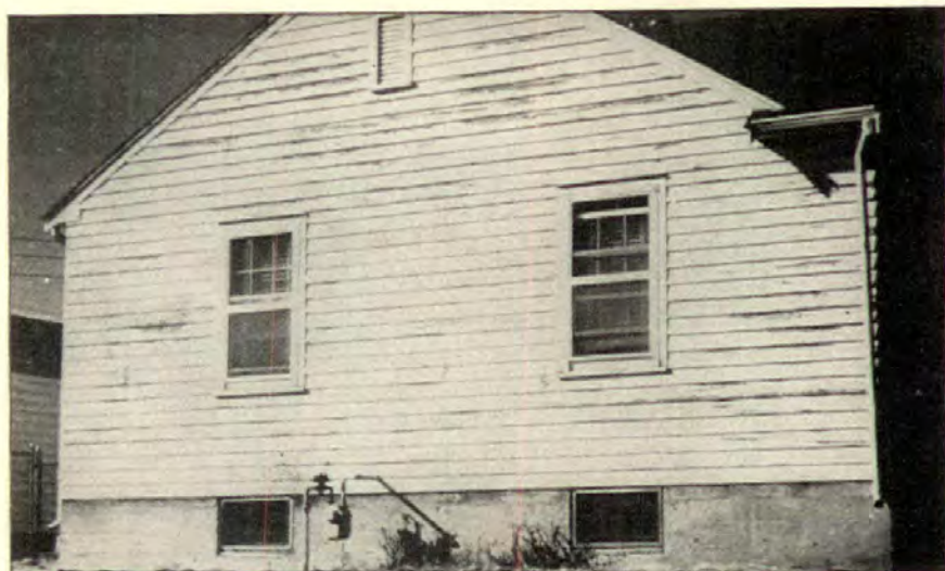
Blistering and peeling paint is one of the most common types of damage caused by the collection of excessive vapor in the side walls.
