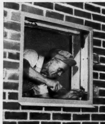
Leave an opening about 27 inches wide, 23 inches high to install General Electric Thinline through wall. Adapter kit makes it easy.
