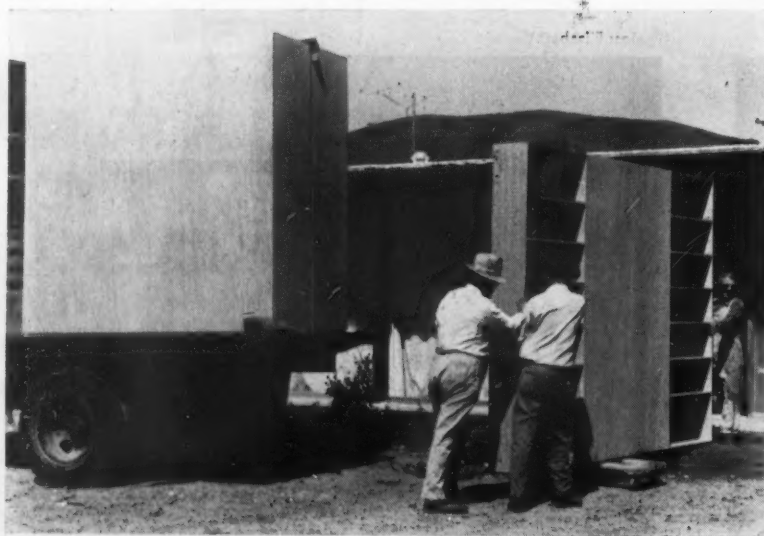
Shopbuilt cabinets were installed after frame, are movable for flexibility.
