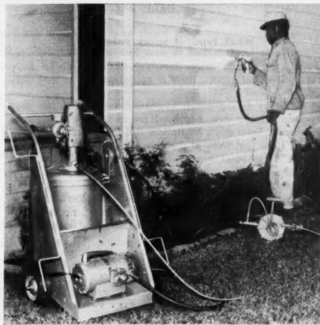
AIRLESS SPRAY EQUIPMENT cuts down the time needed for masking. Because there is no air in the spray, there is no fog or accidental dispersion of the paint to be cleaned up.
