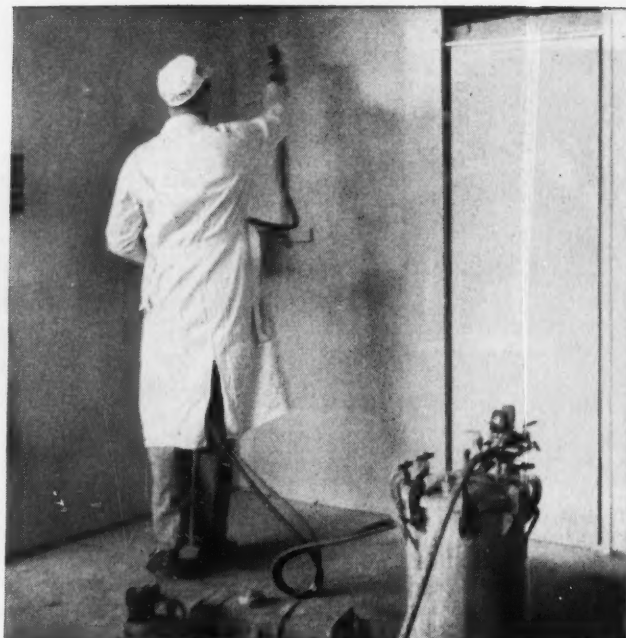
ONE-COAT PAINTS can be applied so fast with industrial cold-spray equipment that a typical room like this Levitt test room can be completely painted in six to seven minutes.
