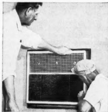
Slide the Thinline in later. Six screws make a strong and weather-tight seal.
