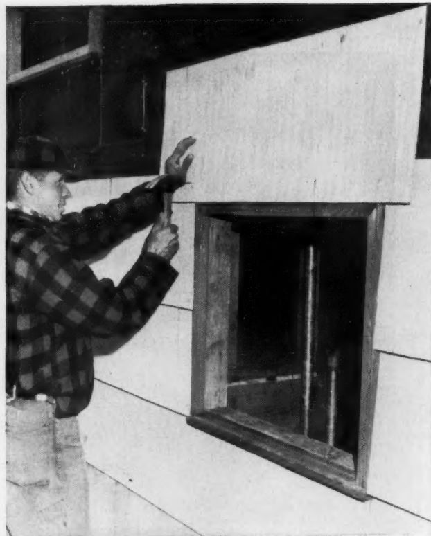
PANEL IS NAILED ON HOUSE by one man. Ready primed shingles eliminate one painting step. Finish paint hides staples and nails.
