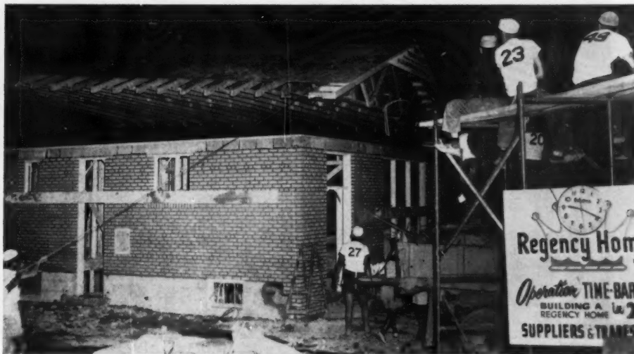
SUN HAD SET BY THE TIME TRUSS ROOF WAS EASED INTO PLACE
