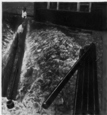
Sewer installation at a project home, by N. J. Rodrigue, Plumbing Contractor, Houma, La. Permaline comes in 5, 8, and 10-foot lengths. Diameters 2, 3, 4, 5, 6, and 8 inches. Full line of fittings, adapters.
