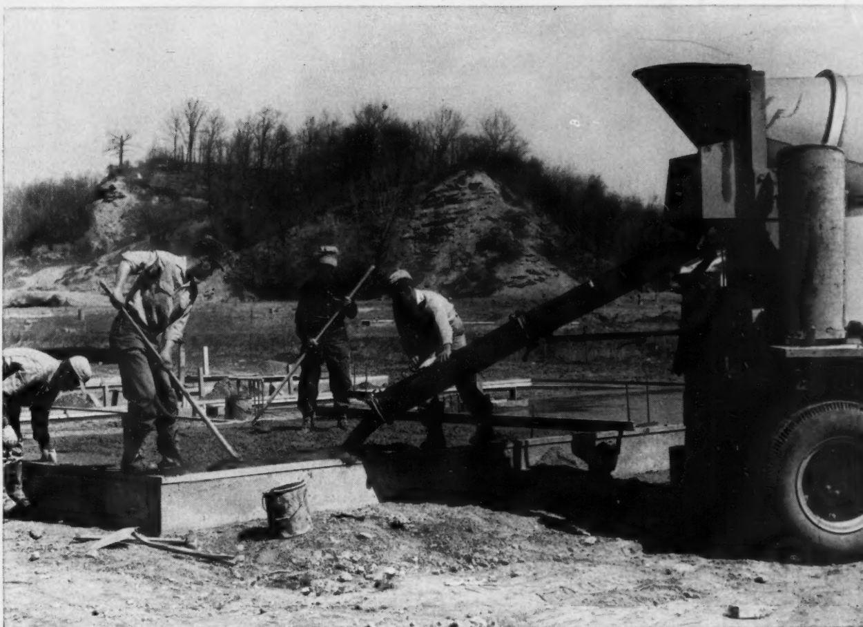
3. Next the slab is poured—and that's it! From experience National Homes finds it has protection from cold and damp for the lifetime of the house.
