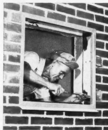
Leave an opening about 27 inches wide, 23 inches high to install General Electric Thinline through wall. Adapter kit makes it easy.
