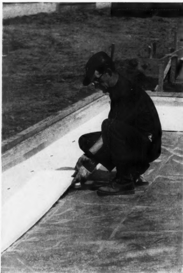
1. National Homes, Lafayette, Indiana, specifies Styrofoam 1" thick placed horizontally around the perimeter 12" from the foundation wall of the house.
