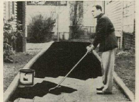
**q. Driveway topping** and sealer combines the resilience of asphalt with the hardness of tar, won't soften in hot weather or crack in cold weather. Use this liquid patch just as it comes from the container. It dries to a hard luster in two to three hours. Product resists gasoline and grease, completely waterproofs and seals driveway at minimum application cost, maker says. One gal. (\$1.75) covers 50 to 60 sq. ft. Sylvania Chemical Co., Cleveland.
