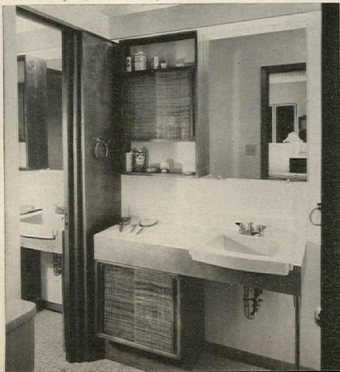
← **SLIDING DOOR**, finished like furniture to match cabinet and vanity, separates full bath (foreground) from lavatory (left). One vent stack, installed in wall between back-to-back toilets, serves both rooms.
