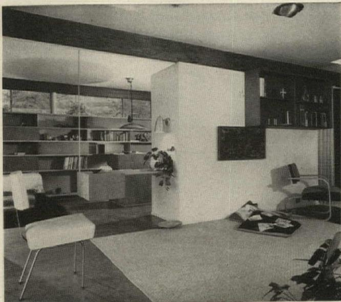
**LIVING-DINING AREA** (b) is separated from studio by storage wall. Continuous lintel (rear) carries roof load, allows room-length window.
