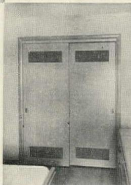
H&K perforated metal grilles in closet doors allow free circulation of air.
