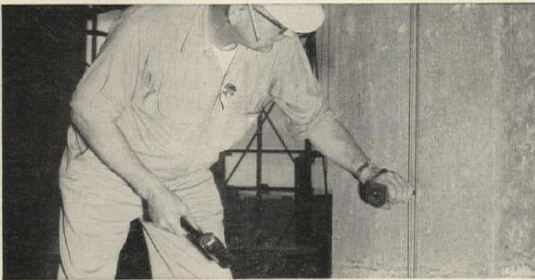
Johnson Service Co., temperature control installers, anchor twin control tubing with SHURE-SET. Drives into hard concrete without a cartridge.
