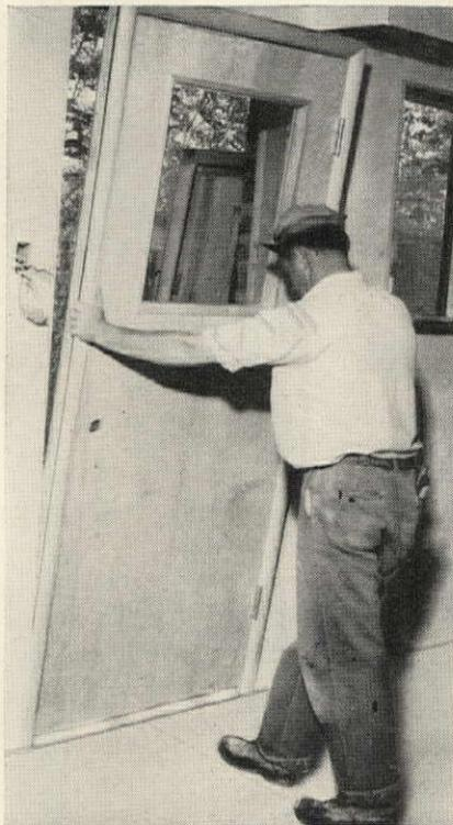
**INTERIOR HALF** is tilted up into opening, dropped into sill notch. Weatherstripped aluminum threshold springs down to grip the finish floor.
