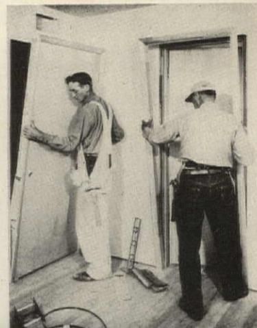
Simply slip the halves together in the opening and nail it in place . . . Takes only a few minutes . . . Assures faster completion and earlier occupancy. Precision assembled to rigid specifications in the factories of the Nation's largest makers of door units, Ready Hung Doors give the entire house that keen look of "expert craftsmanship" that pleases the most discriminating.
