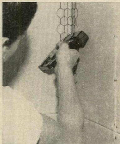
Use either nails or staples with Keycorner. For use over doors or windows, or as strip lath, it can be pressed flat to provide a smooth surface for plastering.
