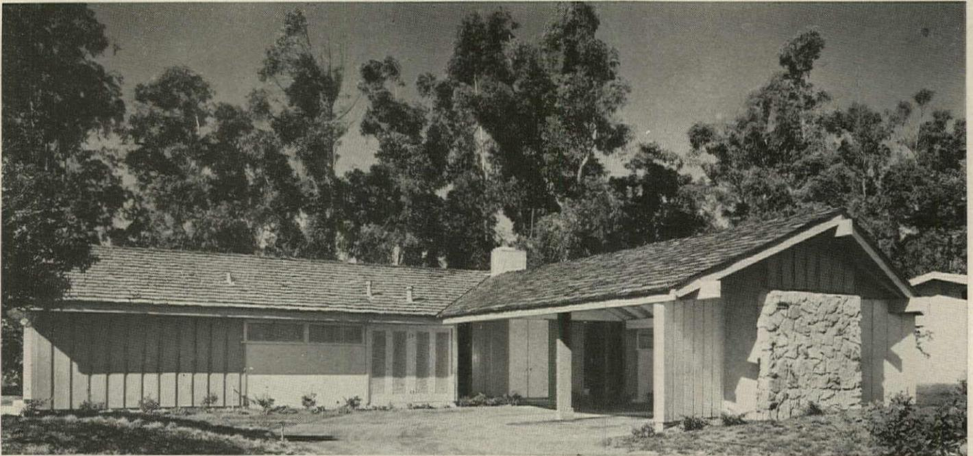
**FRONT VIEW** shows shake roof, reverse board-and-batten siding, stucco under windows, louvered doors to air conditioner, stone at end of carport.
