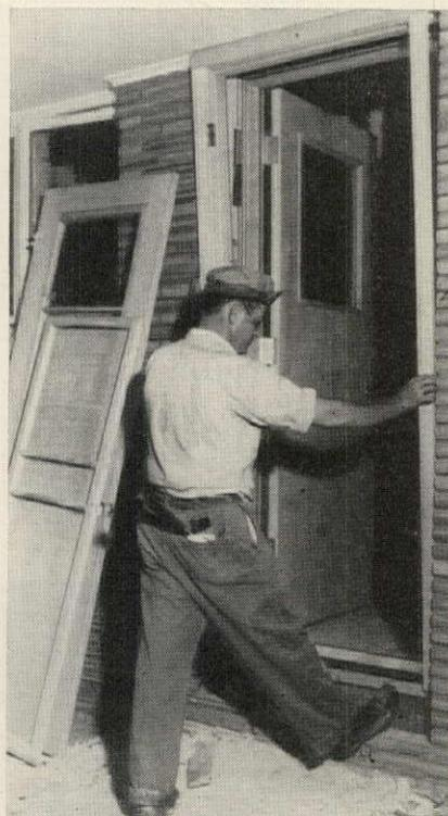
**EXTERIOR HALF** is slipped into groove. Trim laps over butting strips, is nailed flat to it. Frame hides any construction scars on the butting strip.
