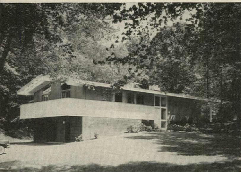
**SPLIT-LEVEL ENTRY**, reached by path from driveway, is between first and second floors, gives equal access to both. From entry, exterior plywood panels with battens extend around house to form balcony wall (left). Other siding is 6" t&g fir. First-floor walls are cement block.
