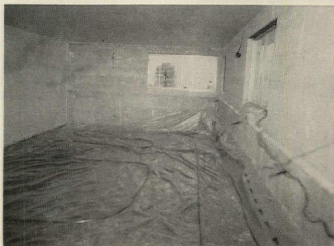
**RADIANT COILS** placed under slab in recreation room carry 205° to 210° return water. Less coil is needed at this high temperature.
