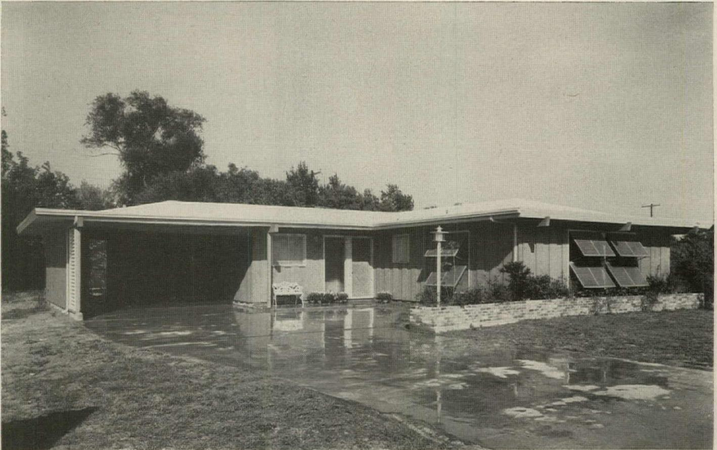
**FRONT VIEW** shows Bermuda flavor. The unusual roof (hips to wall; deep, flat soffit formed by extending ceiling joists) costs no more than most roofs.
