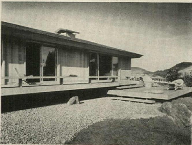
**ON VIEW SIDE**, the wall is mostly sliding glass doors. Upper deck runs the full length of the house; lower deck is outside living room only. Canted fascia makes a thin roof edge (see drawings on pp. 88-9).
