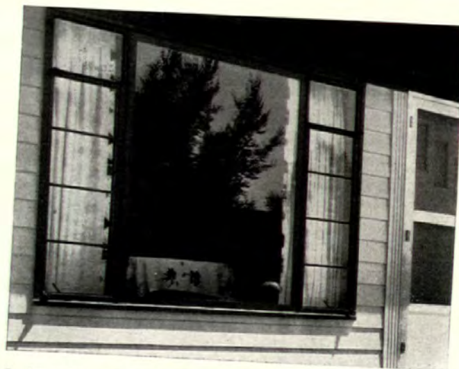
In this cottage, a fixed picture window is flanked by casement-type windows. Thanks to steel's rigidity and its freedom from warping, these casement windows will stay easy to open and close for many years of service. And occasional painting will keep them good-looking for the life of the house.
