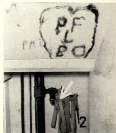
SLASHED FIRE HOSE (arrow) typifies vandalism, as does burned scrawl on walls above. In one 12-floor unit, not a hose worked.
