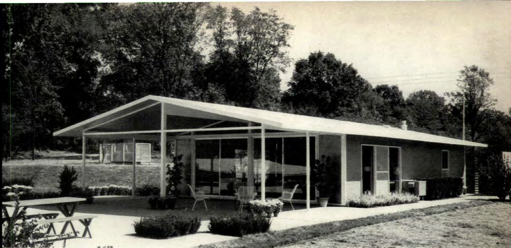
WALLS AND ROOF of this community house in Lafayette, Ind. are "all panel." Ridge beam and porch posts are the only other structure.
