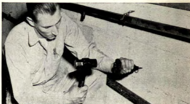
The Feldman Bros. Co., steamfitters, use a chain held by SHURE-SET wire loop fasteners, to support radiators. There's no drilling necessary.
