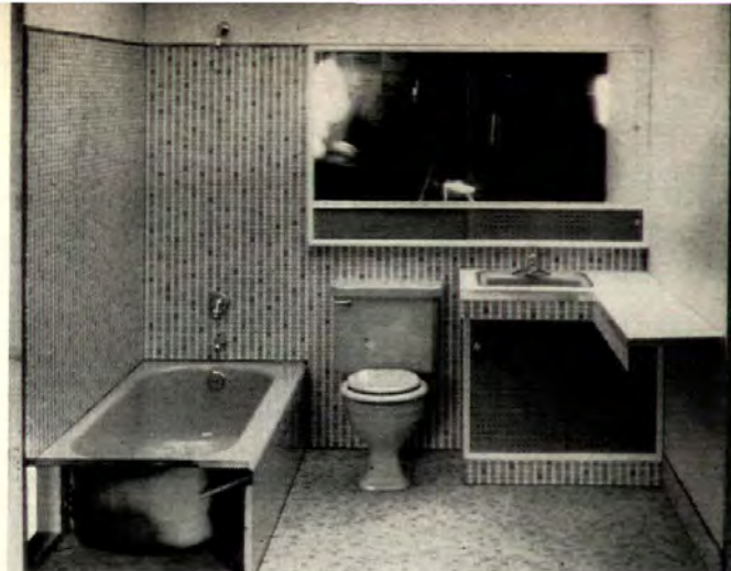
house, luminous ceiling, and prefabricated copper plumbing wall. In the photo left wall panels are removed to show plumbing wall; at the right is a complete unit except for fourth wall (missing in foreground).
