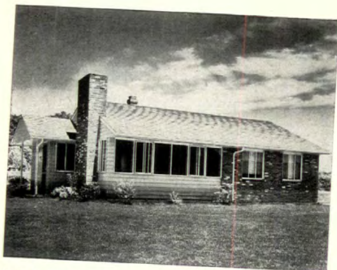
Outstanding feature of this modern home in Washington, D.C. is its window wall—set in frames of steel. Because steel is so strong, it is able to support large areas of glass with slender, inconspicuous frames. Aubinoe, Edwards & Beery, Architects; Aubinoe Construction Co., Builder.
