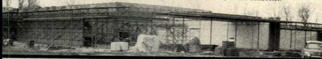
Keywall was used in every course in the Continental Transportation Warehouse. Arnold A. Peterson, architect. Industrial Construction Co., Inc., general contractor.
