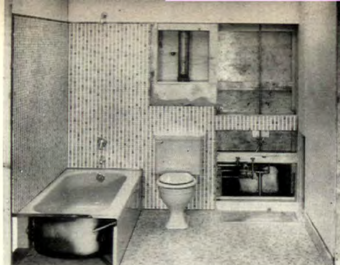
PACKAGED BATH UNIT. available to prefabbers this month, comes with white or colored fixtures (including wall-hung toilet, not shown), ceramic tile wall and floor panels that fasten to the frame of the
