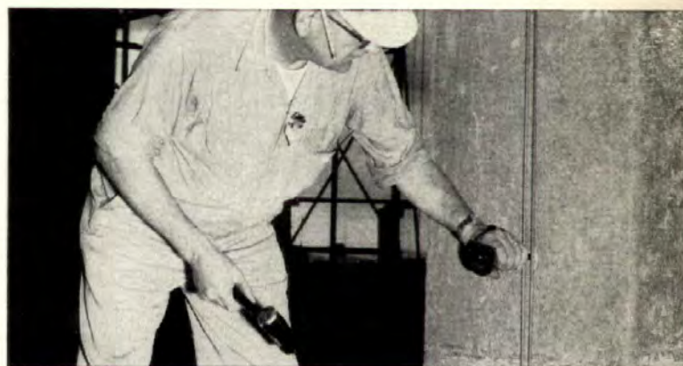
Johnson Service Co., temperature control installers, anchor twin control tubing with SHURE-SET. Drives into hard concrete without a cartridge.
