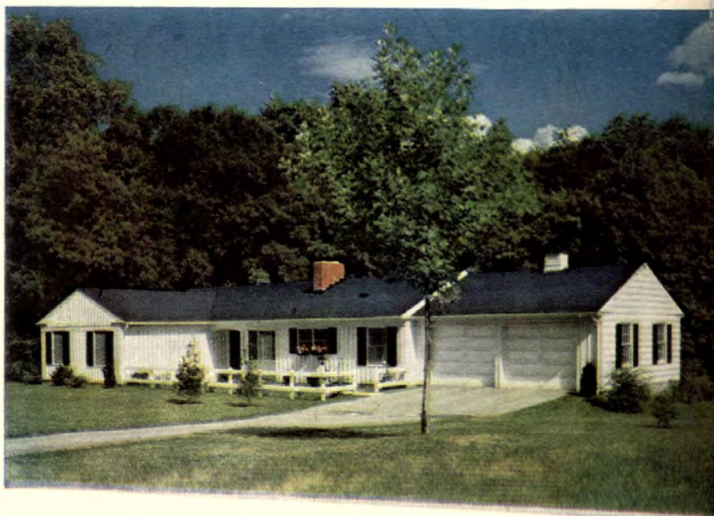
Combination of board-and-batten and bevel siding is one of many exterior-treatment options.
