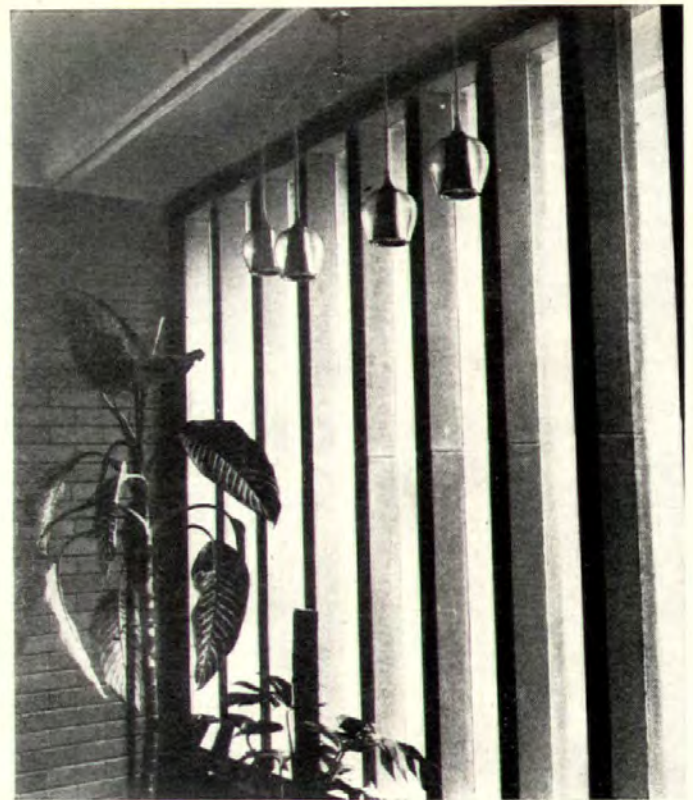
PRE-CAST MULLIONS for front-entrance window trellis are made of the same strong, marble-aggregate-surfaced concrete used for the window frames at left. Windows are glazed with fixed 1/4\"
