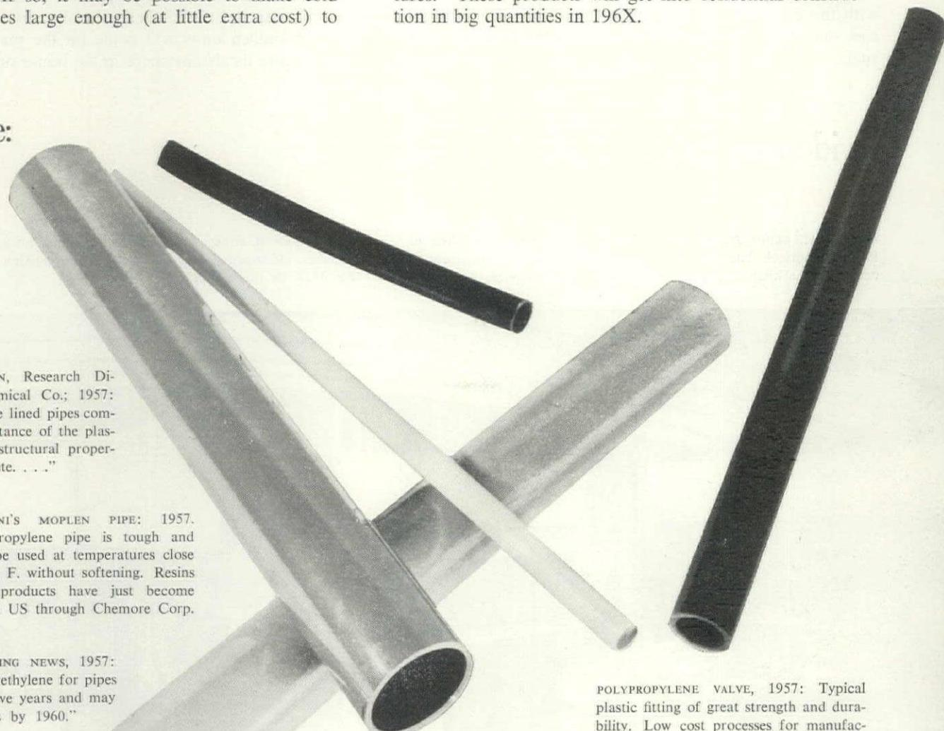
POLYPROPYLENE VALVE, 1957: Typical plastic fitting of great strength and durability. Low cost processes for manufacturing such plastic will shortly put these fittings into residential use.
