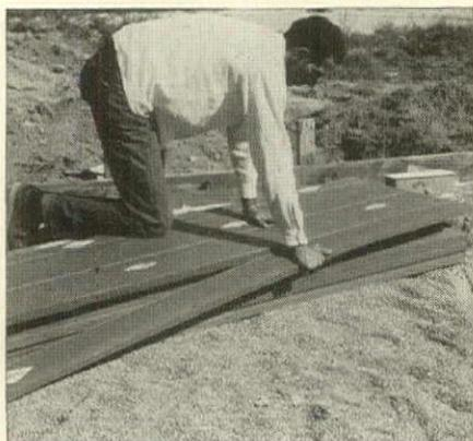
**Black Styrofoam** is now scored so it can be broken to different widths right on the job. Grooves at 3", 12" and 20" marks across the 24" width of each board make on-the-job selection of sizes quick and easy, give a choice of size to fit most foundation and cavity walls. Called Scorboard, boards are 1" thick, 8' long.
