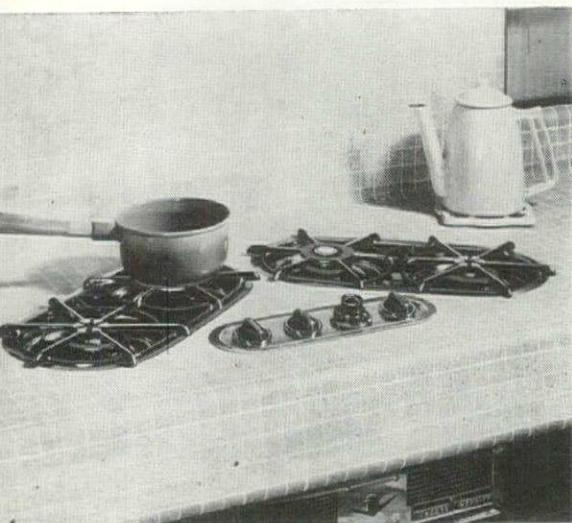
**Built-in cooking top** is designed for installation with ceramic tile. Burner pans fit level with counter top and small lip on pan allows a tile setter normal leeway in fitting tiles around pan area. No cut-out in the cabinet front is needed since controls are included on the cooking panel.
