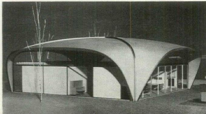
**FOLDED ROOF, Atlanta, Ga. 1957:** Circular patio in center of this house is covered by stressed skin, wooden folded roof. Steel compression ring in center contains skylight. Tension cable around periphery keeps roof from flattening out. Architects: Alexander & Rothschild.
