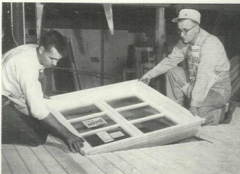
**6** Window installation is easy (calls for no wedging) because opening has been framed and trimmed accurately. Casement and double-hung units are already glazed, hung and prime-coated when Auburn buys them, get final paint coat at site.
