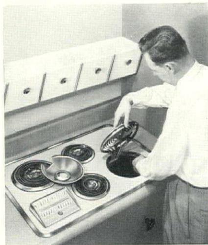
Tighten six thumb screws . . . connect one conduit . . . the job is done in minutes! Built-in oven and drop-in cooktop have been completely installed in as little as 36 minutes from cartons to finished job.
