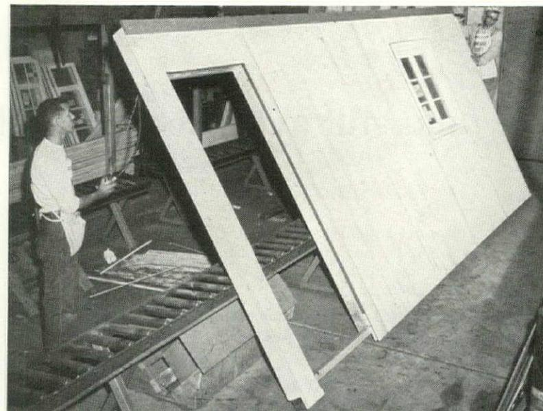
**7** Finished panel is lifted off assembly conveyor and set on dolly (photo 8) by two electric hoists. Smart idea: to keep door frames from buckling, bottom plate has been extended under opening—will become stool when panel is erected.
