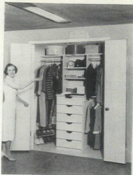
**Bi-Fold door unit** operates without guides, tracks or pivots. Doors are hung on regular full-mortise hinges and a spring in mortise at top of door passes over hinge pin to give automatic folding and unfolding operation. Spring holds doors straight when closed, keeps them folded when open. Two-door unit for openings up to 3'; four-door units for openings from 3'-6'. With split jamb, installation takes about 20 minutes. Ready Hung Door, Fort Worth.
