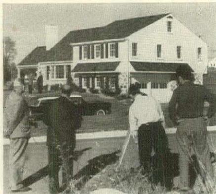
borough, and Max Fink show how they each have used the "new look" in asbestos-cement siding, and why. They detail how—with a full undercoursing of fibreboard to "kickout" the shingle and reinforce it—the flat look that used to be asbestos' giveaway has been eliminated. They point out the savings they have enjoyed in using asbestos shingles, the simple installation, the wide variety of colors and easy maintenance they can offer their buyers.
