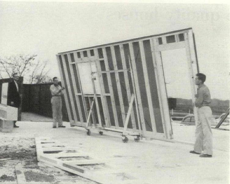
**8** Shop-made dolly is used to tote panel into trailer, which carries all components for one house. Two chunks of scrap lumber, nailed to bottom plate, serve as bumpers to protect panels. They will be knocked off before panel is erected.
