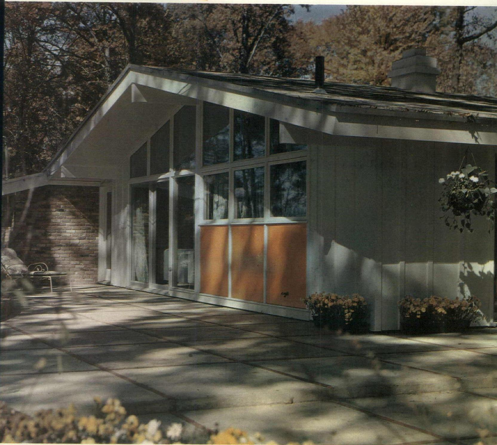
The exterior finish walls are built with pre-primed Johns-Manville Asbestos Flex-board which lends itself beautifully to the authentic board and batten styling of the true California ranch style architecture of the Mark 58. This siding material is rotproof, fireproof and weatherproof. In addition it provides an excellent paint base, not subject to the wide variation in paint holding characteristics of other siding materials.
