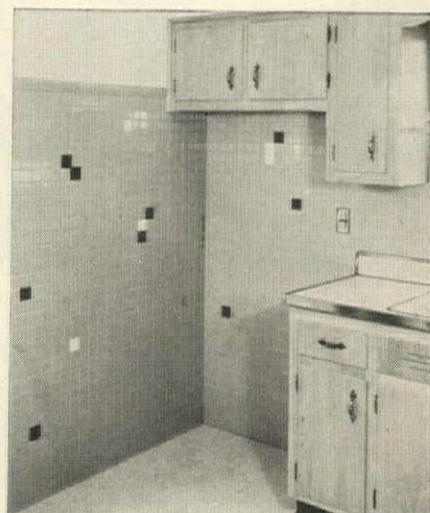
**Plastic wall tiles** in 4 1/2" squares are now molded to give appearance of four small squares. But it has 50% more water seal contact with the wall, goes up faster than small tiles. Costs and application methods are the same as regular 4 1/2" tile. Known as Modern Mosaic, the new tile is available in 15 colors, may be combined with individual quarter tiles as shown above.
