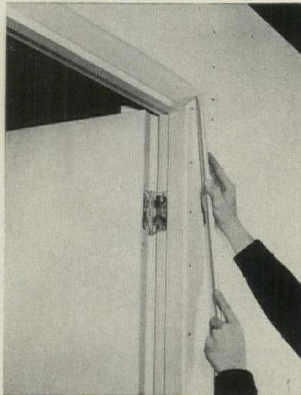
**SPLIT-JAMB DOOR** slips into opening . . . . . Stop and trim complete the job.
