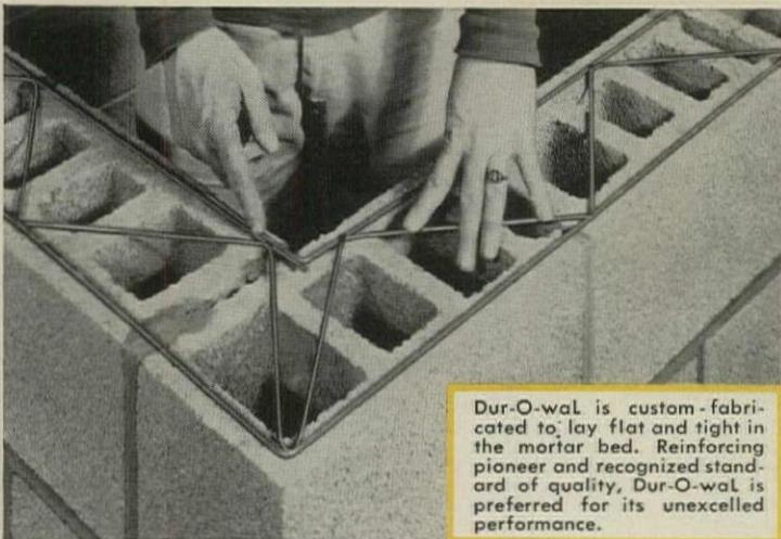
Dur-O-wal is custom-fabricated to lay flat and tight in the mortar bed. Reinforcing pioneer and recognized standard of quality, Dur-O-wal is preferred for its unexcelled performance.
