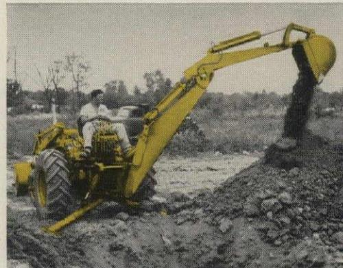
Ruggedly-built Case "320" backhoe, with exclusive hydraulic foot-controlled swing, digs hard clay with ease. Comfortable back-rest seat reverses for operating loader.
