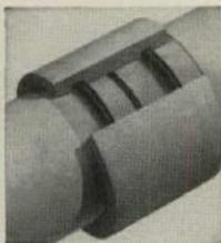
The familiar Ring-Tite® Coupling speeds and simplifies assembly of Transite Sewer Pipe.
