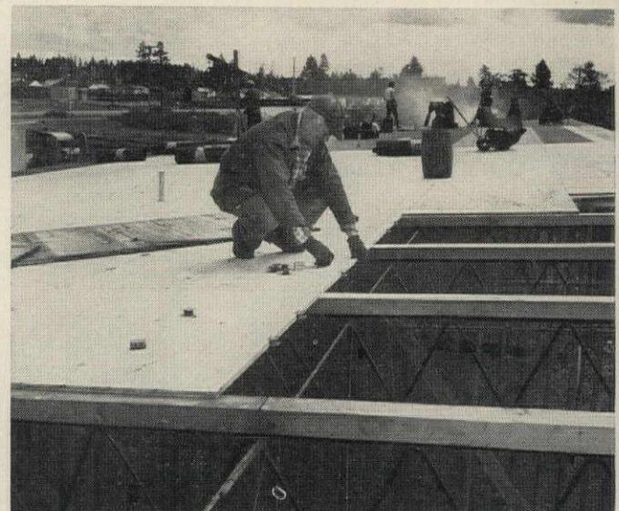
**HOW YOU USE PLYCLIPS** is shown in this installation of a plywood roof deck on beams 4' o.c. on a new supermarket, a DFPA's test job.
