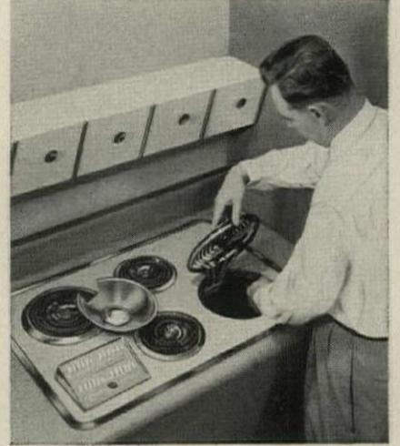
Tighten six thumb screws . . . connect one conduit . . . the job is done in minutes! Built-in oven and drop-in cooktop have been completely installed in as little as 32 minutes from cartons to finished job.
