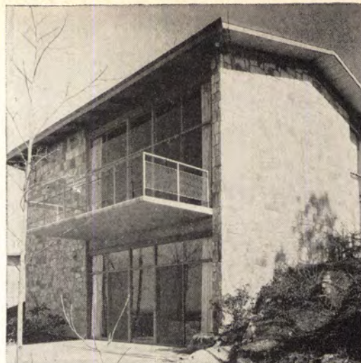
Only steel frames had the combination of strong yet thin sections which made this design possible.
