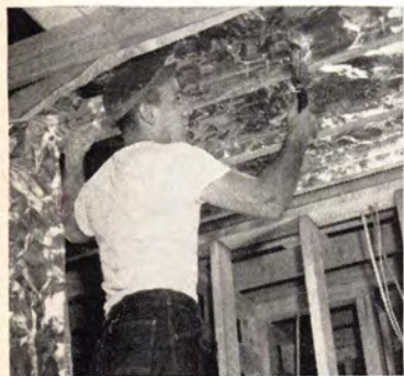
1. One man installation. Light weight blanket is self-supporting while handy tabs are stapled.
