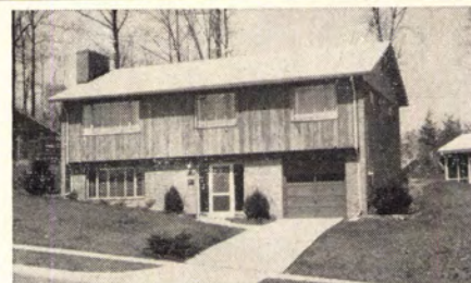
GARAGE under house costs about $1,200 less than if built alongside, allows 14% drive. Bldr: Northwood Pk Devel Co, Arch: Jack Cohen; Silver Spings, Md.
