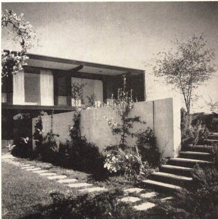
RETAINING WALL of reinforced concrete is dramatic part of house, also shelters terrace on upper ground level, provides surface for vines. Architect: Roy Binkley; Builder: W. J. Schuchardt; Prairie View, Ill.
