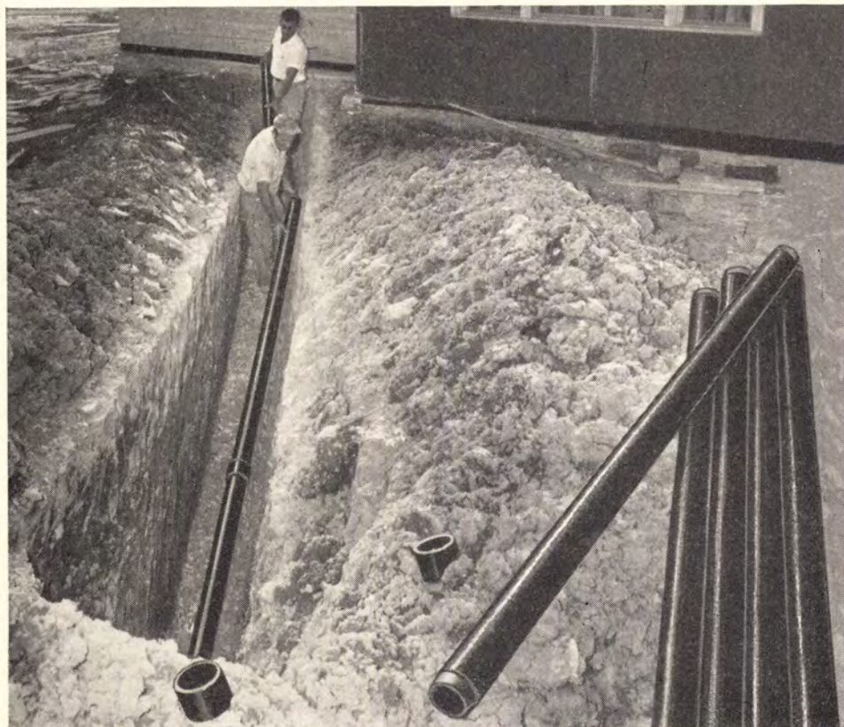
A Permaline fibre pipe house-to-street sewer installation by N. J. Rodrigue, in a home project at Houma, Louisiana. Builders all over the country have found Permaline economical, profitable to install.
