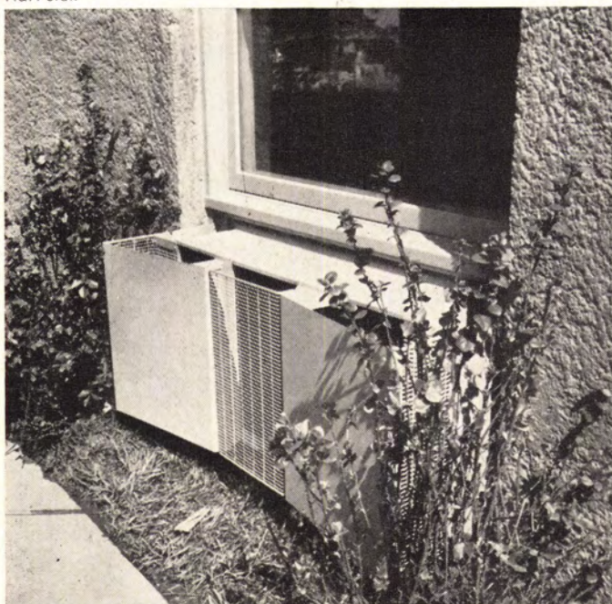
OUTSIDE GRILL fits over outer face of heat pump, provides plenty of space for air flow. Grill was designed by George Nelson.
