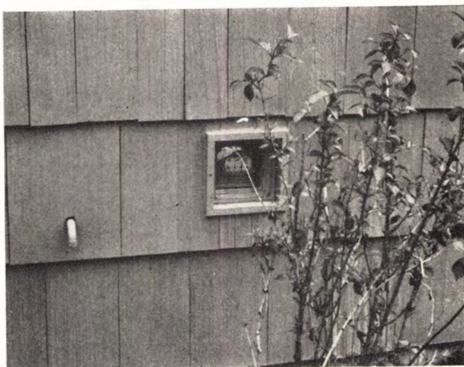
SMALL WINDOW in outer wall permits reading of interior gas meter from outside. Exterior meters cost more, are also unsightly.
