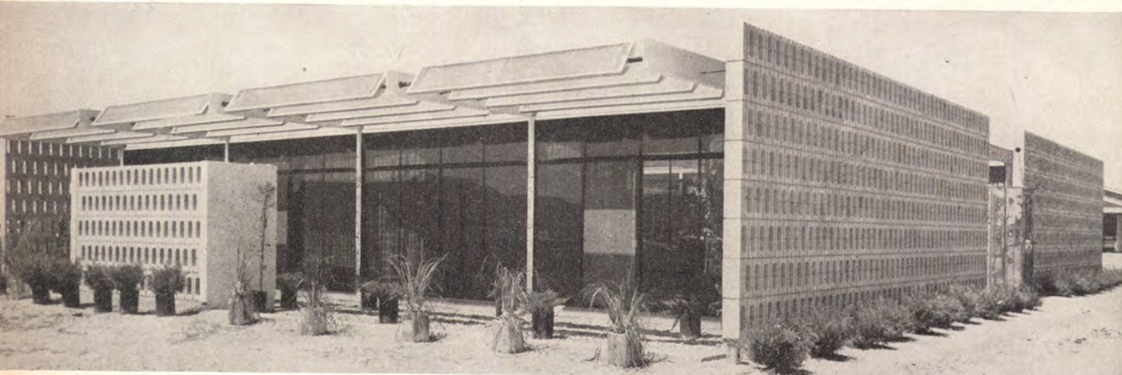
FOR SUNSCREENS in solar heated house in Phoenix (H&H, Jan 1958), specially sized blocks make a wall pierced by cell openings. The block
