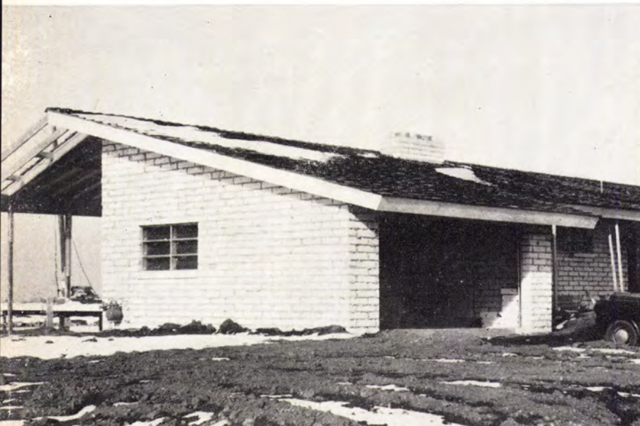
EXTERIOR WALLS of this Denver house are made of Durox block—a foamed concrete. A wall like this has a U factor of .11, works well in the north. Exterior gets silicone treatment.
