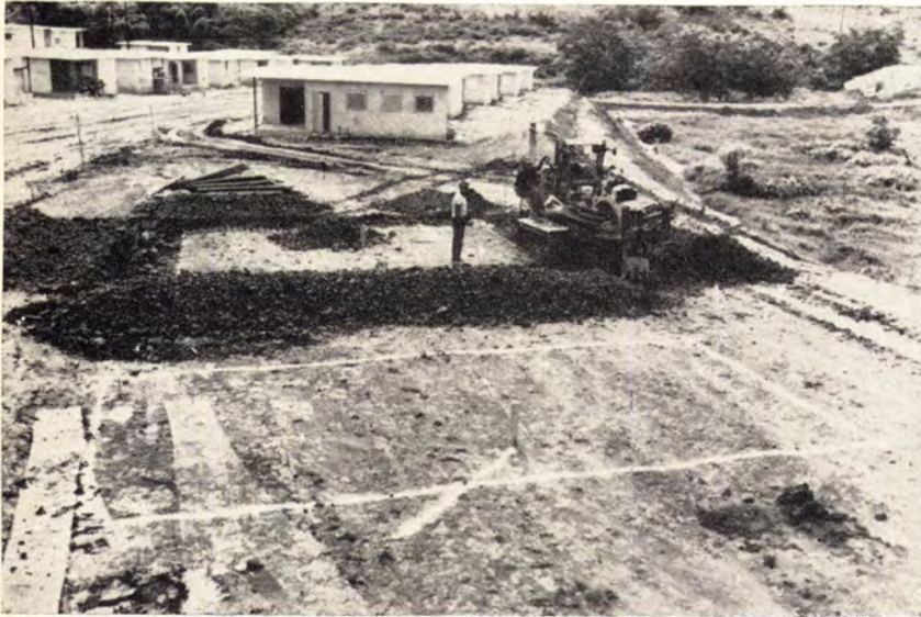
TRENCHER digs 2½' deep footing trench for foundation. Back-hoes are also used for this job. Subgrade under house is pneumatically compacted to 95% density.
