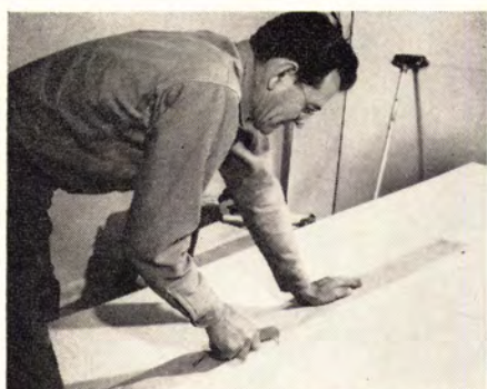
You can cut Clad-Rex with linoleum knife ...
