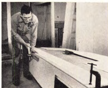
and bend over table edge at score mark.
