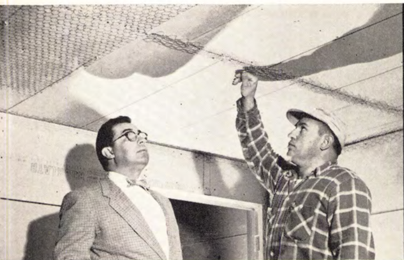
Eby (left) inspects application of Keycorner, used to reinforce joints. Keycorner is also used at all wall and corner junctures.
