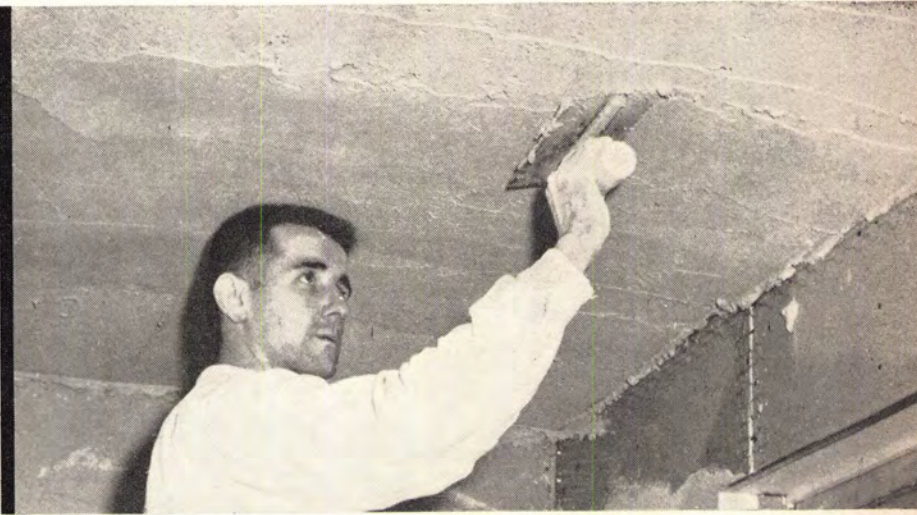
Plaster is applied over reinforced ceiling. The open mesh of both Keymesh and Keycorner assures imbedment in plaster. The open mesh also insures full bond of plaster with gypsum lath.
