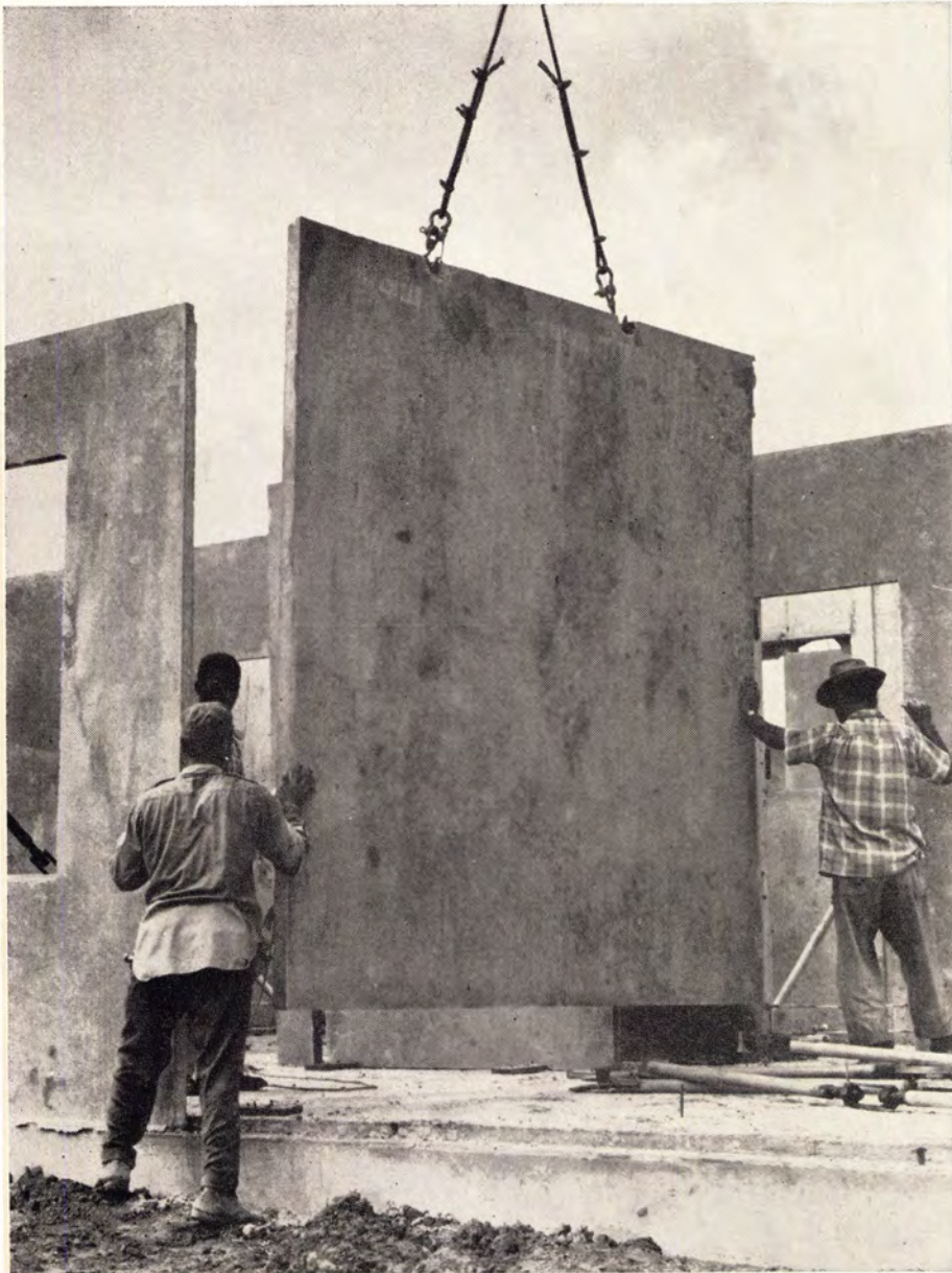
PRECAST PANELS are moved into place on slab by crane. Finished two bedroom houses will sell for $6,500, three bedroom houses for $7,750. Even flower boxes and porch walls are precast.
