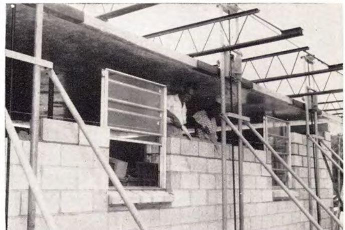
FOURTH STEP. Block walls are built with windows in place. Roof slab is lowered on.
