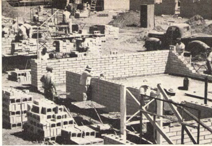
Concrete block walls of John Long houses going up in Phoenix.
