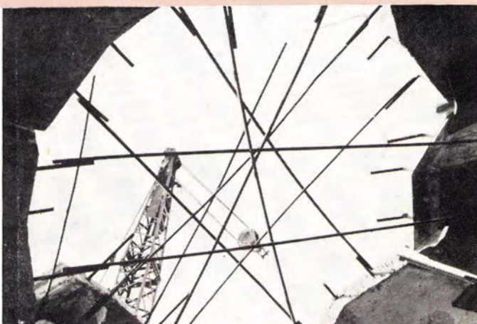
VIEW from middle of house shows opening which will have concrete framed skylight.
