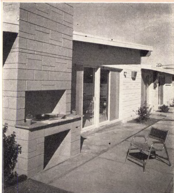
FOR A BARBECUE , only two sizes of block are needed for patterned face in this Tucson house by Bob Lusk.
