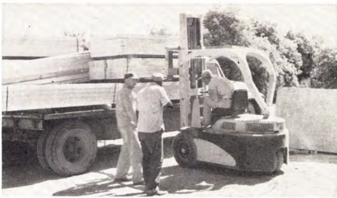
FOAMED CONCRETE SLABS called Siporex come strapped on pallet. Fork lift is used for rapid unloading. Slabs are 8' long, 3 and 4" thick.
