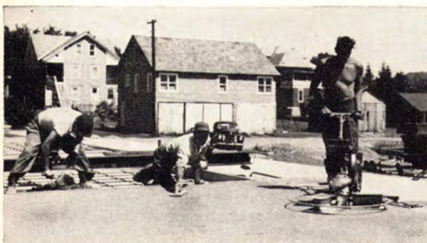
FINISH FOR WALL PANELS is very smooth to take paint inside and out. They are first wood floated and then steel troweled with the power float at right.
