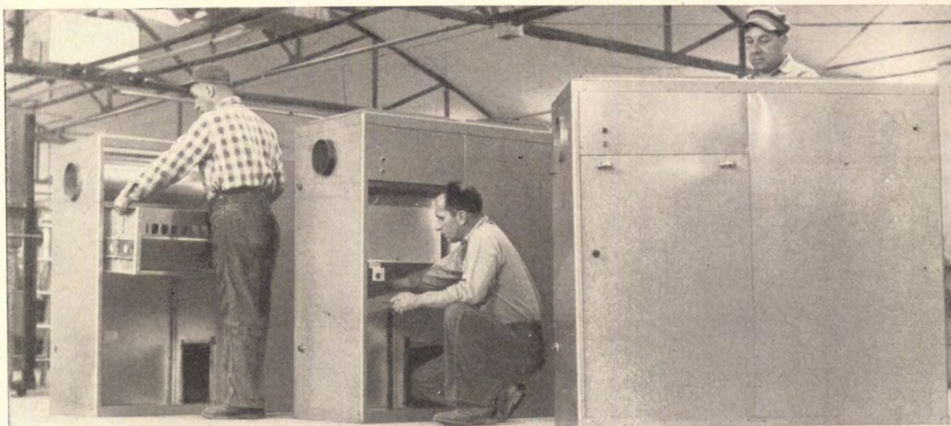
FIRST PRECIPITRONS are installed in Steel City furnaces.
