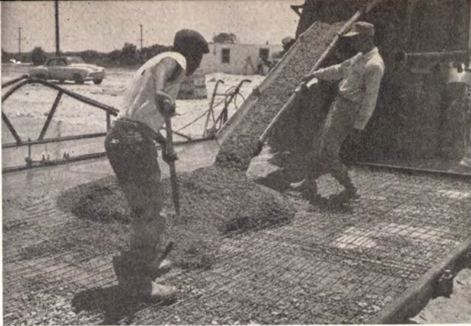
Floor slabs being poured at Isle of Pines project.
