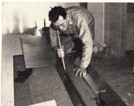
To bend it, score metal with glass cutter ...
