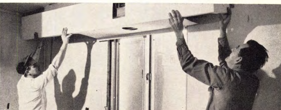
position form on adhesive-coated wall, roll in place to get sure contact.
