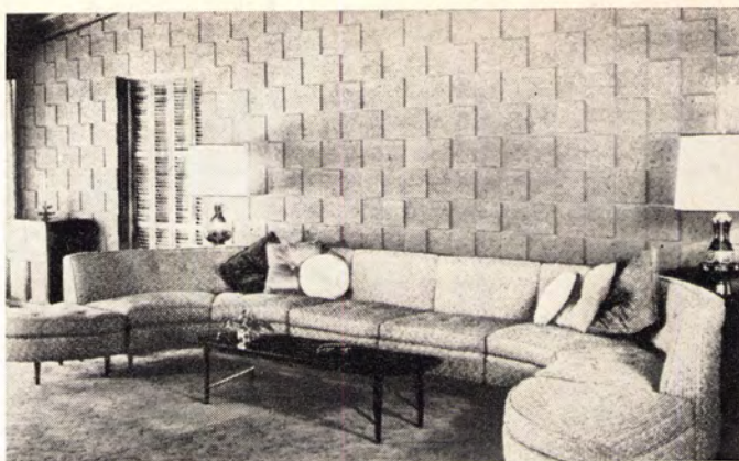
FOR LIVING ROOM WALL , square concrete block units are set in an alternating offset pattern. Mortar joints are tooled flush with face.
