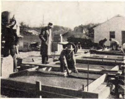
CONCRETE SANDWICH panel is cast on slab of house for small volume operation. Foamed glass insulation is placed in core, then top concrete finishes sandwich.
