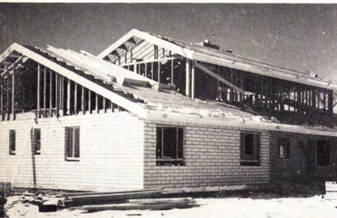
BLOCK WALLS of Durox for first floor of this Colorado house are combined with stud walls on upper half story. Sole plate for gable end is nailed right into block wall.
