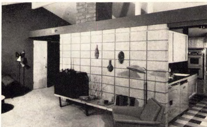
FOR ROOM DIVIDER in house by Palmer & Krisel solid concrete block units are laid up in stack bond with a deeply tooled joint.
