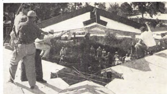
I-BEAM LIFTING RIG on a crane places 34' long panels.
