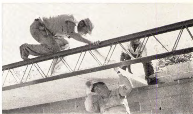
3" CEILING SLABS are set in place by hand on joist flanges. Each slab weighs 120 lbs. Ceiling finish will be acoustic plaster.
