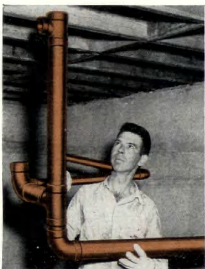
Lightweight tube and fittings make possible time-saving preassembly sections which are easily handled and can be readily put in place.
