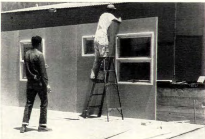
NEW SOLID CORE PANELS , joined by spline in edge grooves, form structural wall said to cost less than frame construction.
