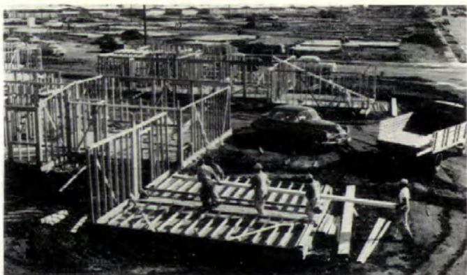
GARAGE RIDGE BEAM IS POSITIONED as soon as it is unloaded from truck to reduce later handling of heavy component. Laborers rest one end of beam on already-erected garage wall. Other end will be raised after other walls have been erected.
