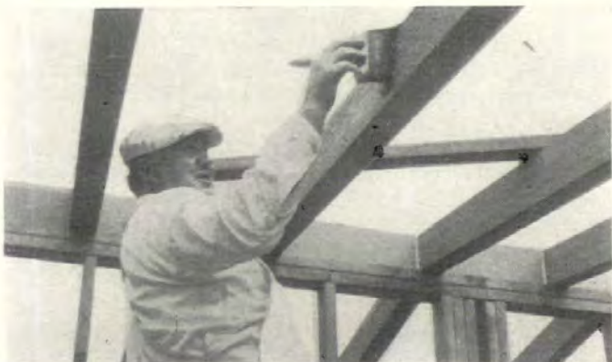
RAFTERS ARE FINISH-PAINTED before roof decking with ceiling on underside is applied. Reason: to avoid tedious paint "cuts" between rafters and ceiling. Ridge is painted later at same time as walls. Fireplaces are also completed before roof goes on.
