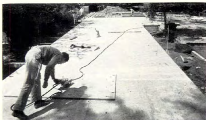
COMBINATION SUBFLOOR and underlayment is 1\frac{1}{8} " plywood over 4x4s on 4' centers with 2x4s between. Piers support the 4x4s.
