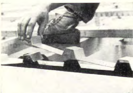
In prototype house aluminum strips were nailed to purlins with aluminum ring nails in field. Plant nailing will be faster.
