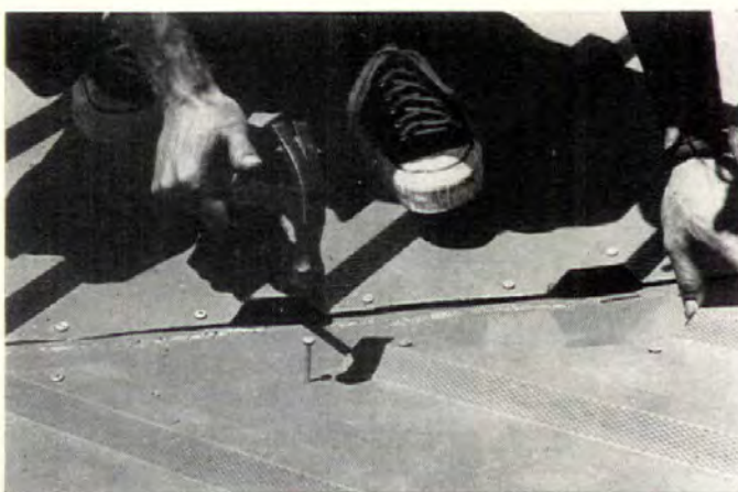
Nails holding valley sheets go through metal and rubber to plywood.
