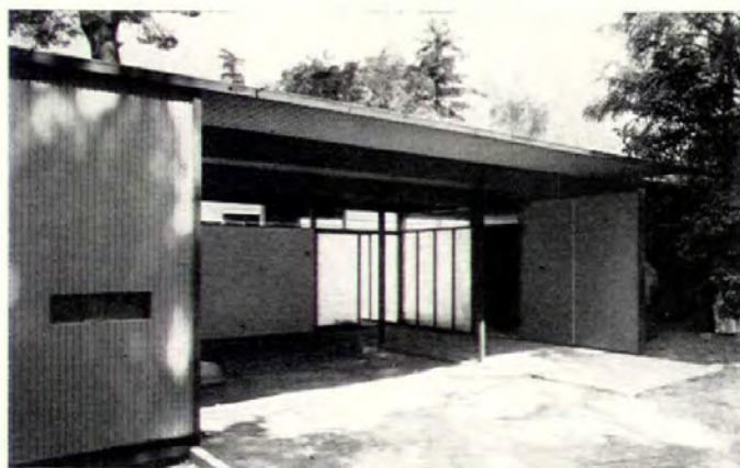
CARPORT AND ENTRY show how grooved plywood (left) and resin overlaid plywood (right) were used on exterior.
