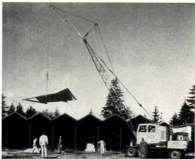
FOLDED PLATE ROOF is made up of 5'-7½" plates of plywood stiffened with dimension lumber. It costs only 80¢ per sq ft in place. Roof is supported on four laminated beams running the width of the building.
