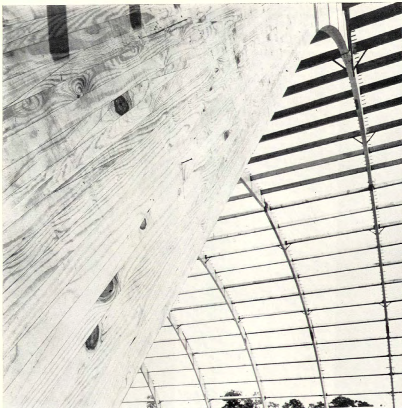
HUGE ARCH dramatizes new technology of wood structures. Laminated of southern pine, arch spans 247', is 8 stories high at crown.
