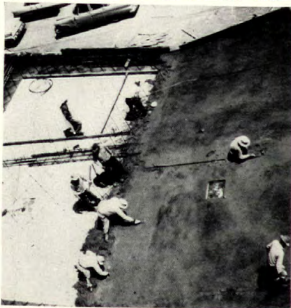
SMOOTHING went on during pouring. Retarder was used to give finishers more time. Reinforcing (left) is #3 or #4 rods 18" oc both ways, set diagonally to edges of roof.
