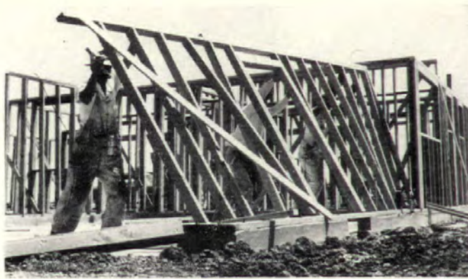
WALLS ARE TILTED INTO PLACE , then toe-nailed to sill. Sills are copper-pressurized redwood that resists moisture. Studs are kiln-dried Douglas fir. Skilled framing crews leave slab only to move from house to house. Laborers bring them materials from piles between houses.
