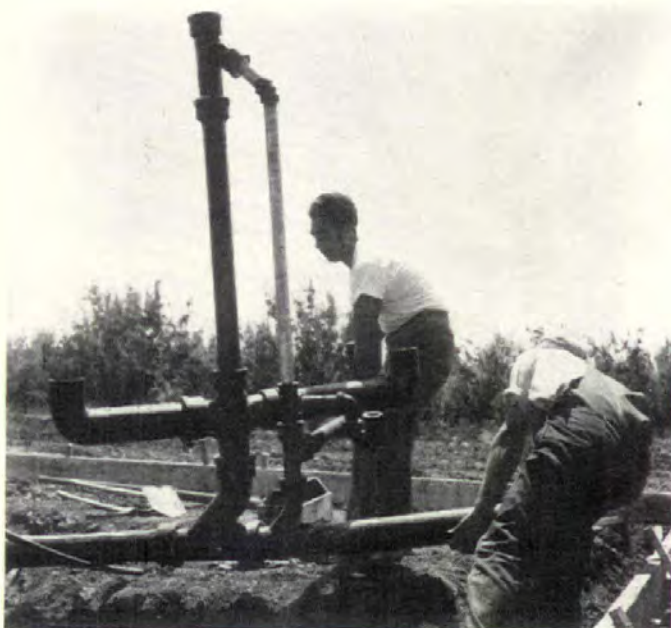
PREFAB PLUMBING TREE (left) and precut lumber (above), stacked handily on slab, save time at site. Plumbing tree, installed by subcontractor before slab is laid, is prefabricated, Branden explains, "because we can't delay slab building while pipe is pieced together at the site."
