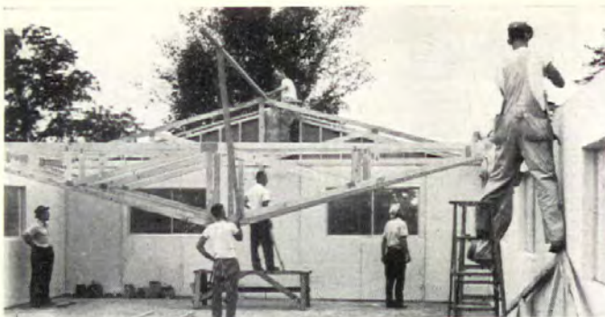
Nailed, H-brace trusses 24" o c go up fast after walls are assembled.
