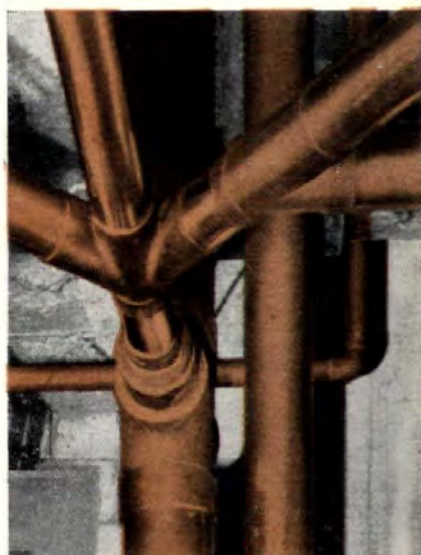
8" soil stack and 6" vent in 43-story office building. Space-saving, easily installed solder-joint fittings are a big advantage in large work like this.
