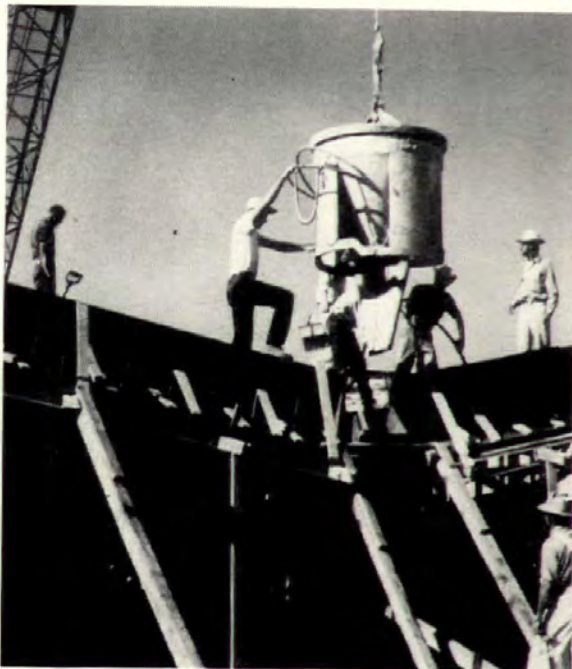
POURING of roof and columns was one continuous operation that took only six hours. Bucket was hoisted by crane. 6½-sack mix of 3,000-lb concrete with 3" to 4" slump was used.
