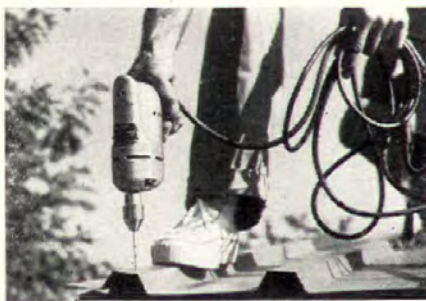
After roof sheets are in place one man drills \frac{1}{8} " rivet holes 24" apart through both the sheet and nailer strip. Ridges are 8" o c.
