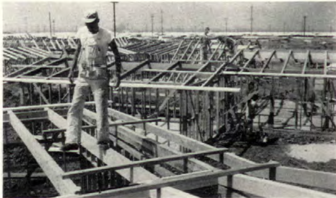
RAFTERS ARE PLACED after frame has been plumbed, blocked, and braced by special crew following on heels of rough-framers. Rafter crewman in foreground is preparing way for next crew (roofers) by spacing temporary boards on which bundles of decking will be set.
