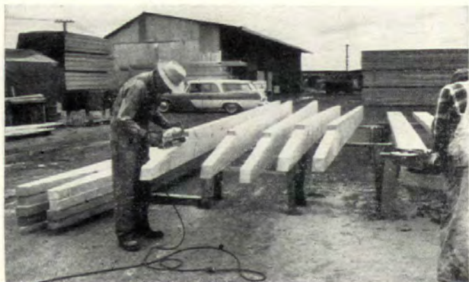
RIDGE-BEAM OUTRIGGERS are shaped with power saw at right, smoothsanded at left. These are unlaminated garage beams. Outriggers of laminated ridge beams for houses are also shaped. Architect detailed shaping simply to make exposed beams more interesting looking.
