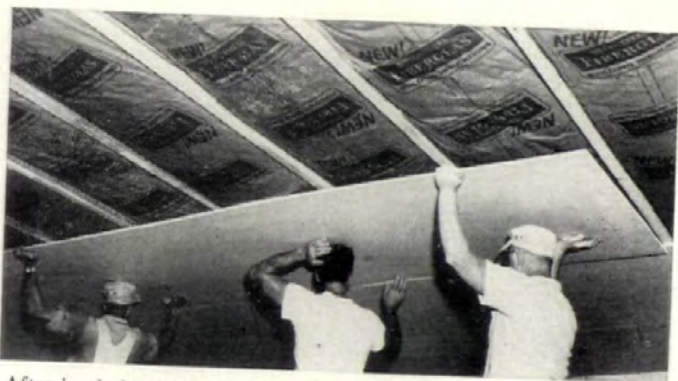
After insulation is installed the sheets of 1/2" gypsum are put up.
