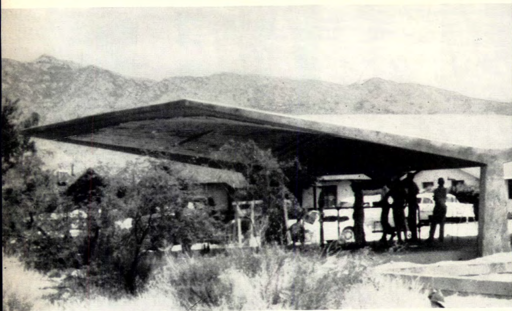
HYPERBOLIC PARABOLOID ROOF gets strength to span 50' from its curvature, not from its mass. Concrete is eggshell-thin 2\frac{1}{2} " except thicker
