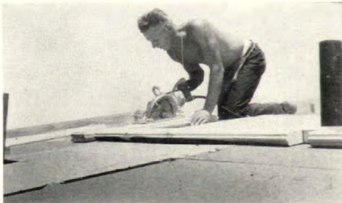
ROOF DECKING IS CUT with power saw. Portable electric generators, located between houses, supply power. Bundles of 2" t&g decking are hoisted to roof by high-lift equipment, then spotted conveniently on boards laid across rafters (see second photo, this column).
