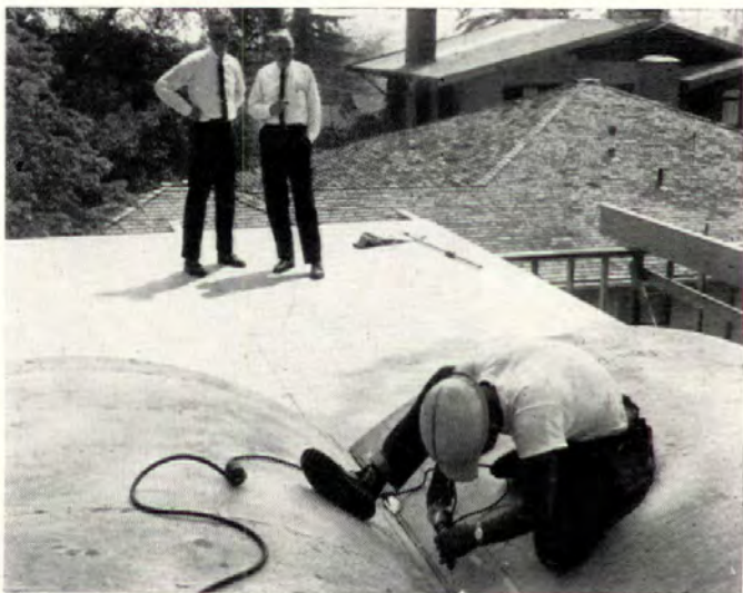
HOLES DRILLED in edges of barrel vaults position 16d nails, prevent splitting when vaults are nailed to supporting beam.
