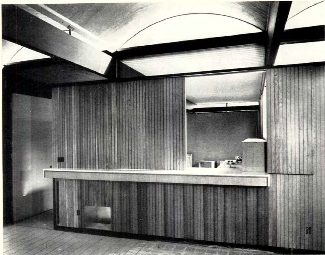
KITCHEN pass-through is framed in vertically grooved plywood. Vaults rest on chamfered beam, in turn supported on metal brackets on beam.
