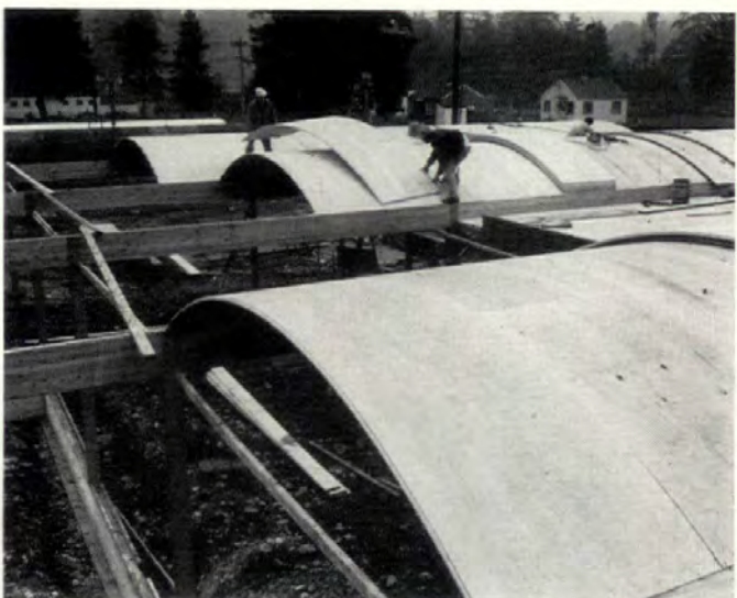
BARREL VAULTS on this building span 16', are 1 5/16" thick by 4' wide, have ¾" honeycomb core and 1 x 3 core framing between 5/16" and ½" plywood skins. Cost: $1.10 per sq ft in place.
