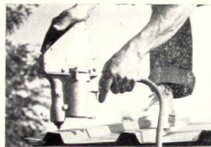
Using Pop rivets, second man rivets with pneumatic, hydraulic or hand pressure gun. Rivet heads are almost hidden.
