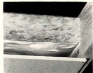
Easy-to-sell benefit for home buyer. Retains full thickness at edges. Snug fit cuts passage of heat.
