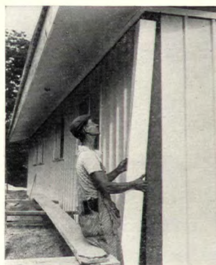
Finally pre-painted aluminum is snapped on.
