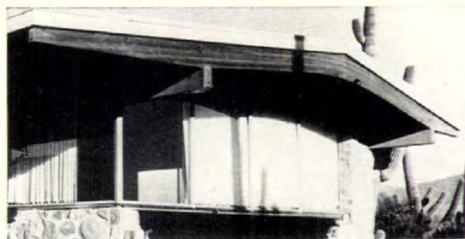
LAMINATED ROOF BEAMS on this house are 42' long, 14 \frac{5}{8} " deep. They were fabricated by Rilco. Architect: Joe Salyers, Tucson.
