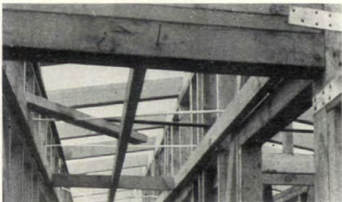
PREBUILT DROPPED CEILING GOES IN as single unit in bedroom corridor. Also prebuilt in Branden's construction yard (see p 99) are kitchen cabinet soffits, corner posts, corner crickets. Steel strapping at upper right eliminates need for toe-nailing.
