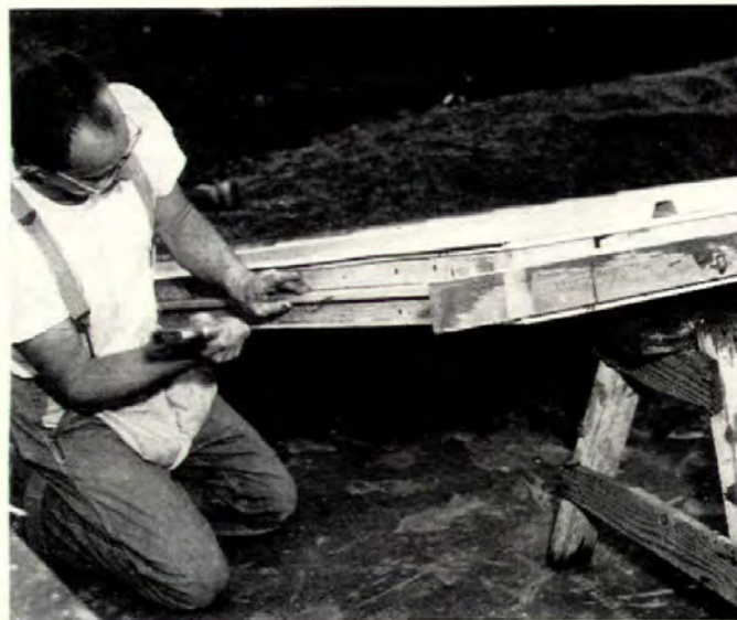
At the site a workman pushes the spline into a routed 2x4 in panel . . . Spline is then nailed in 2x4 with 8d common nails, spaced 32" o c.
