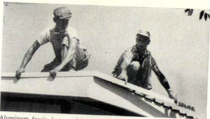
Aluminum fascia is topped by preformed factory painted corner strip.
