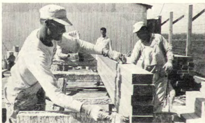
TWO-MAN PAINTING TEAM prime-coats tops and bottoms of rafters stacked six-high to save time and paint (union prohibits spray equipment). For prime-coating sides, rafters are laid close together side by side. Finish coat is applied in field.
