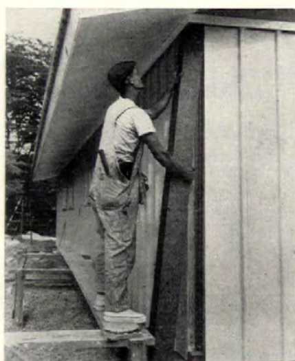
Then L-shaped fibre board cover is nailed on.
