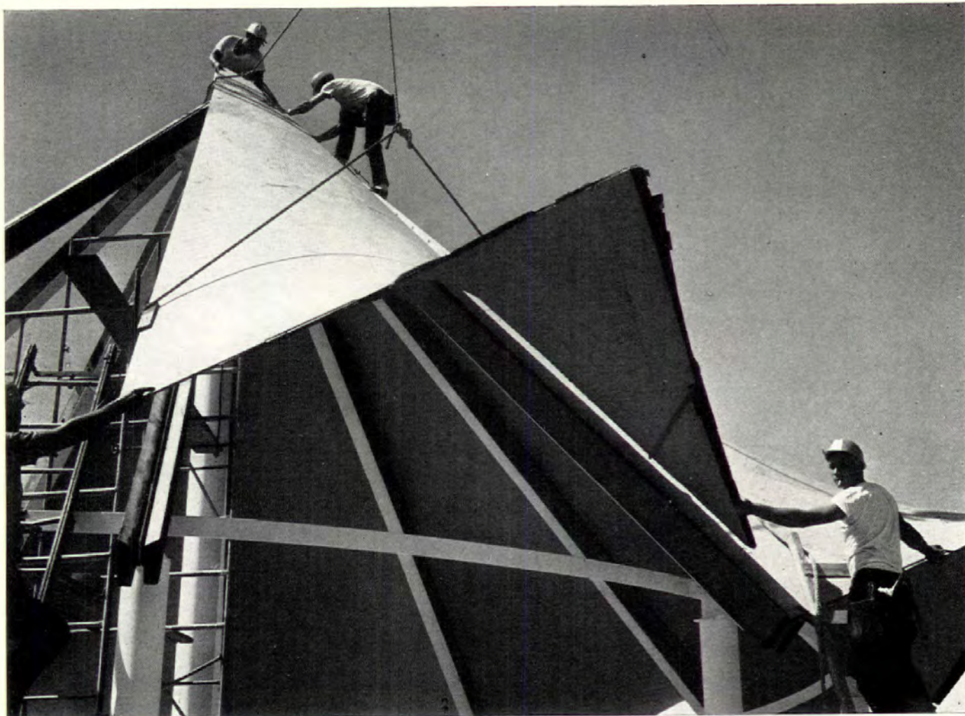
HYPERBOLIC PARABOLOID roof segments dramatize the new shapes in structural elements. Architect of this pavilion is Edward Stone.
