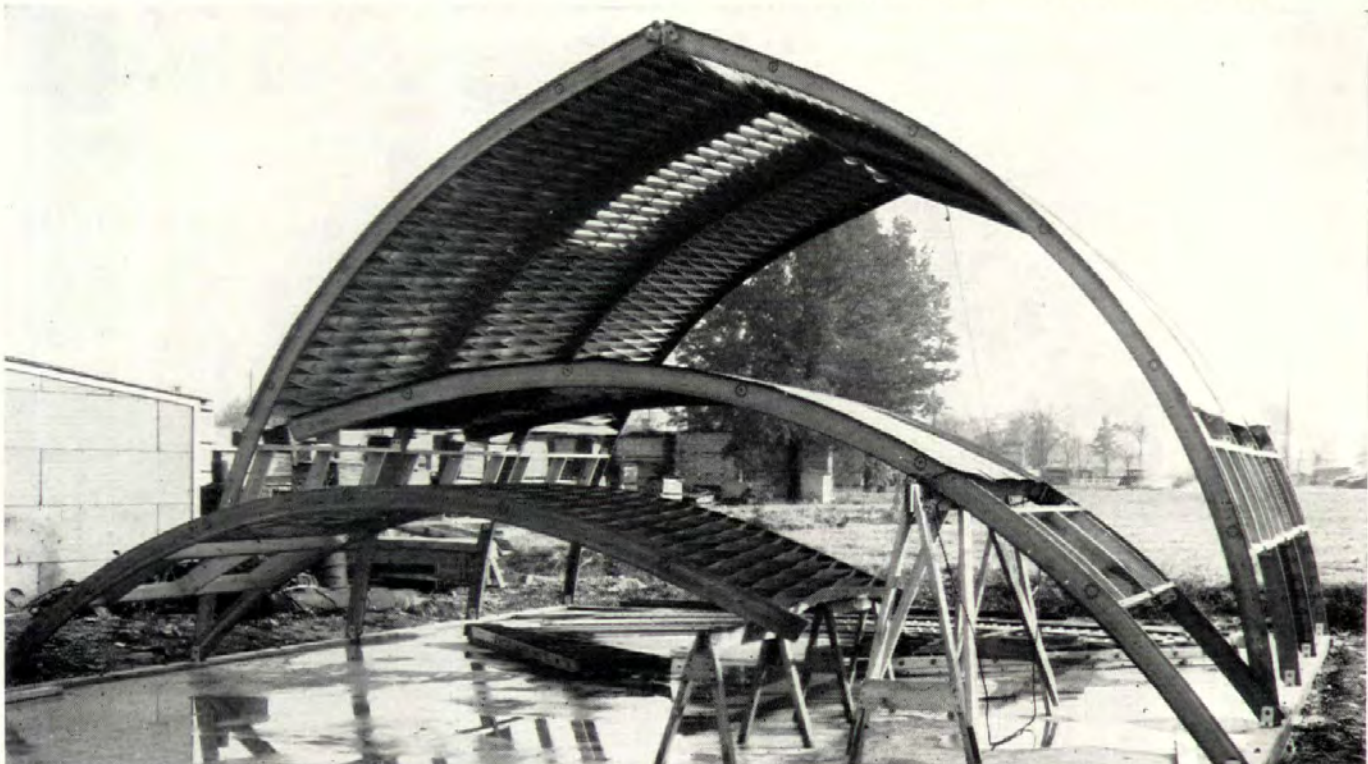
BUILDING MADE OF OAK SLAT LAMELLA , manufactured by Gamble Bros (Louisville) spans 30'. Telescoping jacks were used to raise roof sections. The lamella section, unexpanded, measures 9"x8'. When ex-
