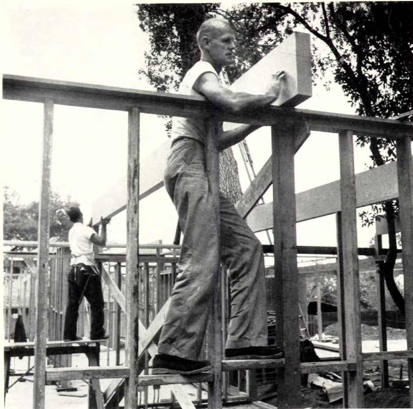
PLYWOOD BOX BEAM is easily handled by two men. Beam is 12" deep, made of two \frac{3}{8} " resin overlaid plywood skins nail-glued to 2x4s.
