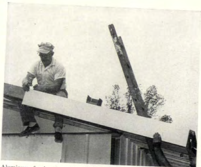
Aluminum fascia on gable-end overhang fits around wood member.
