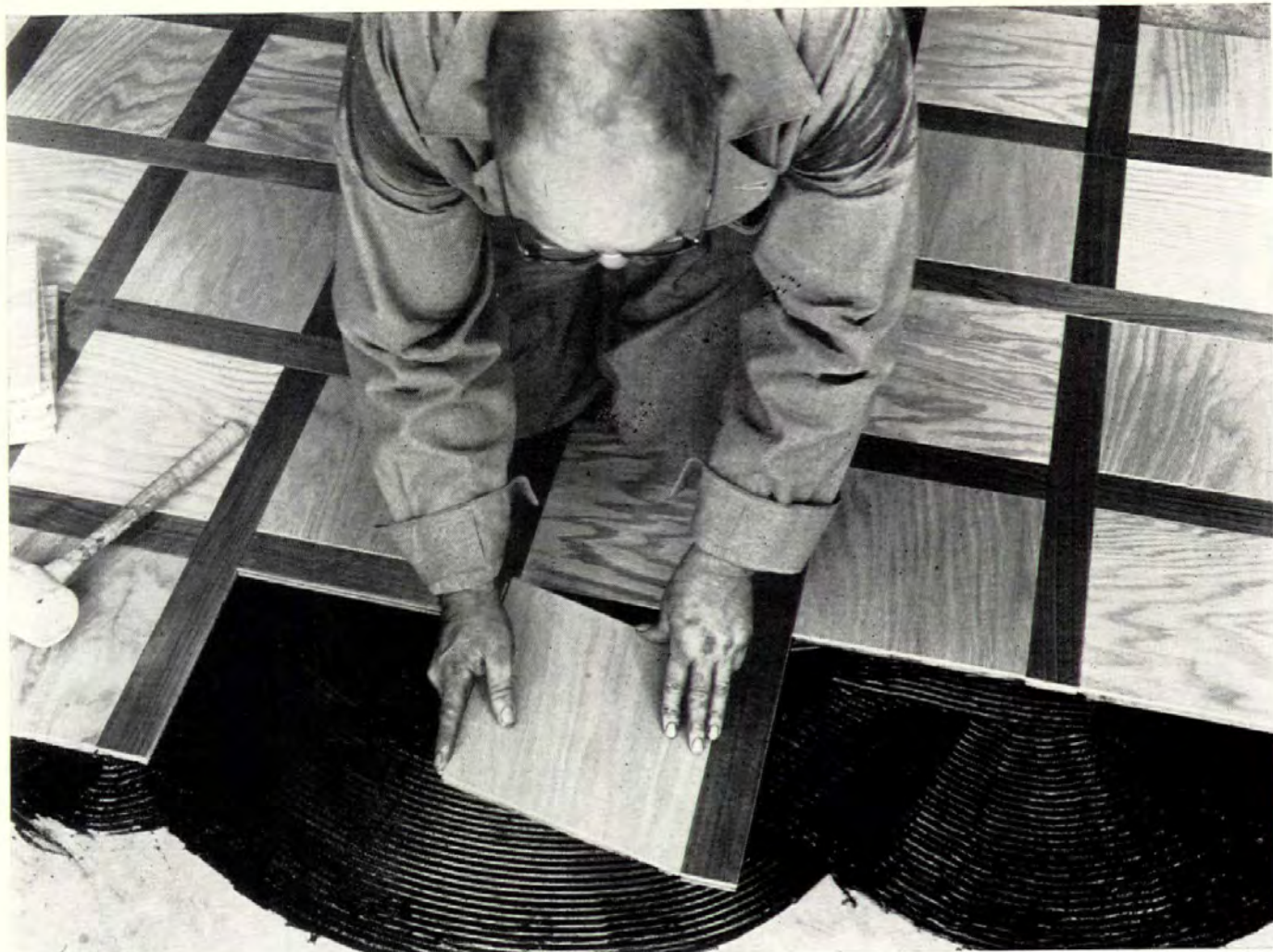
BREAKTHROUGH in adhesives is development of new elastomers for installing hardwood (here, Wood Mosaic) to concrete.
