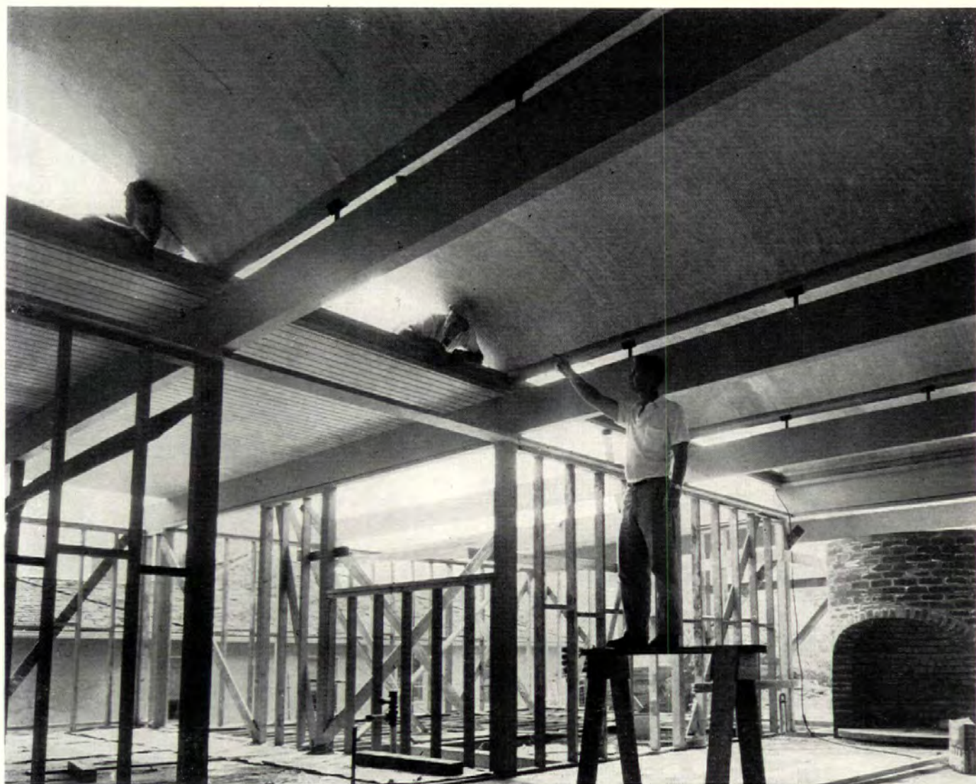
LIVING ROOM in construction shows how barrel vaults, stressed skin panels, plywood box beams work with conventional framing.
