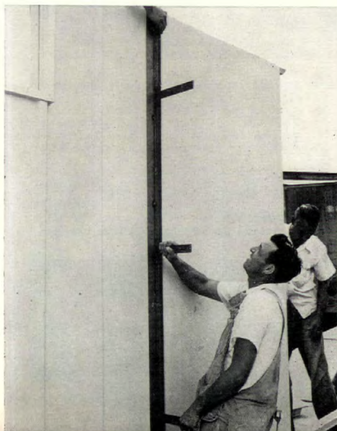
After one panel is slid over another the overlap is drilled, riveted.
