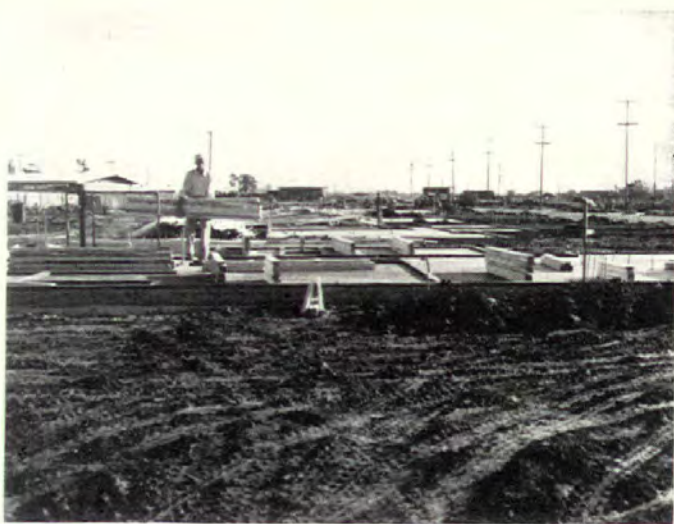
PREFAB PLUMBING TREE (left) and precut lumber (above), stacked handily on slab, save time at site. Plumbing tree, installed by subcontractor before slab is laid, is prefabricated, Branden explains, "because we can't delay slab building while pipe is pieced together at the site."
