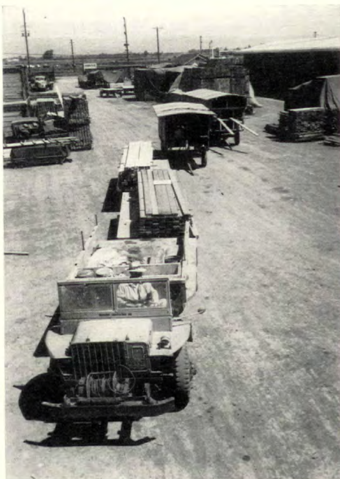
TRAIN OF TRAILERS , towed by truck, takes day's supply of lumber from yard to field. Flat-bed trailers carry framing and siding. Covered trailers, in background, carry trim. Trim trailers are left at site, reloaded with unused trim at day's end to avoid waste of costly material.
