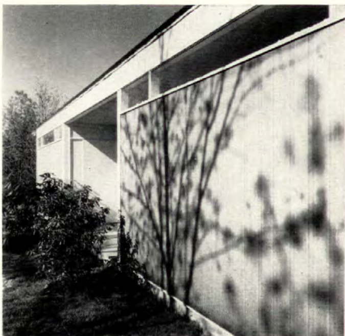
BIG PANELS finished with oils and phenolic resin for greater durability in outdoor use are coming on the market.
