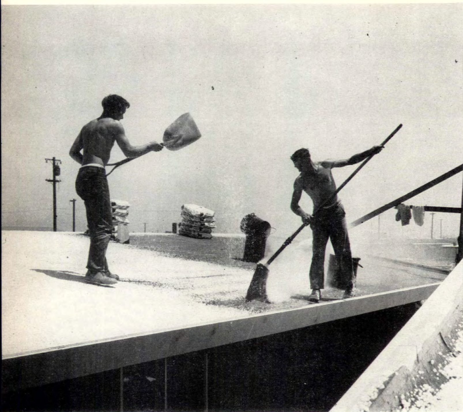
BUILT-UP ROOFING is applied to finished roof deck (see p 101). White aggregate is spread as soon as roof is hot-mopped with asphalt.
