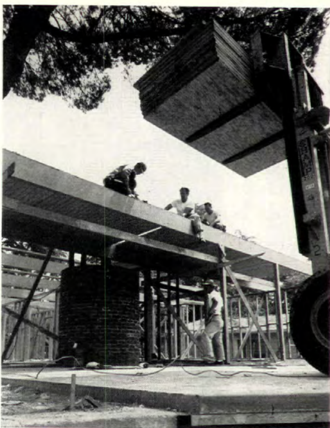
FORK-LIFT was the only piece of big equipment on the job—all of the big wood structural members are light enough to be man-handled easily.
