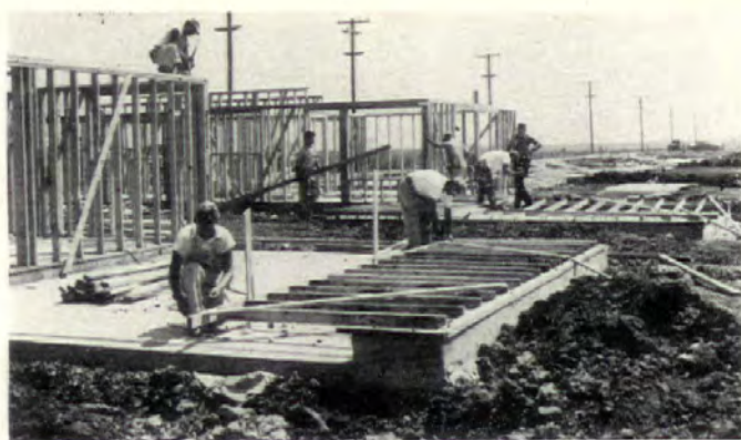
WALLS ARE NAILED TOGETHER while lying flat on slab by three-man rough-framing crew. Sills, previously bolted to foundation by another crew, have been marked to show where vertical framing goes. Branden's carpenters, assigned to specialized crews, do all framing.
