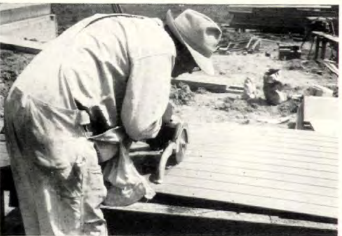
PREFINISHED HARDBOARD SIDINGS are now on the market. These smooth, surface-sealed panels make cutting, lifting, and nailing easy.
