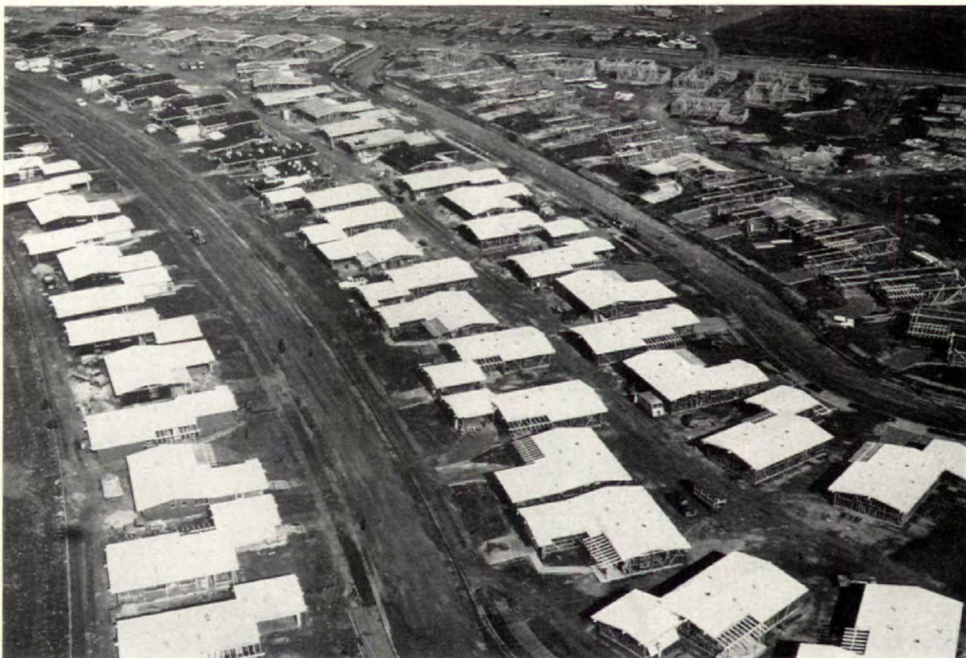
TWO WEEK SPAN , shown by aerial photo, will take the bare slabs in background to the stage of closed-in houses seen in the foreground.
