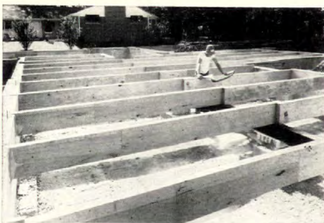
PLYWOOD BOX BEAMS used 4' o.c. in this crawl space house cost 75¢ per linear foot, reports Builder Bob Kronenberg, Hinsdale, Ill.
