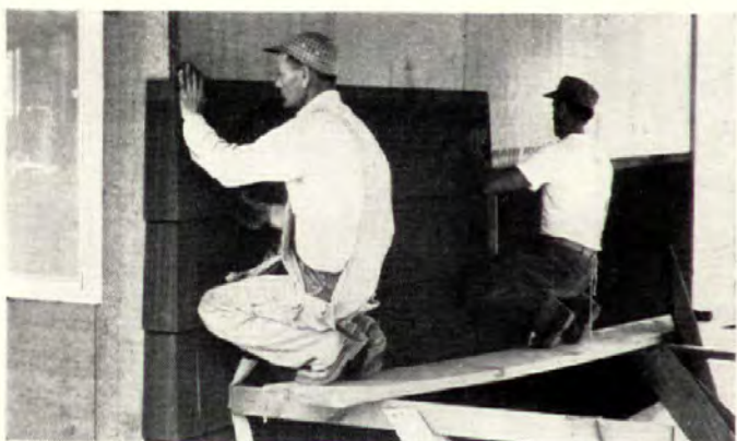
STRIATED ALL-WEATHER SIDINGS get their texture from machine grooving. Mitred corners cut materials costs, assure a neat joint.
