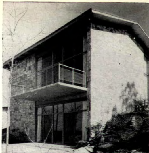
Only steel frames had the combination of strong yet thin sections which made this design possible.
