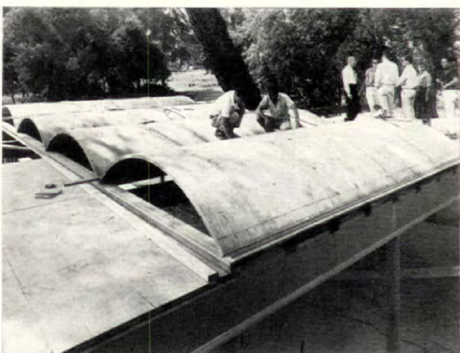
OPEN ENDS of the barrel vaults over the living room will get fixed glass, so from inside they give the same high open feeling as clerestories.
