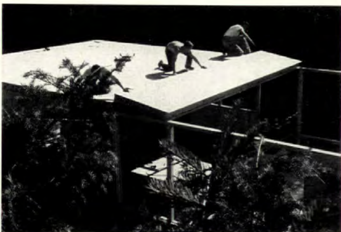
STRESS-SKIN PANELS form roof, walls and floor in 20' x 40' house erected by five men in 7 1/2 hours. Architect: Edward L. Cushman.
