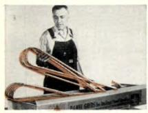
Machine-formed PG's are furnished ready to install. One tube end of each panel grid is expanded so that it can be solder-connected in series without requiring fittings.
