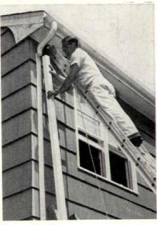
Downspout pipe slips over the end of the elbow then snaps in place in the wall channel.
