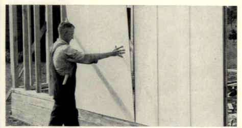
Sheathing and siding are one in Upson's Dubl-Bilt, a ¾" fiberboard made of two ¾" laminations. Dubl-Bilt comes plain or primed—off-white on the face for a better paint base,
