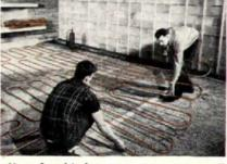
Heat for this basement game room will be provided by ½" PG's embedded in a concrete slab. For floor or ceiling radiant panel heating systems, Anaconda PG's offer many installation economies.
