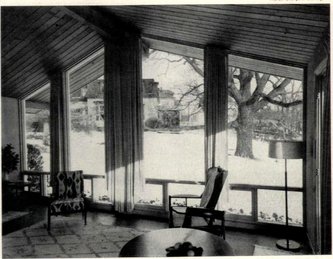
LIVING ROOM ROOF (a) has no tie beams or rafters. Large sections of glass extend from venting units to roof deck (3x6 t&g Douglas fir).
