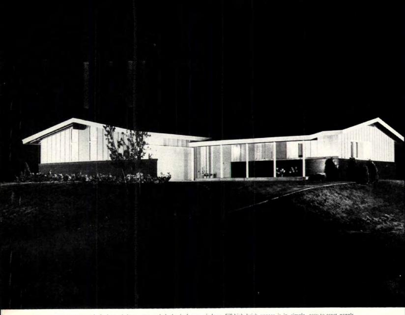
FRONT PORCH is 5' deep, shelters entry and shades bedroom windows. Sill-high brick veneer is in simple, easy-to-erect panels.
