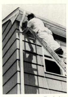
Downspout is in two parts. Here the downspout channel is nailed to the side of the house.
