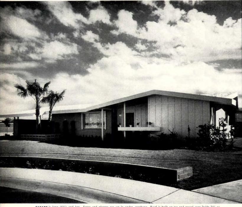
FACADE is long (64') and low. Entry and planter are set in under overhang. Roof is built up tar and gravel over 2x10s 24" oc.
