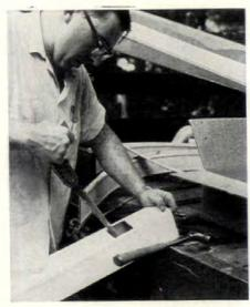
Hole for drop outlet is cut in the plastic gutter with a keyhole saw or tinsnips.
