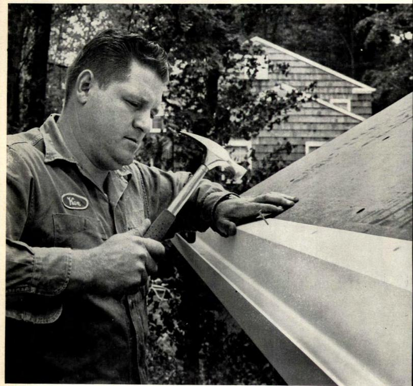
EXCLUSIVE FLASHING FEATURE! No other gutter has its own flashing that fits right under the first row of shingles. Eliminates the need for a drip edge. Saves time, money and extra labor!
