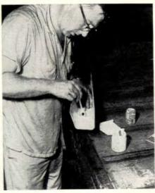
Gutter opening is coated with epoxy resin to make a permanent bond with the drop outlet.
