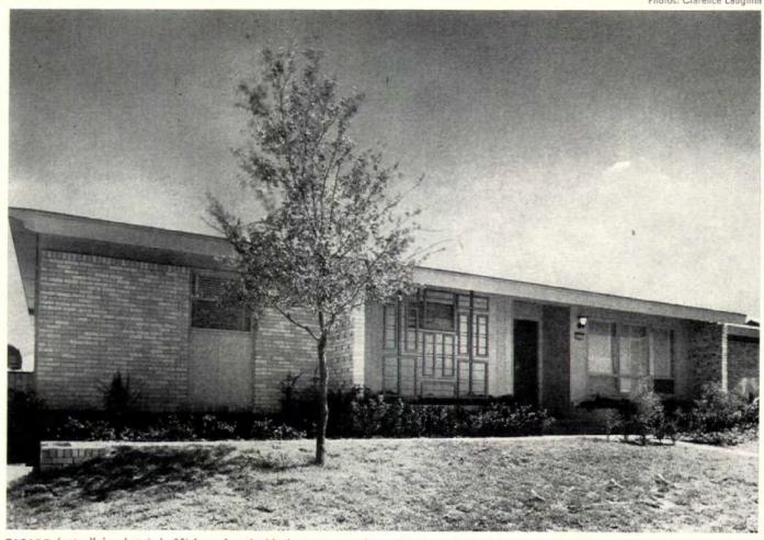
FACADE (not all in photo) is 85' long, has double-door entry set in under 4' overhang, brick veneer in big easy-to-build sections.
