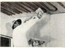
No sags or dips in the tube lines. PG's are uniform and fasten snugly to ceiling construction permitting a uniform thickness of plaster with resulting savings in materials and time.
