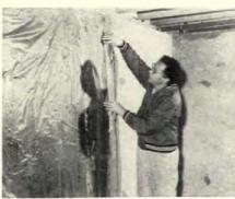
Adhesive for polyethylene, Bondmaster Z377, takes hold fast to give permanent moisture control on concrete, wood, or any porous building surface. The new material is a trowelable synthetic rubber with a tack life of two hours—an entire foundation can be coated at once so the polyethylene can be applied in a continuous sheet with resulting savings in time and labor. Adhesive should be applied at least 18" from the top and bottom of the wall; the rest can be spot tacked to save adhesive.
