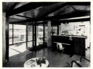
**LIVING ROOM** (a), open to screened loggia and kitchen (rear), has plank ceiling laid on specially designed, exposed trusses (see facing page for details). Ceiling in separate bedroom wing is flat.
