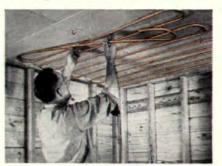
Hook-type fasteners of nonrusting Everdur, \*\* also offering easy, fast installation, are partially set in joists—PG's slip over hooks. Fasteners are driven to draw tube to ceiling.
