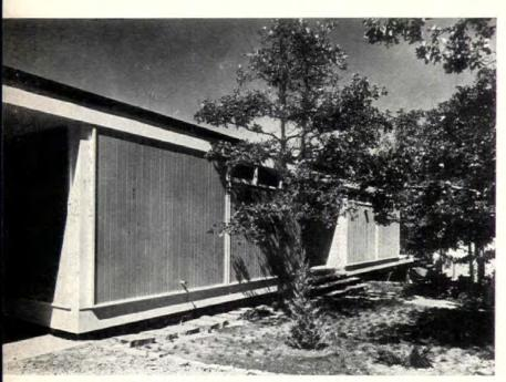
**SOLID WALL** and carport at left screen interior from street. House seems to float because it is cantilevered 2½' over foundation to reduce joist span. Post-and-beam construction is based on 11' module.
