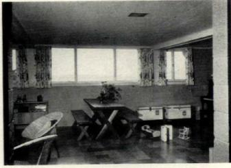
**LOWER-LEVEL RECREATION ROOM** (c) is below living room, shares view of lake. Room is free of supporting posts because it is spanned by steel beams. Acoustical-tile ceiling holds down noise.
