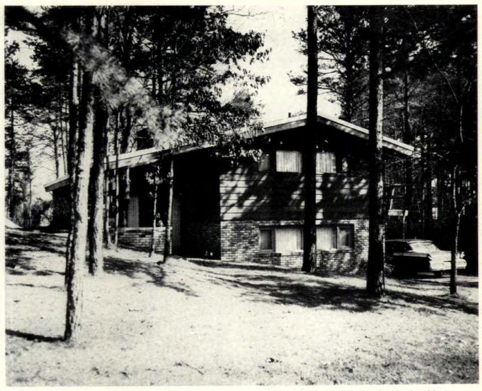
FRONT VIEW shows how pitched roof, sloping down over living room at left, holds design together. Siding is redwood and used brick.
