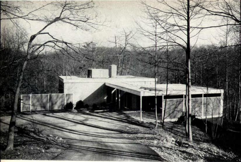
UPHILL SIDE faces driveway. Carport and entry walk add length to almost square house. Boxlike structure on roof encloses fans, skylight.
