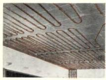
Ceiling installation on gypsum lath. Note changes in spacings— $4\frac{1}{2}$ " centers near the outside walls where heat loss is greatest but with the c-c spacing increased at the center and inside areas.
