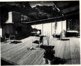
BIG DECK (a) with fireplace is protected on three sides—by carport at left, ramp wall at rear, and house itself, out of photo at right. Floor is 2x4s-on edge and spaced to let water run through.
