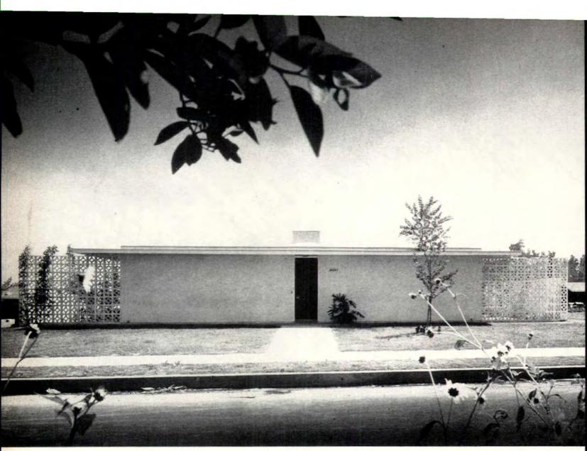
SIMPLE, CLASSIC FACADE is set off by pre-cast concrete grilles that extend to lot lines. Exterior walls are stucco over 2x4 framing.
