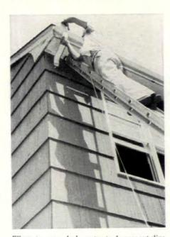
Elbow to carry drain water to downspout slips easily on the drop outlet. It is not bonded.
