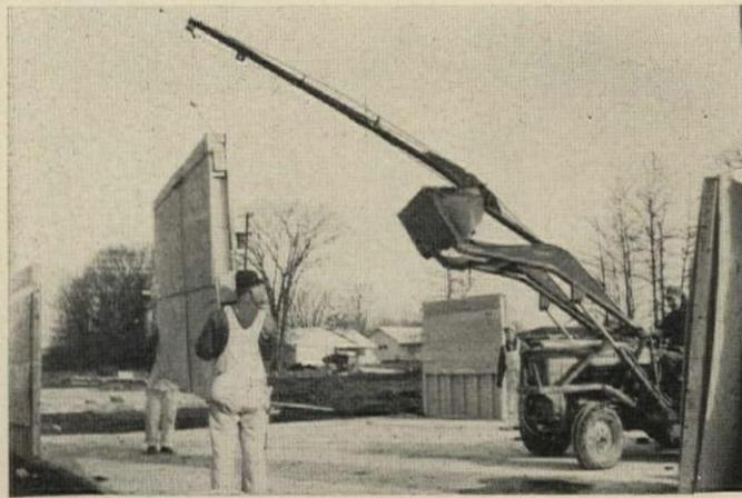
**PANEL IN AIR** will be dropped into final position on sill where nail had previously been driven in to indicate center. Double-glazed windows in panels are protected from breakage by sheets of plywood. Plywood is removed and used for sidewall sheathing on blank wall sections, made at site with precut studs.
