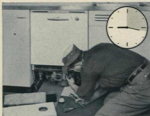
**9:17** Connect utilities. Easy-to-reach plumbing connections are made in front on left; wiring on right.
