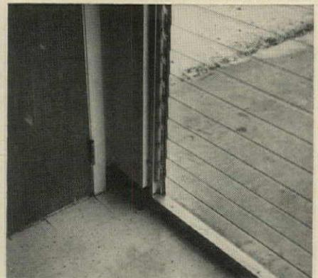
**WINDOWS** are floor-to-ceiling glass louvers set in panel-size bucks and 4' high louvers over 4' high panels. Sills of the bucks are fastened to plates anchored to the foundation.
