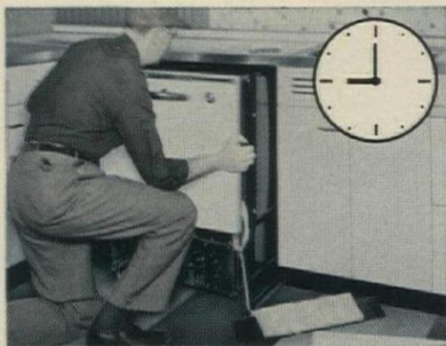
**9:00** In a typical base-cabinet opening (24" W x 34½" H x 24" D) with plumbing and wiring roughed-in; slide unit into position.
