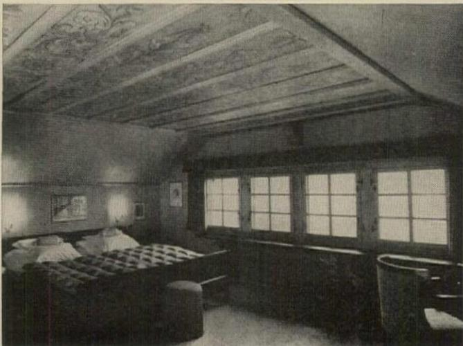
**Decorated ceiling** is over bedroom in chalet Bärghlamm (Gstaad), built in 1647. Battens are 1/2 meter (approx 20") oc, were milled from 2"x4" stock. The traditional flower and foliage pattern is painted on the panels in soft pastel tones. Bracket at right extends up to ridge, and out to deep gable overhang. Note traditional hardware on windows.
