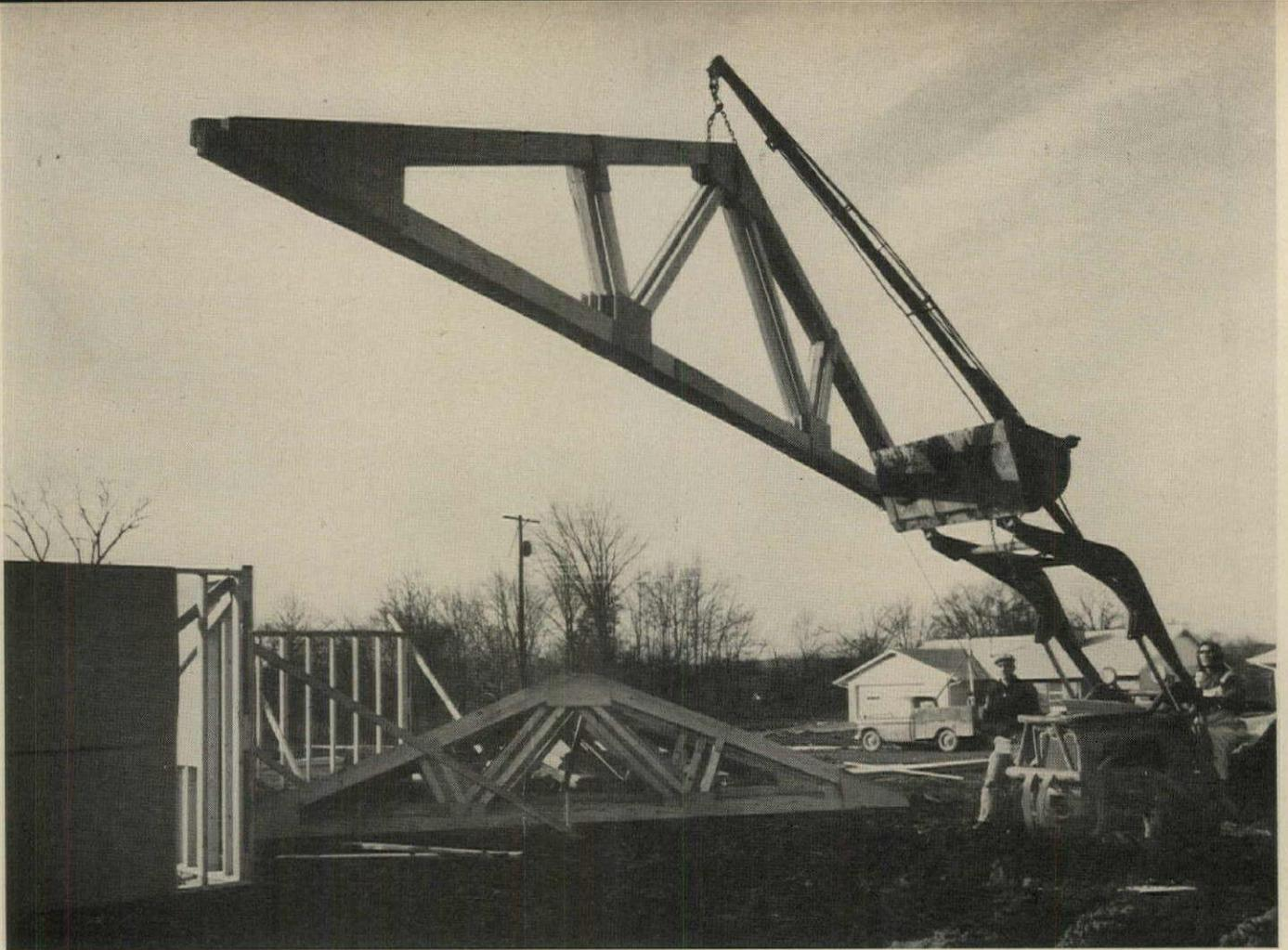
**THREE TRUSSES IN AIR** were lifted from upright stack near house, will be set onto top plate of exterior wall in one pass.
