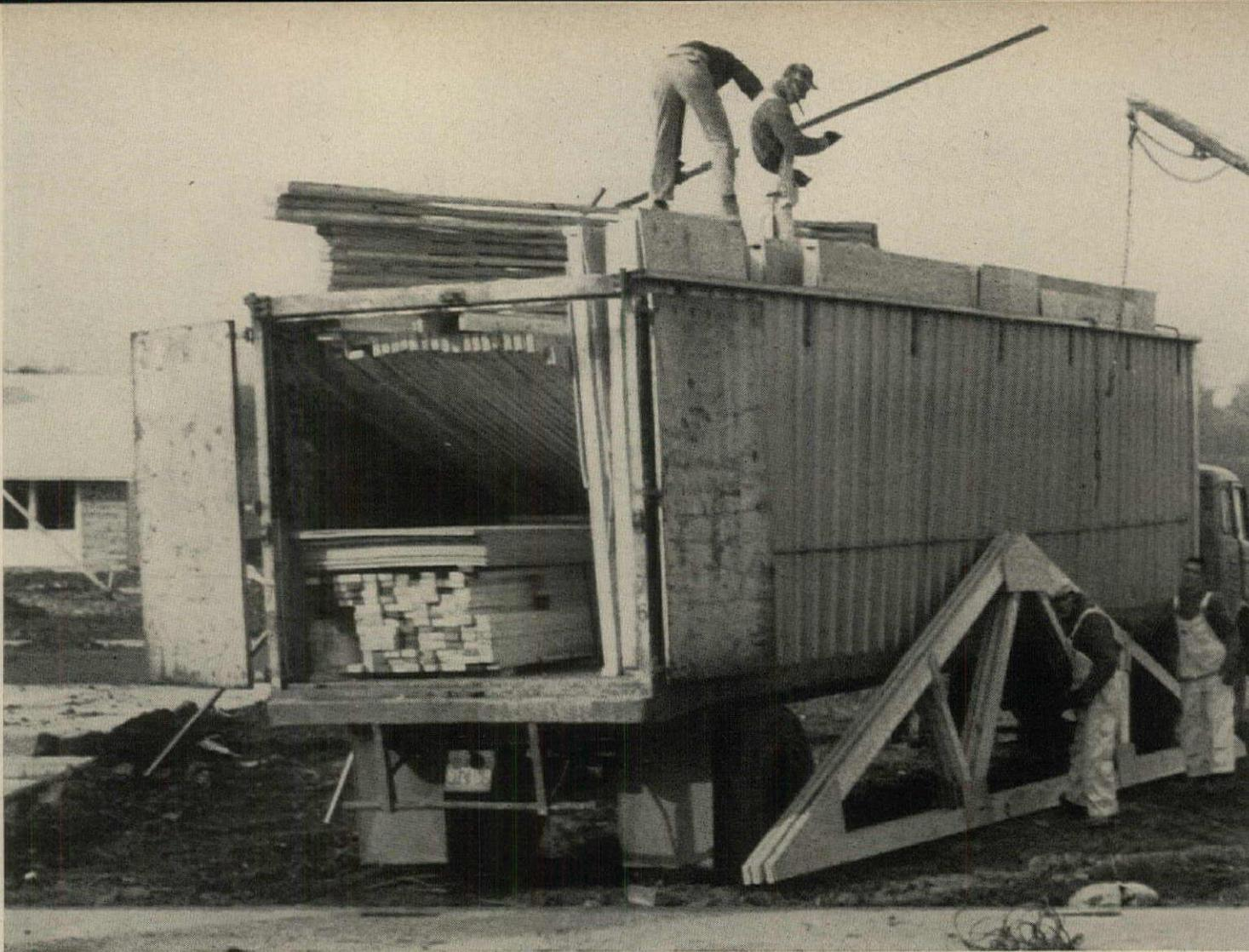
TRAILER-LOAD of components, plywood, and precut studs for a house is backed into "L" of slab to get materials close to point of use.
