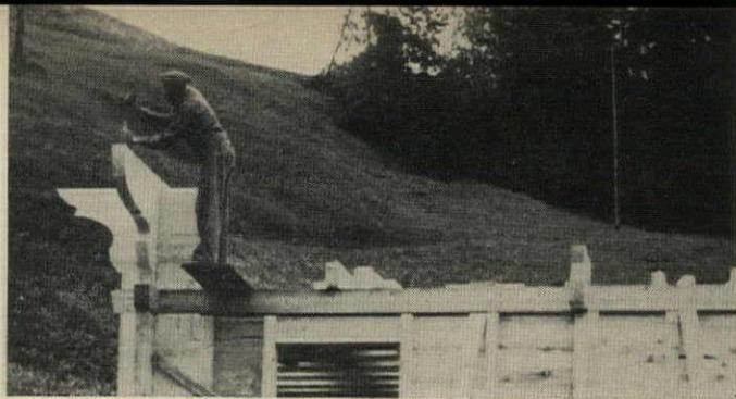
**ROOF BRACKET** is assembled and fastened with dowels on top of walls.
