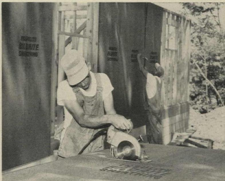
Easy sawing, easy nailing are two more great virtues of Bildrite and Graylite. You will actually save one or two sawblades on an average house, because Insulite has no lumps or gummy spots. Application time, compared to lumber, is up to 40% faster.
