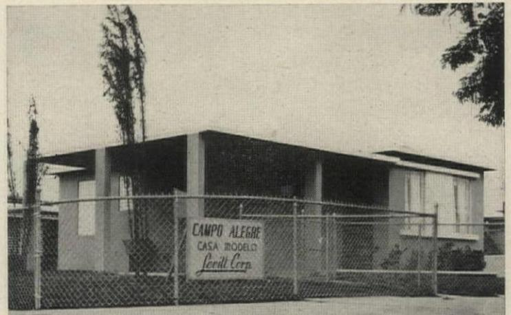
**LEVITT'S MODEL** is adapted to Puerto Rico building methods (i.e. reinforced concrete walls), rapid construction. Levitt expects to complete five a day when construction gets rolling.
