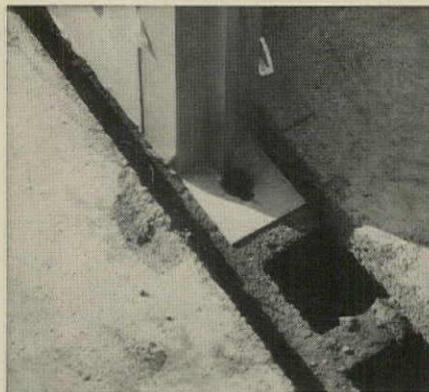
**COLUMNS** between exterior wall panels have welded base plate held by anchor bolts to block foundation. Panels sit between columns, are not tied to foundation (see opposite).
