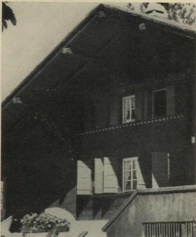
**Gable overhang** on Chalet Bärglimatt is 8' deep. It is supported by huge bracket spanned by purlins. This chalet is now roofed with shingles, but originally had a slate roof. Rocks are often placed on chalet roofs to hold them down in strong winds. The 25° roof pitch keeps snow on the roof for insulation (chalets were not well heated until recently). The deep gable overhang protects the end walls, with all their joints, from the weather.
