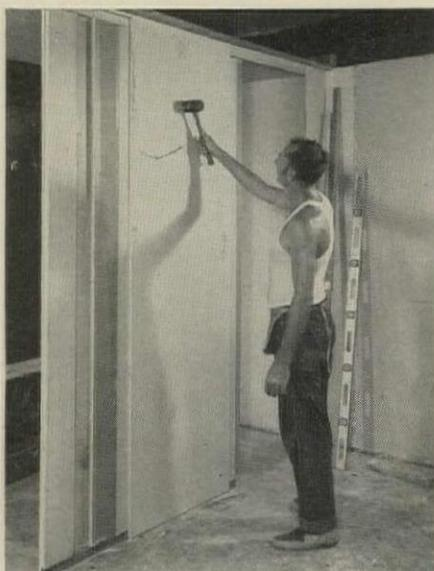
**OTHER DRYWALL FACE** is glued up to ribs, nailed top and bottom to complete job.
