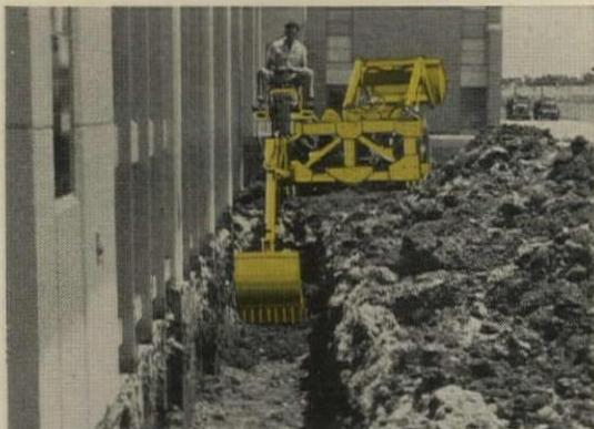
The Davis Backhoe is the only machine that will dig flush. 200° continuous operating arc lets you dig or dump to either side and never get cornered.
