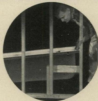
3. Patented wall-hung installation. Exclusive anchor lugs hold the tub firmly in position, absolutely eliminating separation of bathtub from wall after it is installed. 1" wall flange eliminates seepage into wall.
