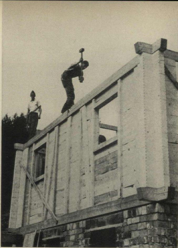
**WALL PLATE** is interlocked with partition (seen through window), then fastened with dowels, shown being hammered in. Partitions are plastered. This stage marks end of second day of construction.
