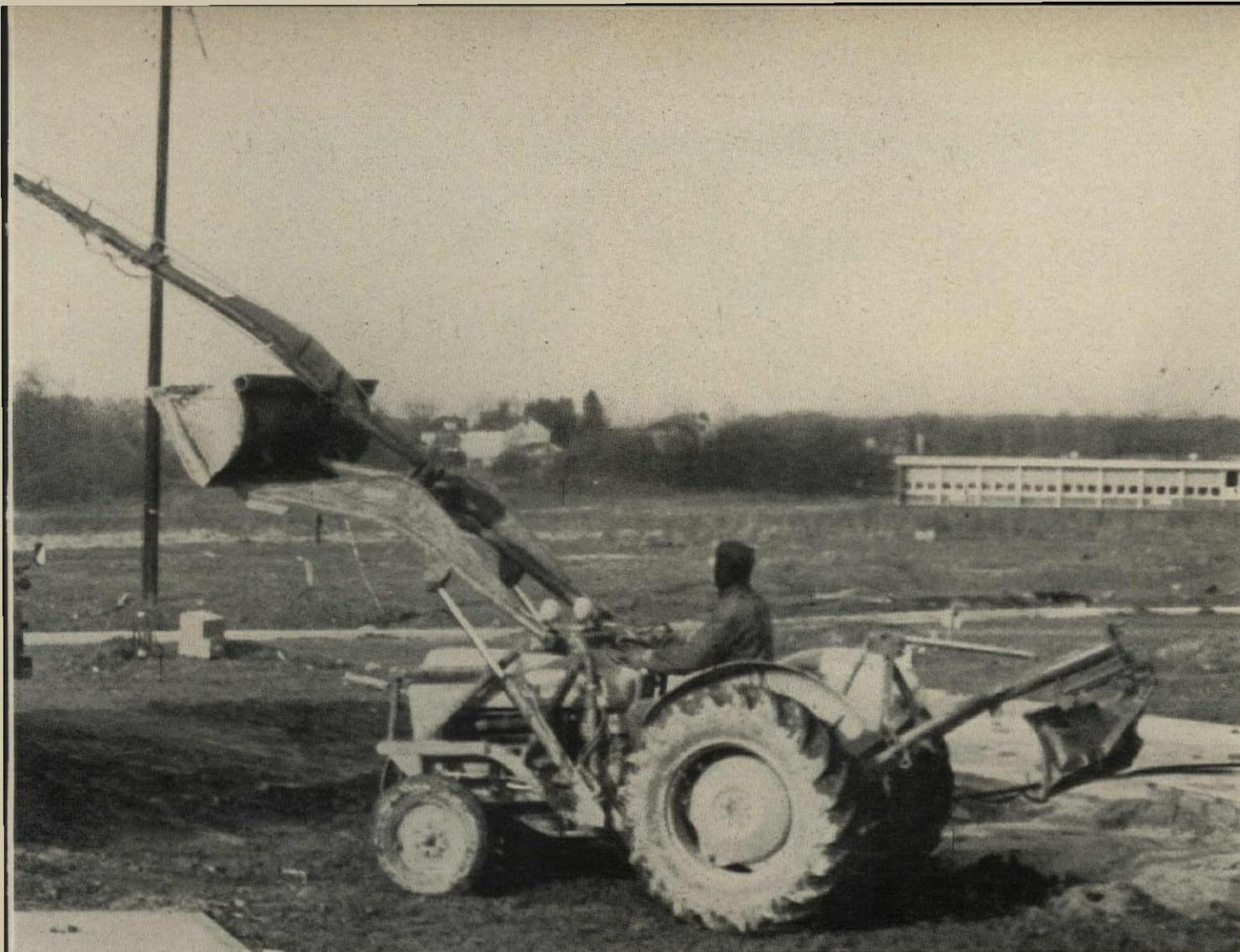
**BOOM** attached to high-lift tractor lifts trusses from top of load, sets them upright at sides of truck; later sets panels directly on slab.
