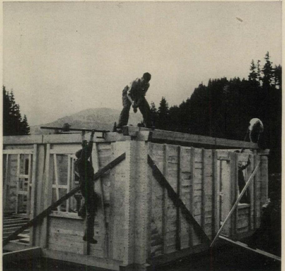
**TOP PLATE** is driven home on top of wall. Lower man in foreground is tilting a header already in place so that notches in it and wall
