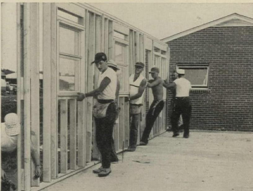
**Saves time, materials!** To install Strutwall, Fister-Seeberger workmen simply cut two load-bearing side struts to fit header. Nail in place. Tilt up with wall. In multiple openings, Strutwalls are butted against each other. This eliminates need for anything heavier than two 2 x 6 headers in single story construction.
