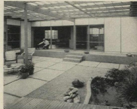
**COVERED PATIO** in Ryan house is sheltered beneath reinforced plastic roof supported by rafters.
