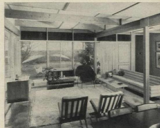
**DOUBLE 2x10's** form beam supporting exposed joists in the living room of a \$21,000 Ryan house.
