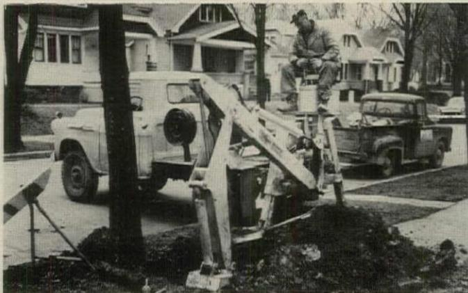
**Ottawa Model LX backhoe** fits many makes of trucks and tractors, digs to 12½' depths in any position on a 190° arc. Patented ejector bucket speeds work in muck, quick on-and-off mountings make for economical use of equipment. A front-end loader works off the same hydraulic system.
