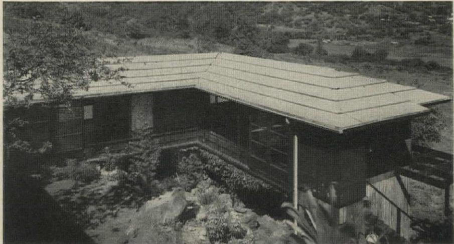
**L-SHAPED HOUSE** stands on posts that lift it above its sloping site. Use of posts is characteristically Japanese. Grey mineral roll roofing is nailed over batten strips, which give pattern and interest to the low-pitched roof.
