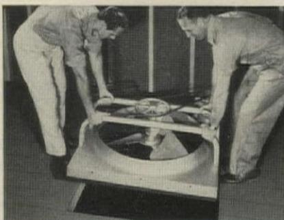
**1.** In normal installation, R&M-Hunter Fan (Package Type) is placed on attic floor with automatic shutter in hallway ceiling.
