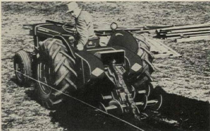
**Auburn trencher** is designed to work with Massey-Ferguson tractors. Variable hydraulic drive adjusts tractor speed to ground conditions. Unit will take trenching chains 6", 8", 10", 12", or 14" wide and booms up to 6' long. Hydraulic boom operates in 190° arc to control depth or backfilling under sidewalks, streets, etc. Auger-type conveyor spills dirt equally to each side. Special Pent-A-Bits are available for digging in rock, shale, or frozen ground.
