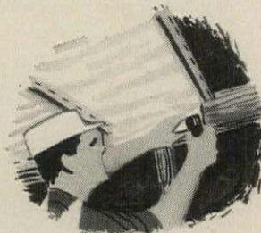
Fold ends of blanket and fasten to sill plates on either side, sealing the insulation. Fold the flanges over the face of the studs to close the edges. Final seal is made when gypsum board is applied.
