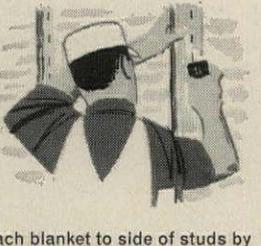
Attach blanket to side of studs by staples not more than 6 in. apart to form a  $\frac{3}{4}$ -in. air space between vapor barrier and gypsum board.
