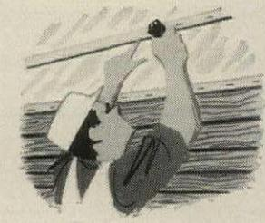
Staple flange to inside surface of next ceiling joist.
