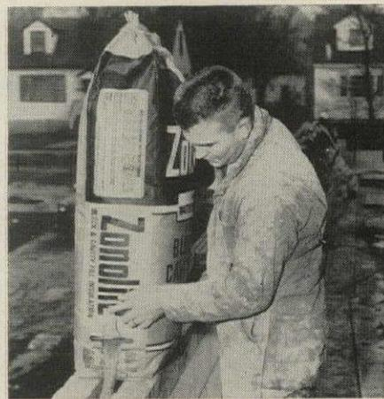
**Zonolite insulation** is claimed to improve U factor of an 8" cinderblock wall from .39 to .20 for only 10¢ a sq ft of wall area. Expanded vermiculite is water-repellent treated, will not hold moisture, set up capillarity, or compact through settling. A 4-cu-ft bag will fill 16 three-core 8" blocks or 14½ sq ft of wall. Bags are tabbed for easy pouring.
