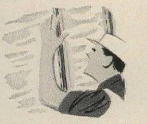
Fold flanges over the face of the studs to close the edges. Final seal is made when gypsum board is applied.
