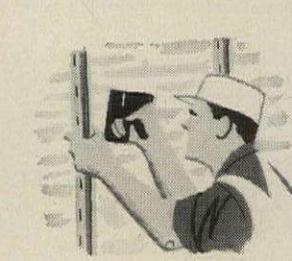
Follow same procedure for wall insulation, except that air space between gypsum board and foil vapor barrier should not be more than  $\frac{3}{4}$  in. Top and bottom of blanket are usually secured first.
