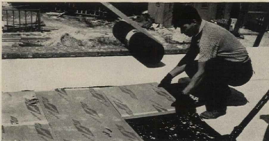
**Dow roof insulation**, called Roofmate, is Styrofoam plank wrapped in laminated kraft paper. Boards are 2'x4', and may be 1", 1¼", 1½", or 2" thick. Light weight, high compressive strength,
