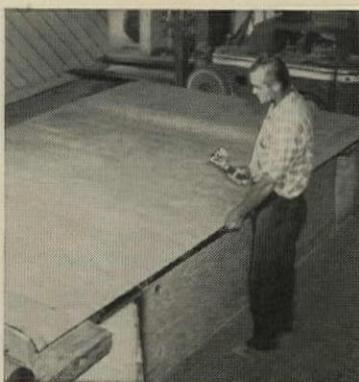
Men in shop staple aluminum vapor barrier in side-walls in a quarter hour. This was a one-hour chore with hammer and nails. At an average of 10 panels per house, builder puts an additional \$16.88 in the profit column on each house.
