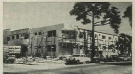
California builders stop stucco short of ground to prevent hydrostatic action.
