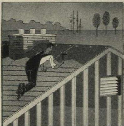
For the sloping roofs of this apartment house development J-M COLORBESTOS® Shingles are specified. Made of asbestos and cement, they are rigid and stonelike, require no maintenance and give lifetime protection. J-M AQUADAM Built-up Roofs recommended for the flat roofs (viz. center building) are bonded for 20 years of satisfactory service.
