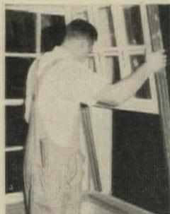
\*Pre-installed Snap-Clips let you remove and replace both window sash and Dura-seal at any time during construction!
