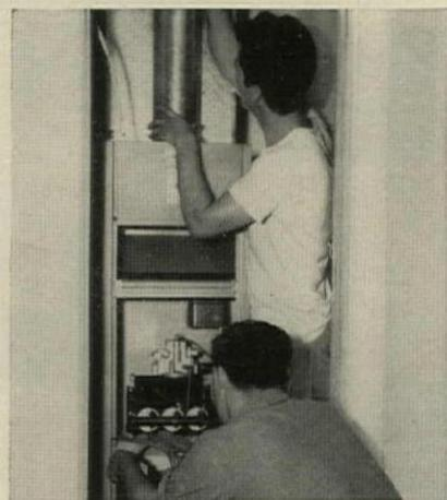
**Two-man team** installs complete unit and ducts in six to eight hours. This gas-fired American-Standard furnace—the G.U.B. 75D—delivers 75,000 B.T.U., requires an area only three feet square. Entire unit is easily accessible for adjustment.
