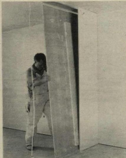
**STAGGERED JOINTS** are assured by starting one face with a half sheet. All edges fall at a spacer strip, are bonded with joint cement. Spacer is 8" shorter than wall.
