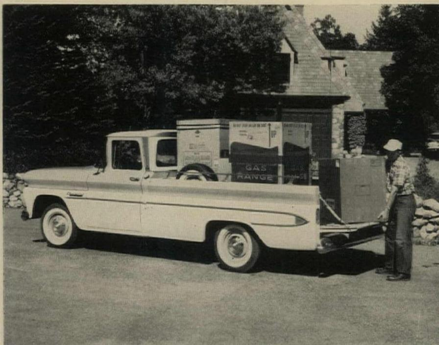
**FLEETSIDE PICKUP** is low to ground, has step-in cab with full-width floors. Cab structure is rubber mounted. Brake and foot pedals are suspended; steering is relay type.
