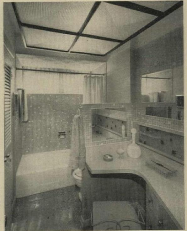
**MASTER BATHROOM** has suspended luminous ceiling with corrugated plastic panels and wood framing (see details, next spread). Fixtures in both baths are by Crane.
