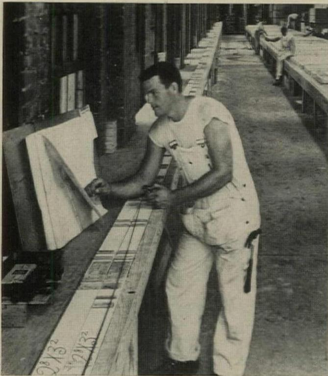
**PATTERN STRIPS ARE LAID OUT** on long table. Working from blue-print, carpenter tacks down blocks to show where framing members go.
