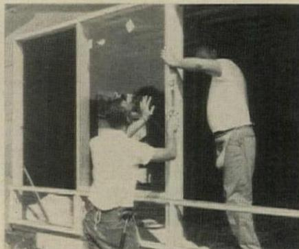
**CENTER PICTURE WINDOW** is installed after the three awning sections. Here it is leveled and plumbed before being nailed.
