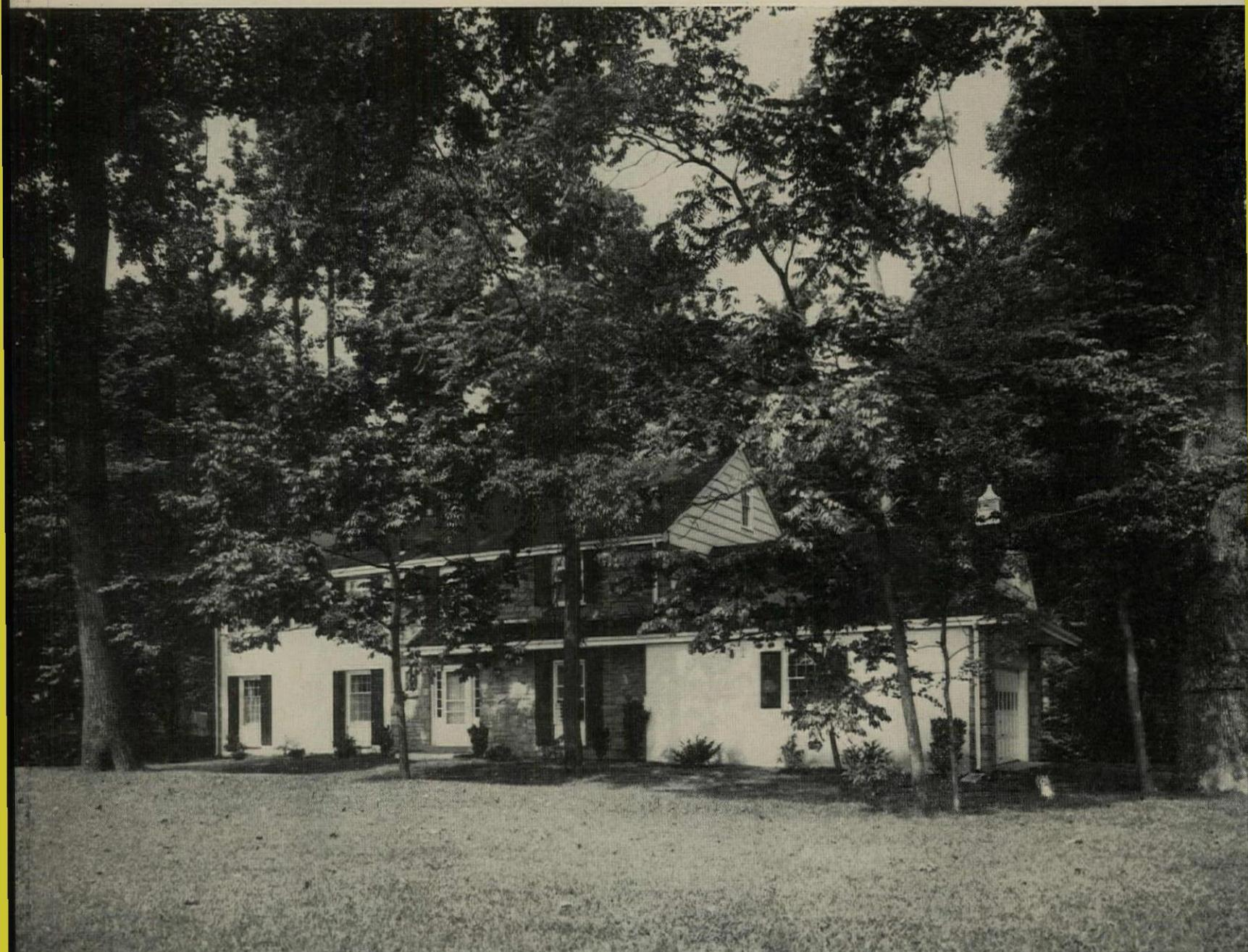
**TRADITIONAL HOUSE** spreads 74' across the lot. House is concrete block, with stucco and stone veneer. Roof is J-M asphalt shingles.
