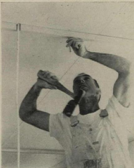
**NAILING STRIPS** 1" x 1 1/2" on ceiling, floor, and sidewalls locate and hold partition. Wiring leads are dropped through ceiling, sandwiched between wallboard faces.
