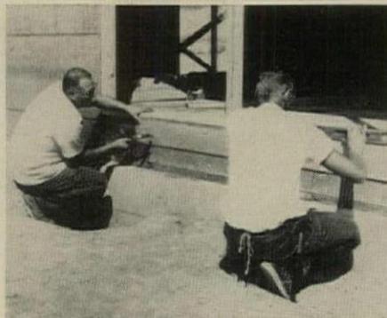
**BOARD IS NAILED** along base line as a straightedge on which the awning section can be rested before it is nailed in place.
