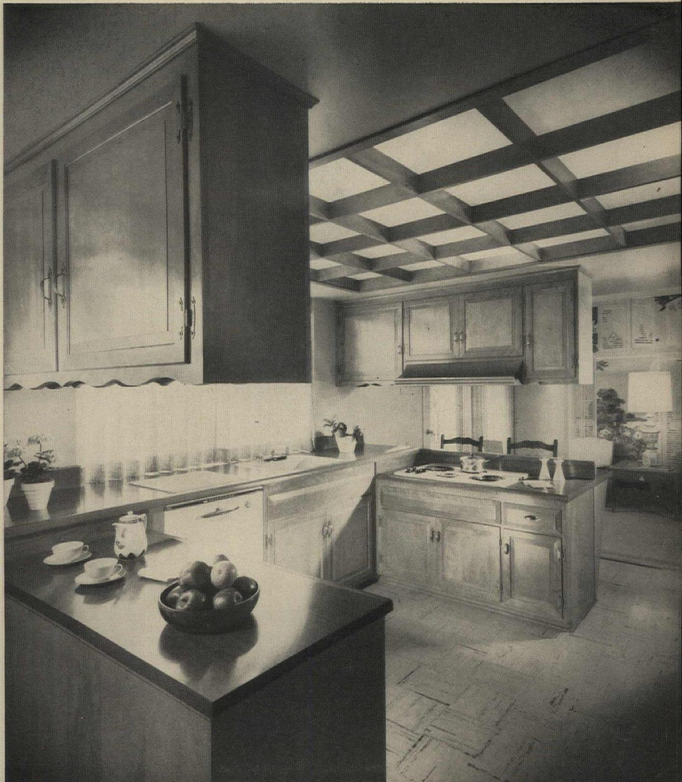
**U-SHAPED KITCHEN** has luminous ceiling ( $\frac{1}{8}$ " fiberglass in stained birch framing) designed by builder and built at site. Cabinets are by McConnell Cabinet Co.
