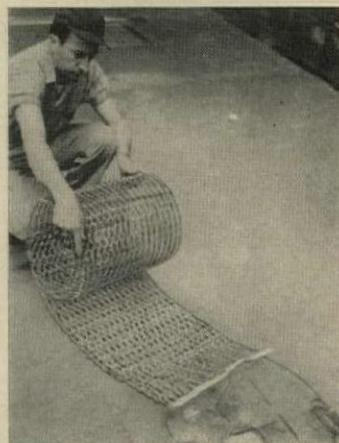
**Chromalox snow melter** for driveways is laid down as a track-wide mesh of wire. The wire mesh is interwoven with electric heating cable, is laid on a concrete base, then covered with the concrete finish coat. Job of hand-tying cable to mesh is cut. Webs are 18" wide, 6' (380 w) or 10' (630 w) long, have 10' cold leads, operate on 240 v.
