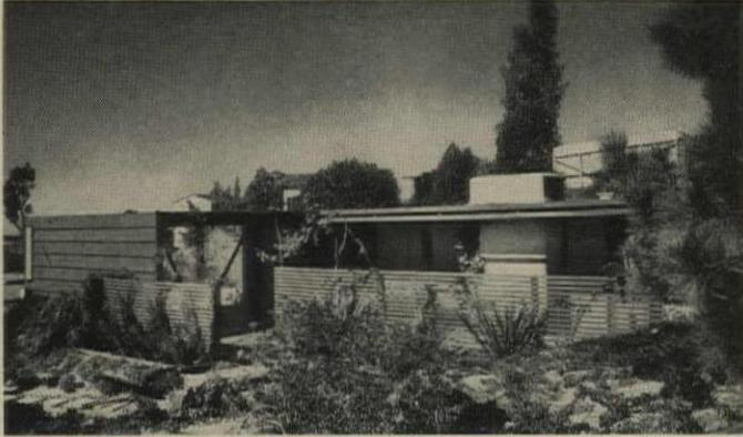
**CARPORT WALL AND PATIO FENCE** screen glass wall of living room from the street. Roof of house is dead-flat to simplify framing.
