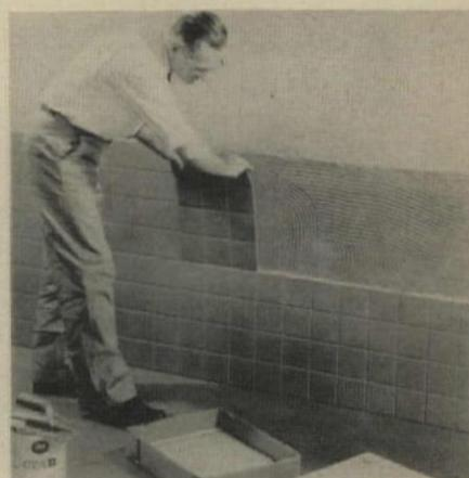
**Tile on sheets** goes up 12 at a time. New American Olean Master-Set tiles have a paper-thin backing that exposes 75% of the bonding area, yet holds tiles firmly enough to assure straight grout lines. Tile may be set with any accepted method; sheets need no soaking before being applied. Master-Set Tile comes in all standard glazed-tile sizes, in regular and crystalline glazes, and in some scored tile designs.
