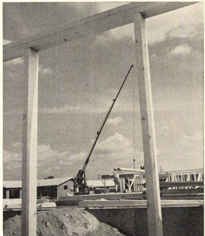
POWER CRANE ("Sky Hook"), mounted on a tractor, lets Medema Builders, Oak Forest, Ill., hoist lumber by horsepower instead of manpower.
