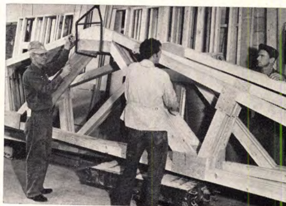
ROOF TRUSSES are standard with builders in many areas. Nail-glued truss shown here is one of several types used.
