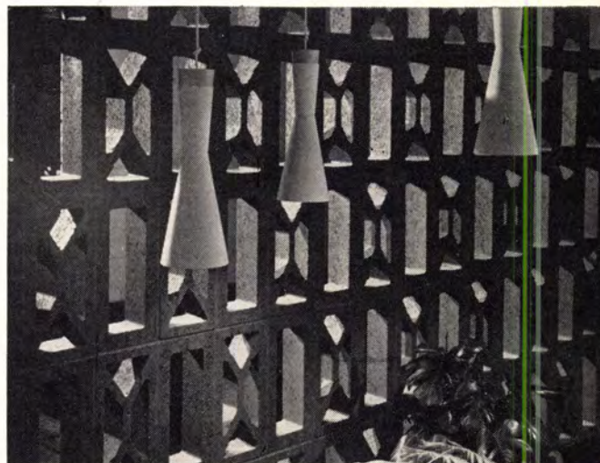
A screen of grille block for either a room divider inside the home or a wall for a patio. Hellmuth, Obata & Kassabaum, St. Louis, designer.
