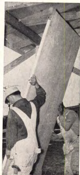
PREFAB PLUMBING WALLS are produced by supply houses like Apsco and by home manufacturers.
