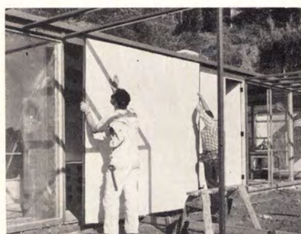
NON-BEARING PANELS being set into place are 1/4" plywood, sandwiching wool insulation.
