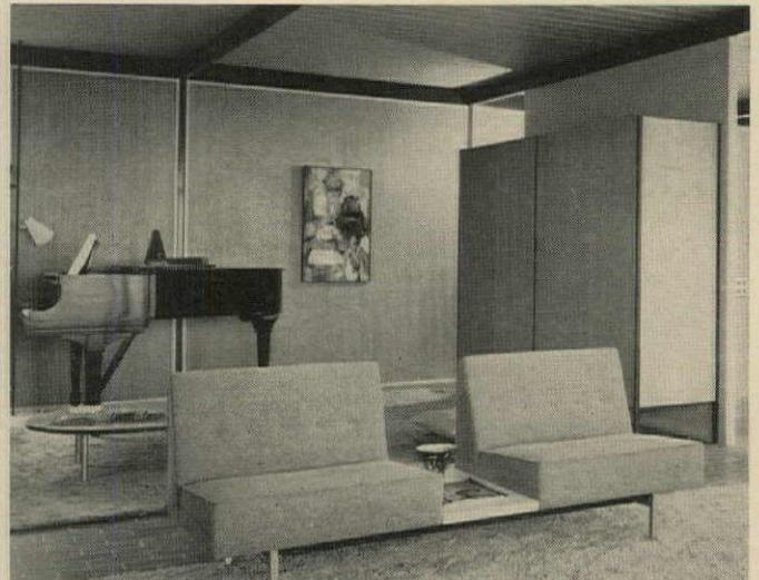
**PANELS 8' WIDE** are formed by butt-joining 4' sheets to fit scale of this large, formal living area. The structural joint is expressed at 8' centers. Designer: Craig Ellwood.
