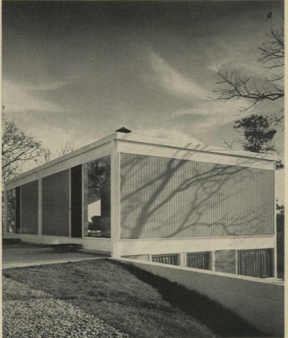
**SMALL PATTERN** of vertical siding that comes from 1-11 plywood is used here in Architect Bruce Abramson's own house.
