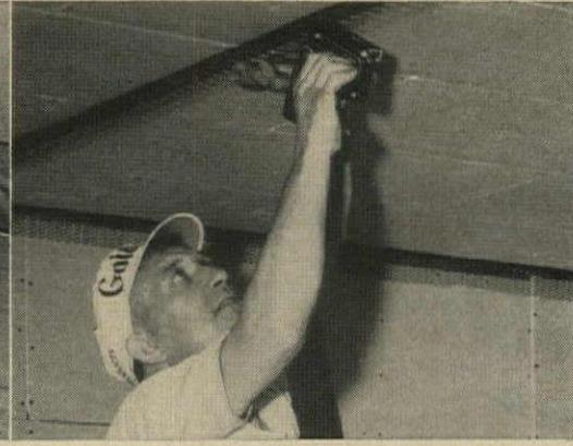
**3** Safe-Edge® Cornerite is stapled to ceiling to hold top of lath panels.
