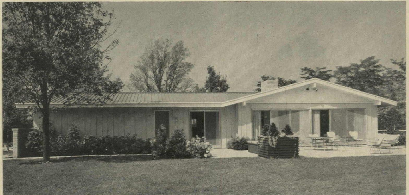
**SMALL PATTERN** of board and batten is pressed into aluminum sheet. The battens have a practical purpose; they give rigidity to the sheets (see H&H, Oct '58).
