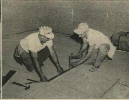
**2** 2" metal floor runner is nailed in position to receive lath panels.
