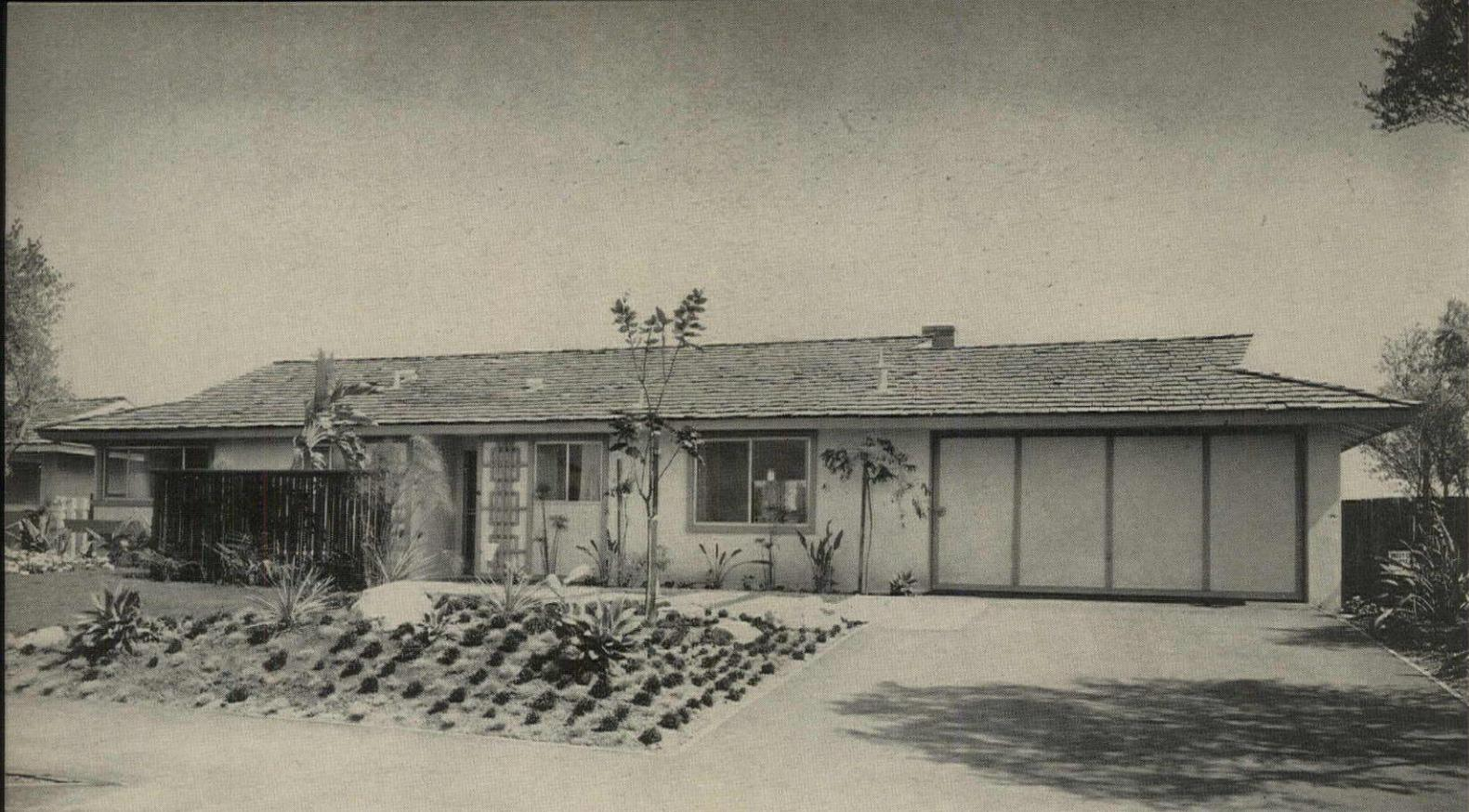
**RANCH** looks larger than its 1,200 sq ft because of attached two-car garage, 4'-wide overhang, and hip roof with ridge extension.
