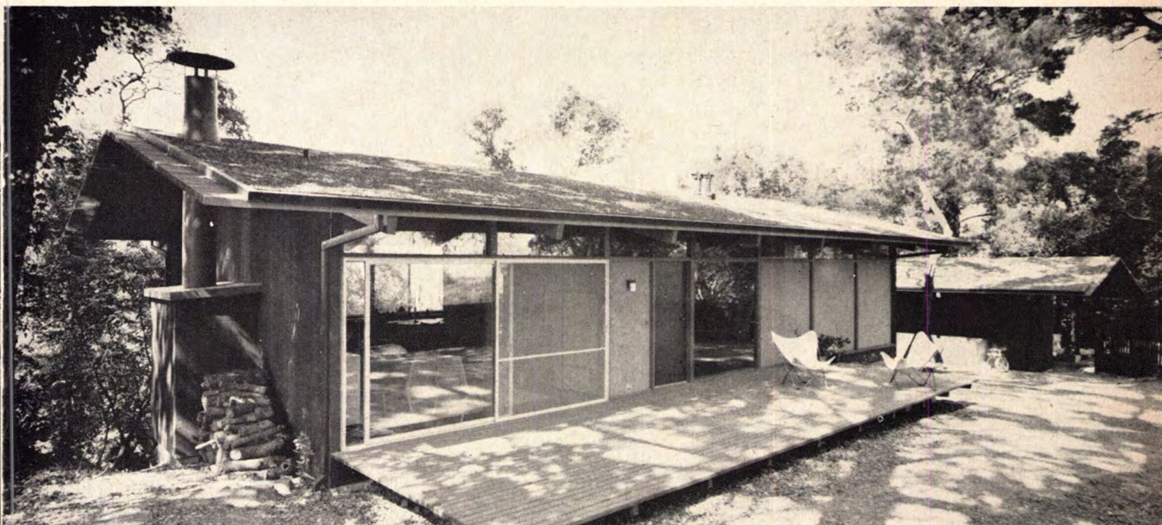
Wide deck extends the main living areas outside the house on the uphill side. Deep overhangs are carried on post & beam framing, 6'8" oc.
