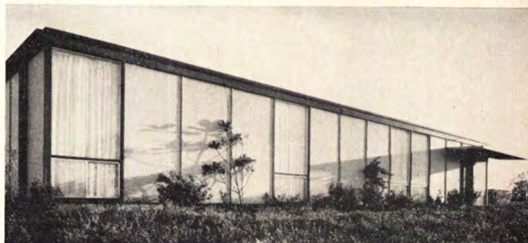
THREE KINDS OF PANELS (wall, window, and door) are interchangeable—all are 4'x8' to use stock sheet materials. Front entry is at far right, bedrooms at left.
