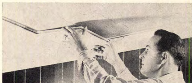
TILE IS PLACED against ceiling; pressure spreads cement evenly.
