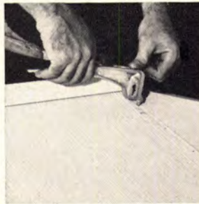
RIVET GUN (single-shot, hand operated) speeds up roofing.
