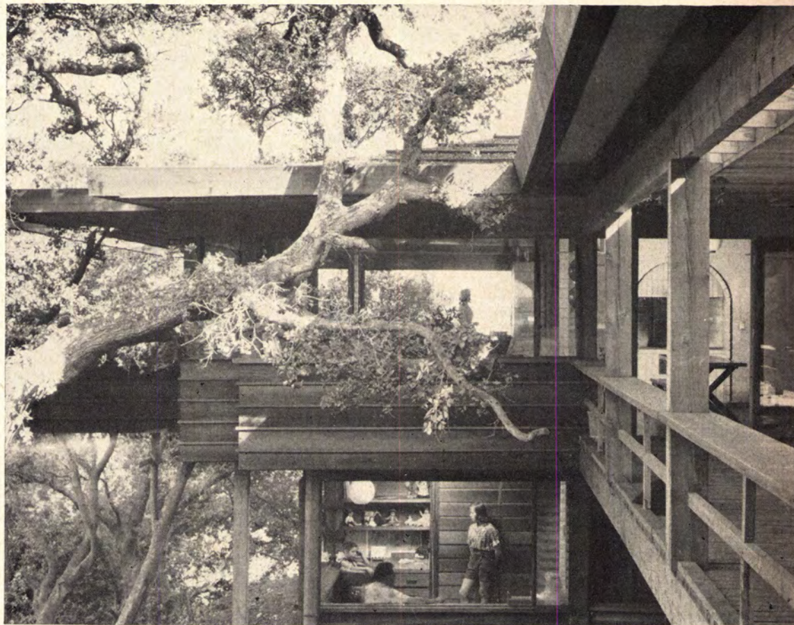
Living room (with its own separate deck) cantilevers out into trees. Roof flattens out into wide overhangs to shelter decks and entry bridge.
