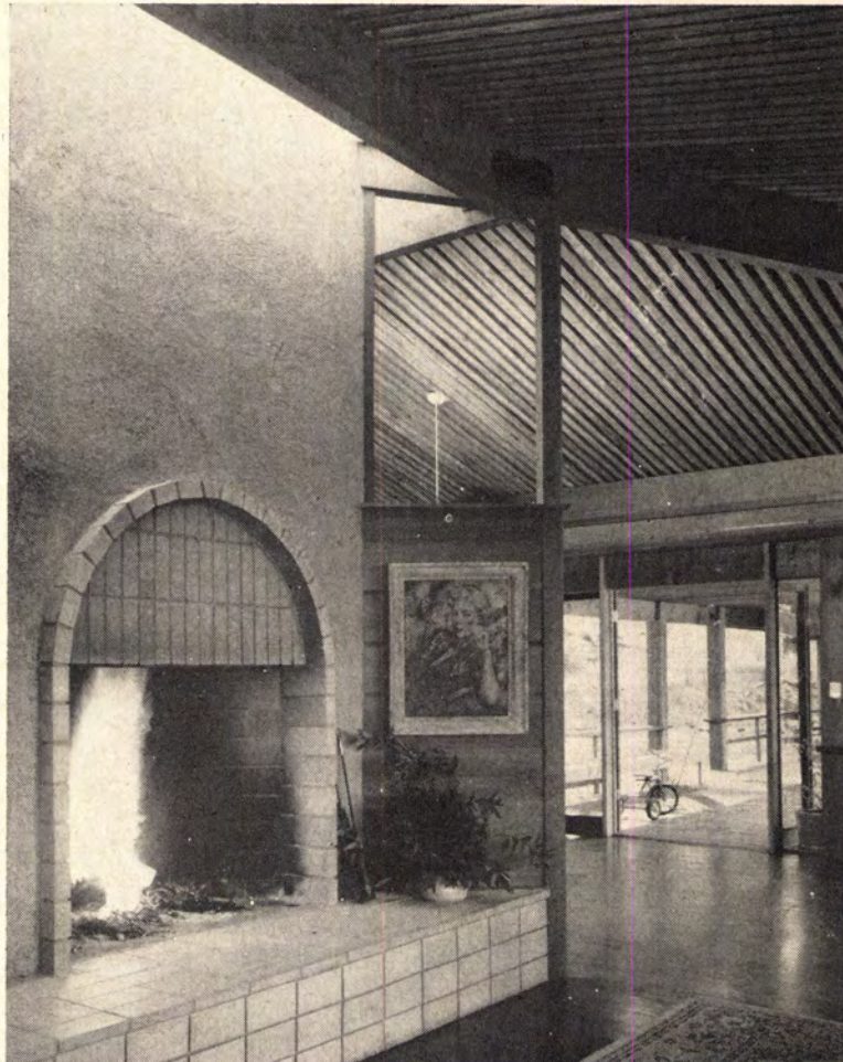
Fireplace core is skylighted on all sides. Exposed ceiling is laminated of alternate 2x3s and 2x4s. Interior partitions are 6'8" high with glass above.
