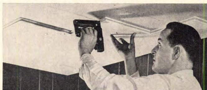
TILE IS TACKED with only four staples; cement supplies bond.
