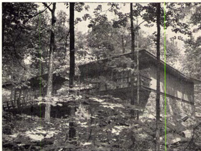
VOLK RESIDENCE, Smoke Rise, N. J. All exterior window walls were constructed of shop-built, prefabricated modular frames, all dimensioned around standard Thermopane sizes. These same panel types, which were fitted into the modular wood framing system, together forming the structural wall and exterior and interior finish, accommodate standard steel sash, blank opaque walls, French doors and regularly hinged doors.
