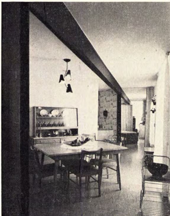
STEEL BEAM , seen here in dining room, runs length of house and is supported by three steel columns 20' oc.
