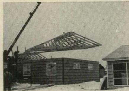
**TRUSSES ARE LIFTED** on angle bar, set on wall panels, and nailed in place.
