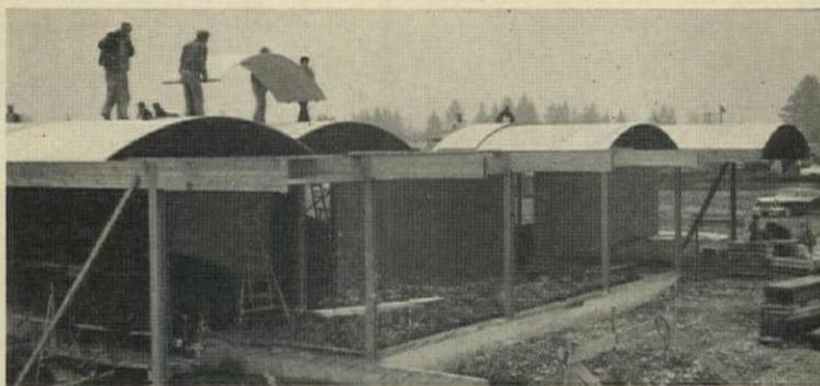
**16** Vaulted roofs like the one on the Redi-Gas building in Parkland, Wash. are being adopted by more and more builders for home construction. Components were four-foot-wide arched stressed skin panels of Exterior fir plywood with paper honeycomb core. Lightweight, easily handled, each spans 16 feet. Component construction helped keep total cost of the building to \$8.10 psf.
