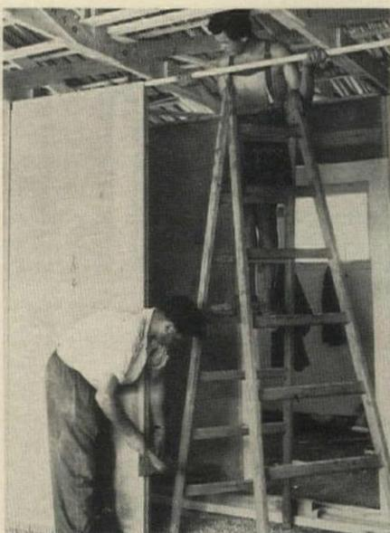
**PARTITION COMPONENTS**, in six varieties, fit into splines between floor slabs and roof trusses. Wiring is distributed through attic.
