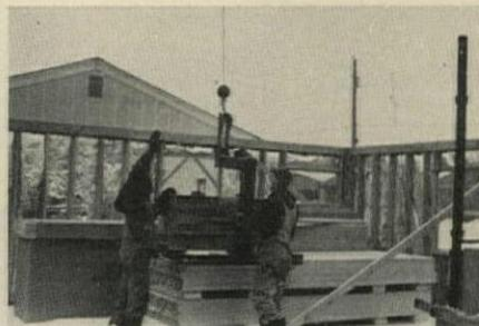
**PALLETIZED LOAD** of sheet materials is deposited exactly where needed inside walls.
