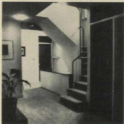
**Add an entrance closet.** The large staircase in this Massachusetts house was closed in so a good-sized hall closet could be built in next to it and near to the entrance. Closing in the stair made a new handrail a necessity so it was made as simple as possible, in keeping with the rest of the modernization. Architect: Frederick Bruck.
