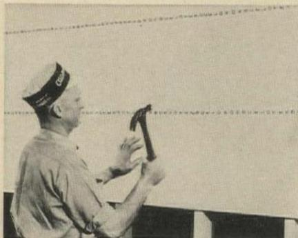
**"Frame locators"** eliminate guesswork in nailing Celotex's Celo-Rok or Fi-Rok gypsum wallboard. Each sheet is printed with small letters spaced 1" apart in lines 16" oc. When drywall is nailed vertically, the lines locate studs; horizontally, letters are the key. Lettering fades when exposed to natural light.
