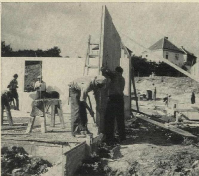
**EXTERIOR WALL COMPONENTS**, shown here during assembly include a blank wall panel, exterior door panel, two small window panels and two windowwall units. All window panels arrive on site ready glazed.
