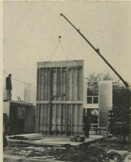
**LIGHTWEIGHT WALL** of NAHB research house has two-story Geon plumbing rig.
