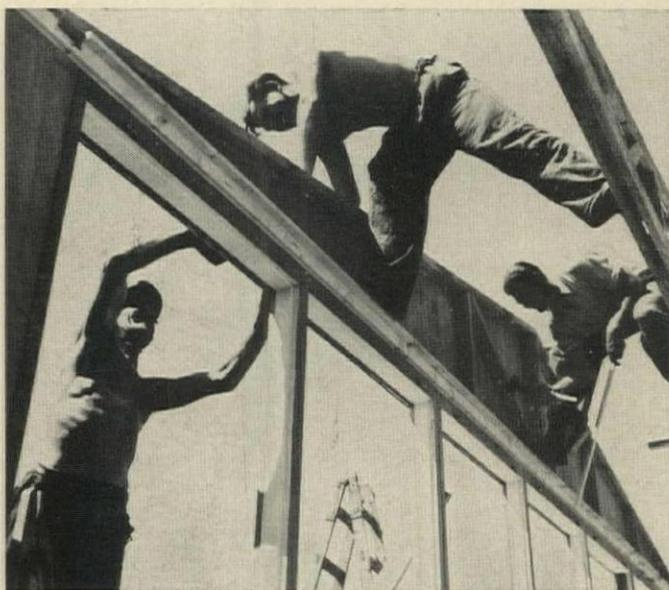
**ROOF TRUSSES** being erected here come in three sizes (7, 8, and 9 meter spans). In the pilot models, trusses were topped either with panels, or with "Fural" aluminum roofing on purlins (see below).
