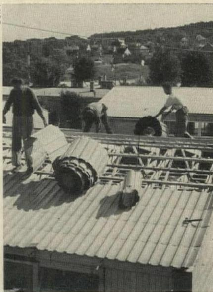
**ALUMINUM ROOF COMPONENT** is a patented Swiss system called "Fural," requires only purlin support, "zippers" together.
