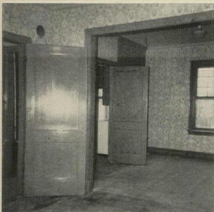
**Add a large living room.** This one in Pennsylvania is big enough to have a dining area at one end (photo, right). To make the room big enough, a nonstructural archway was removed and a door closed up. With redecoration—new wallpaper, repainted trim, and refinished floors—the new living-dining room was complete.
