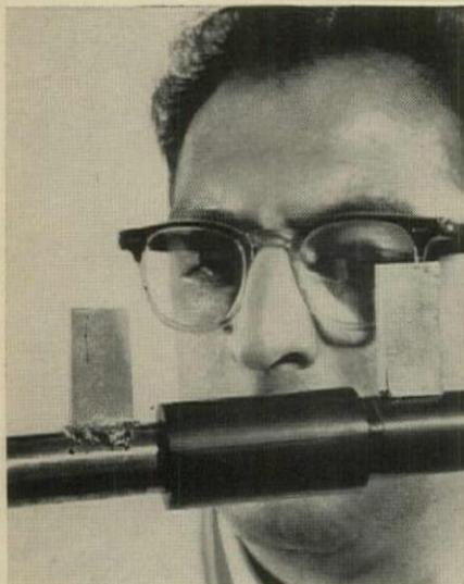
**HEAT TRANSFER** through metal, left, melts test alloy, which stays solid on Geon, right.
