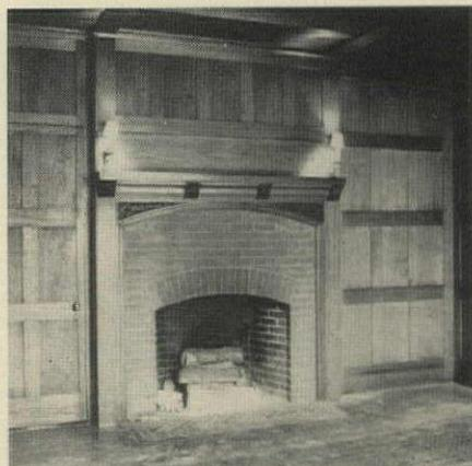
**Add a modern fireplace.** In the case shown here, it was easy; the existing fireplace was left intact and painted to match the walls. A new mantel was added, at a lower height. The surrounding walls were furred, plastered, and then wallpapered in a light colored paper. Architect: Frederick Bruck.
