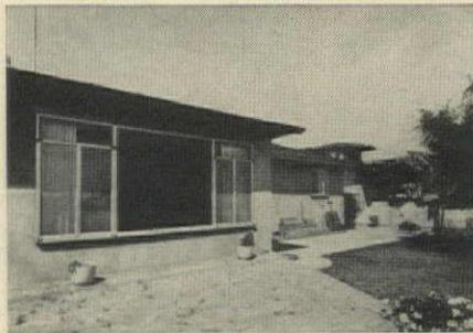
**Add enclosed outdoor living.** In this case, a plastic roof was added, to cover the outdoor living area. New roof line extended the length of the house to remove the old roof line's jagged look and shade the large windows. Brick planter also extends the length of the house to soften the appearance of the stucco finish. New outdoor living room has sliding glass doors and (not in photo), barbecue fireplace.
