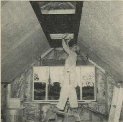
**Add bedrooms in the attic.** The attic shown here was turned into a bedroom and a den-sewing room, with plenty of storage between them. The attic was unfinished, but already insulated. The roof ridge was adopted as a lighting trough; plastic sheets cover the light bulbs and cut the glare. New wider window replaced the existing one. Battens to cover joints of painted plywood sheets give finished room a panelized look. Architect: Walter Widmeyer.
