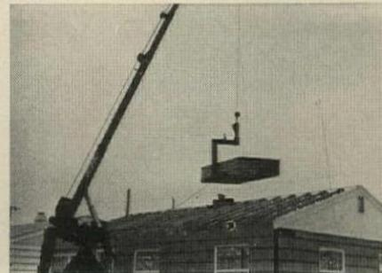
**ROOF SHEATHING**, last cargo unloaded from trailer, is swung onto trusses. /END
