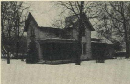
**Add on a garage,** especially when it can be a two-car garage, like this. With the garage set away from the house, the space between is closed in, to become an up-north Florida room. This is part of a modernization program that refinished the entire house, inside and out, in the LIFE Modernized Model House Program. Cost of garage: \$1,838; of the Florida room (with electric heat): \$4,500. Builder: Mt Clemens Construction Co.
