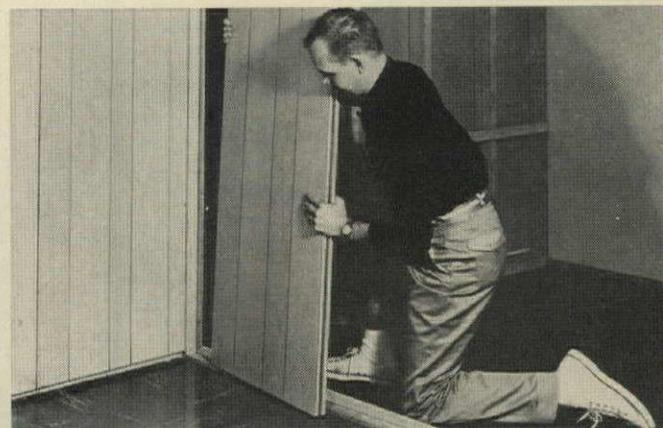
**PARTITIONS** slide in place over floor plate 1/2" thick. Splines and plates tie panels into a wall more rigid than conventional partition.
