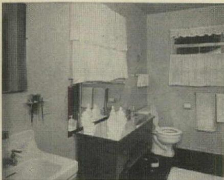
**Add luxury to an existing bath.** This bath, in a North Hollywood apartment, was turned into a glamorous room by some very simple changes. A new lavatory was installed in a vanity counter. The counter, faced with white unglazed ceramic tile, has a mirror its full length and storage cabinets below. The lighting soffit over the counter runs the length of the room. Architect: Lucille Raport.
