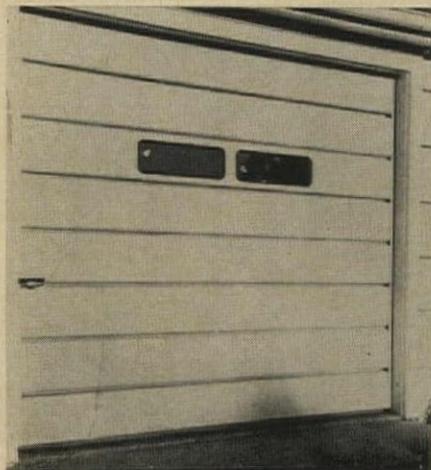
**Primed steel door** is newest Berry Suburban line model. Preassembled hardware cuts installation time to 20 minutes. One paint coat finishes. Horizontal V grooves add strength without weight, are designed to reject fingers when opening or closing. Five-year guarantee.
