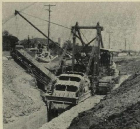
**LARGE TRENCHER**, wheel type, digs sewer main.
