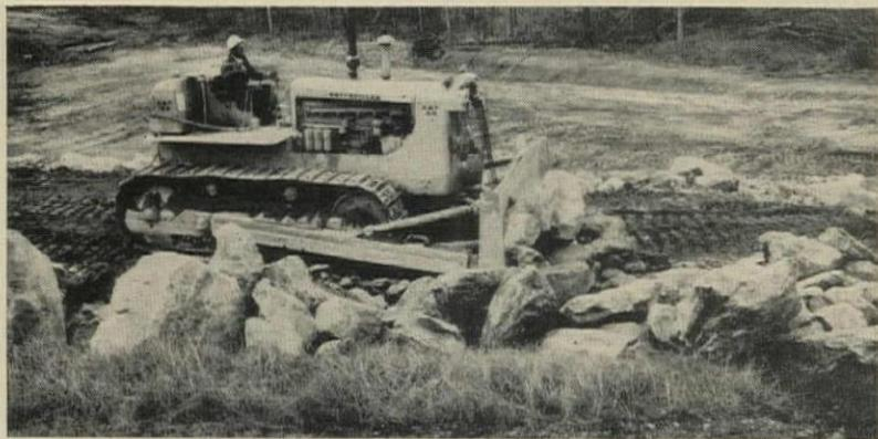
**DOZER** clears ripped rock. Ripper dislodged boulders or broke them in big chunks.
