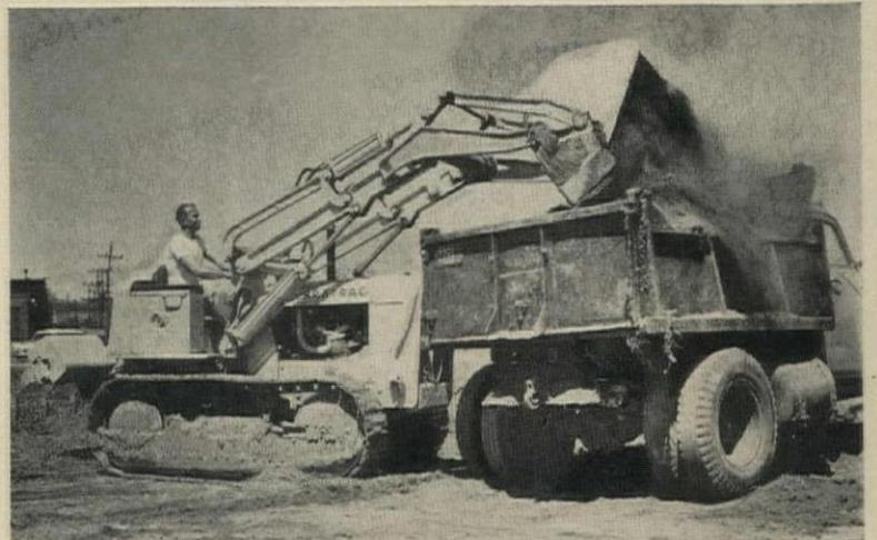
**TRACTOR SHOVEL** loads dirt into dump truck after digging and piling it.
