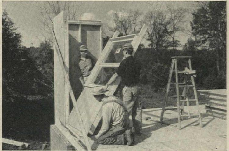
Here you see **Andersen Strutwall**—a complete structural wall component with window unit—being tipped into place at the Fiser Development. Strutwall cuts window installation time from 30 to 50%.
