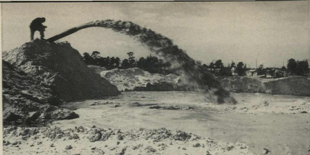
**DREDGE TAILPIPE** spews fill into dike-enclosed settling area. When fill is high enough, pipe is moved.
