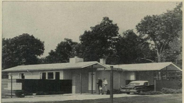
**COMPONENT-BUILT HOUSE** has vertical aluminum siding, interlocking aluminum shingles. Front roof is 42' wide; 57' rear roof extends to cover carport.
