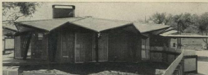
**FINISHED HOUSE** has nonloadbearing exterior walls that can be set at any position because buttresses (photo at left) carry all loads.
