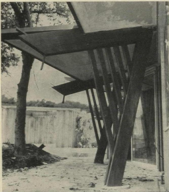
**BUTTRESS**—paired 2x8s braced by five 3x3 struts—supports 3x6 roof framing. Outriggers on ends of 3x6s are 1x12 fascia boards.
