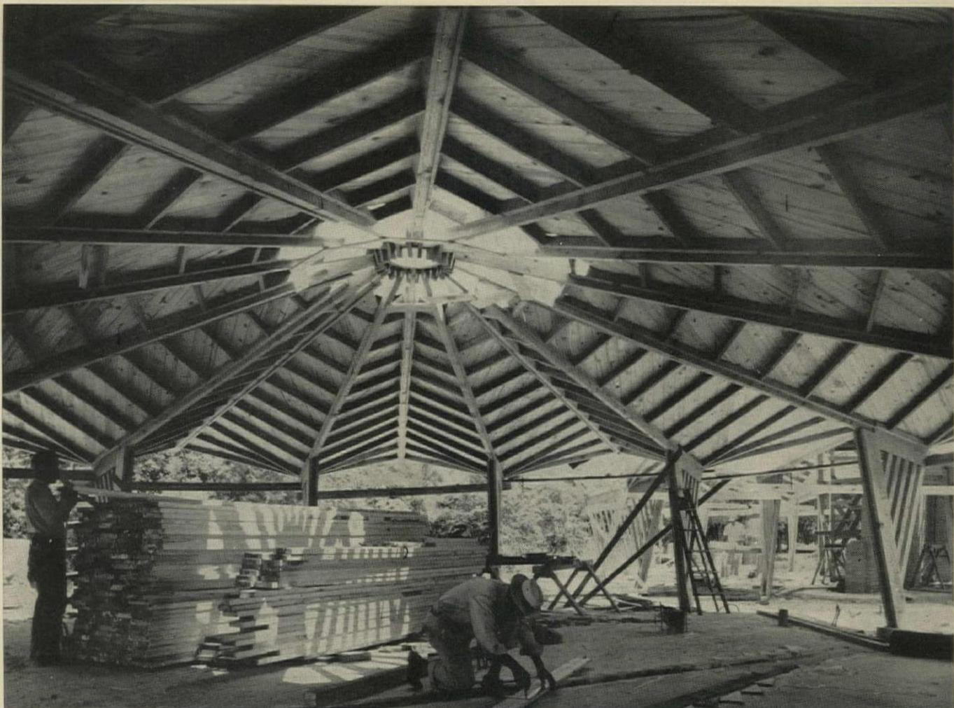
**CIRCULAR ROOF** is made up of 12 triangular folded plates fastened to 12 joists (3x6s). Plates and joists converge at center steel compression
