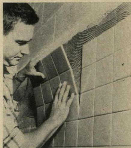
**Stylonet 12-set** is a 3x4-tile sheet of 4 1/4" ceramic wall tile mounted on a paper-mesh backing that allows 70% contact between tile and wall. Sheets will not buckle, handle easily. Mesh is quickly cut with a trowel, is pliable enough to adapt to wall surface.
