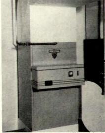
ELECTRONIC AIR FILTER. "We think this unit has tremendous appeal for the housewife. It's almost an automatic house cleaner and it has a health appeal too. It is set in the return-air duct for the upperlevel system. In-place cost of the Trion unit we used: \$375."
