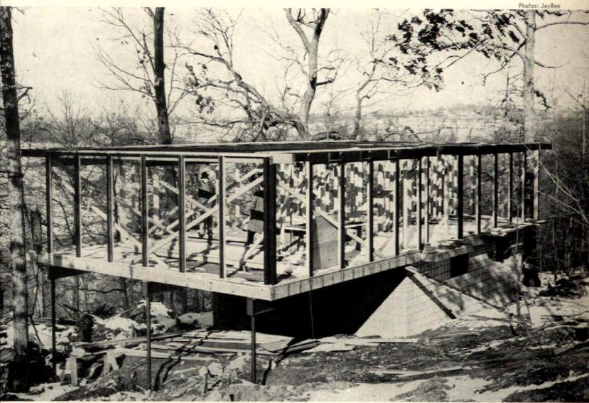
READY FOR PANELS, post-and-beam framing rests on conventional floor supported by I-beams over carport and concrete-block lower level.
