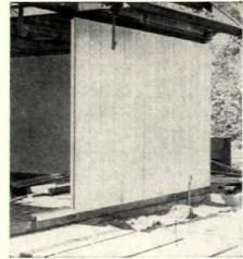
PANEL EXTERIOR has batten at center (see detail). Corner piece is fastened with clips.
