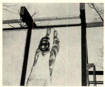
5 Finishing takes two steps: first, elastomer tape is stuck to edge of panel face, then outer stops lock panel in place. Twenty-four panels were used in exterior wall, 60 in the roof.
