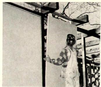
Enclosing house is fast. Wall panel, with aluminum skin out is pressed against caulking bead on inner stop. If panels were used for load-bearing they could support loads of 1,200lb/ft.
