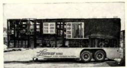
HOUSE PACKAGE arrived at site on standard prefab trailer. Windows were already in place in frame, coiled electrical wiring ready for hookup.
