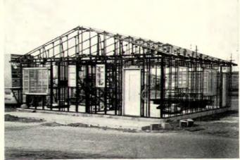
**SECOND STEP** was to set up steel roof trusses, diagonally brace them together and tie them down to wall framing. Then interior partitions went up, tollowed by rough-in wiring and plumbing.
