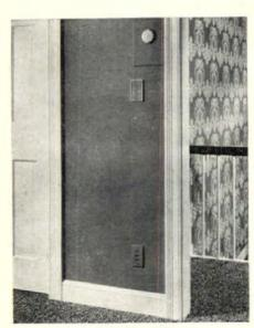
TRIPLE WALL PLUGS. "The top receptacle of each of these Bryant units is connected to the Bryant Fashion Plate wall switch in each room, so several lamps on different outlets can be put on the switch. We put these units in every room but the kitchen.
