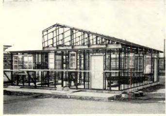
THIRD STEP was to close gable ends with 1'-wide porcelain enameled steel panels. All-steel Lustron houses are so strong that trucks have run into them and been demolished without seriously damaging house.
