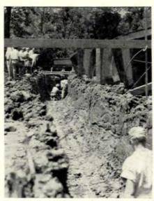
**TRENCH** is rounded to form underside of pipe. Aluminum interior forms are at right.
