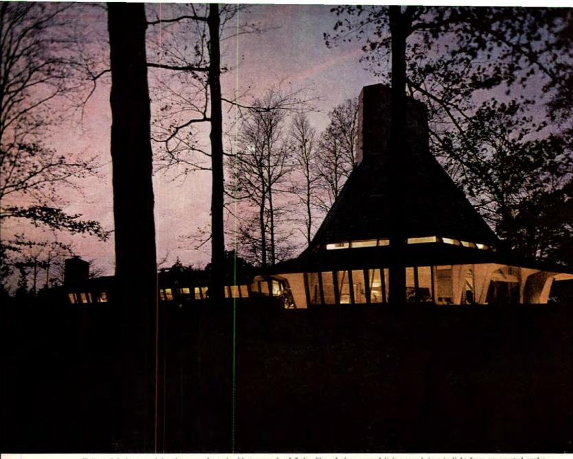
Tall roof is hexagonal in plan, was framed with trusswork of 2x4s. Slot of glass around living area brings in light from unexpected angles.
