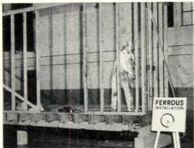
END OF A DAY'S WORK—Copper tube system 100% complete and tested in 7½ hours...less time than installation of only the ferrous drainage, waste and vent lines.
