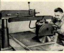
adial saw line. New unit has extra-wide ip capacity (36"), will cross-cut 24", cut 3%" deep, cut 1½" wide dado with a 10" lead. Power options are 2-hp, 3-hp, or 5-lp. Standard Delta features include double werarm, individual miter stops, enclosed rackways, up-front controls. \$645 up.
