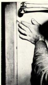
Wallboard cleats eliminate non-structural studs or nailing strips at interior corners of walls and ceilings. Cleat is nailed to framing member (left); drywall is put in place and fastened to intermediate studs; nails are driven through drywall into cleat (right) where a slot pulls them tight, anchors them in place. Claimed advantages: cuts installation time up to 75%; stronger than conventional nailing; cuts nail popping; allows for house settling. FHA accepted. Price: 5¢ each.
