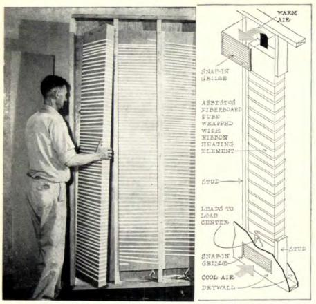
HEATERS are made of radiant ribbon wound on fiberboard tube; drawing shows air flow.
