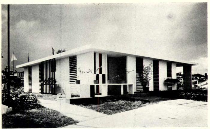
FLAT-ROOFED MODEL has 975 sq ft of living space plus carport and rear terrace. Floor, roof, and all walls are concrete.
