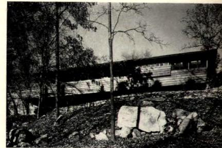
South side faces the view. Here Wright used large expanses of glass set in a wood framework. Horizontal band of siding is balcony parapet,
