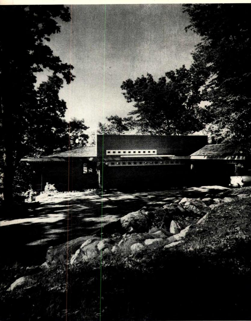
Approach side of the house faces north, has almost no openings. The kitchen is lit through a frieze of glazed perforated blocks.
