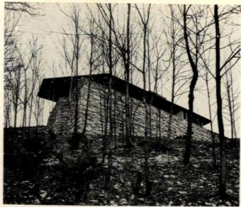
Stone ramparts surround the south and west terraces outside the living area. Perforated roof overhangs bring sunlight indoors without destroying the horizontal sweep of the roof planes all around the house.
