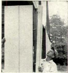
EXTERIOR JOINTS are finished with batten strip held in place by clips over caulked seam.
