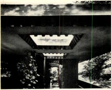
Balcony is sheltered under deep roof overhangs. These overhangs are perforated with square openings that let light into the living area. Planting boxes built into the balcony make for easy transition between indoors and outdoors.
