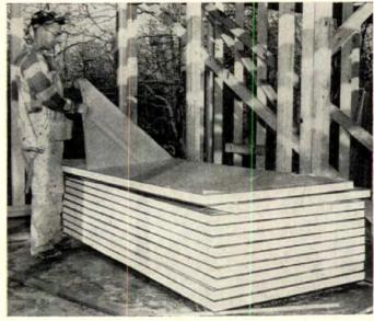
Prefinished panels have paper protection. In background stude partitions with diagonal bracing give racking resistance. Panels can't do this as they are used simply as curtain walls.
