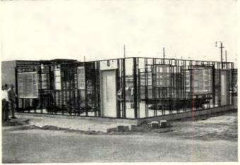
FIRST STEP was to get exterior wall frame up and fastened down to anchor bolts set in block perimeter of concrete floor slab. Note diagonal bracing between doubled steel studs, doors preset in frame.
