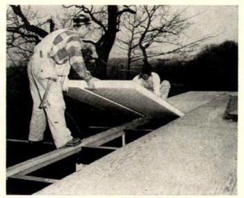
Roof panels at roof edge are dadoed with power saw and hammer (for hacking foam) to cut heat transfer in skin and fit over 2x4 plate that positions roof beams. Panels can span 8'.
