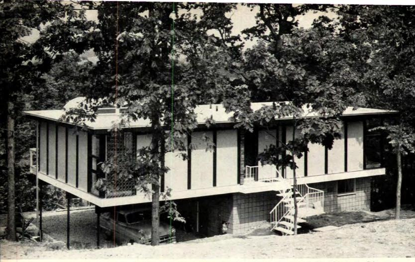
POST-AND-BEAM FRAMING gives strong panelized look. Panels are set between posts with wood stops. Three barrel skylight, left rear, opens living room.
