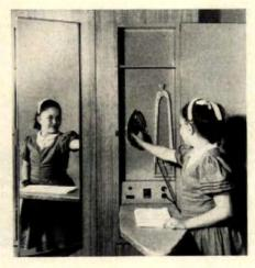
Laundry built-in is a mirror-door cabinet that holds ironing board, sleeve board, timed electric outlet, extra con-venience outlet. Control panel also has pilot light and reset circuit breaker. Steel cabinet is fireproof; silicone-aluminum pads are heat-resistant. Early production models list at \$109.50.
