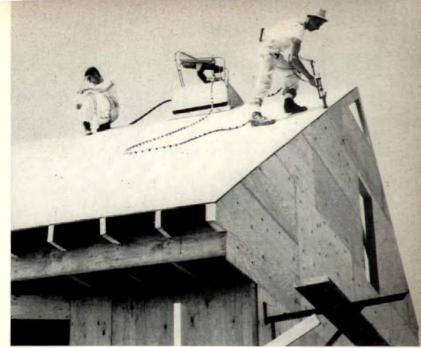
SHEATHING ROOF, operator walks down slope from ridge to gutter. He covers over a third of the roof without having to move the separator.
