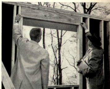
Materials saved: At Ryan's Williamsburg Village development, engineering team measures window framing material. Strutwall eliminated cutting, inventory and eventual fitting of 47 cripples of 14 different lengths, jack studs, sill plates, blocking and headers.
