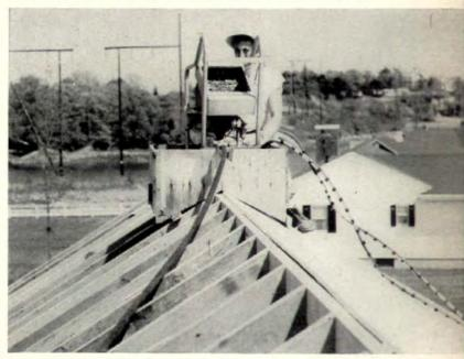
NAIL SEPARATOR rides the ridge in a plywood box cut to match the slope. Separator must be kept level so nails will feed to hose.
