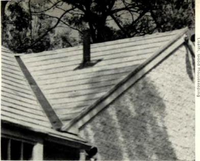
square vs \$22 for a conventional roof. But it goes up much faster, because one man can carry a whole square at a time up to the roof, and because there is only one nail per shingle.
