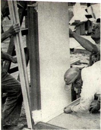
PANEL ERECTION starts at corner. Bottom edge of panel (see detail, below) clips to sill channel. Back of baseboard raceway is being bolted on.
