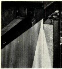
PANEL TOP engages clips welded to header beam. Inside face has stiffening corrugations.
