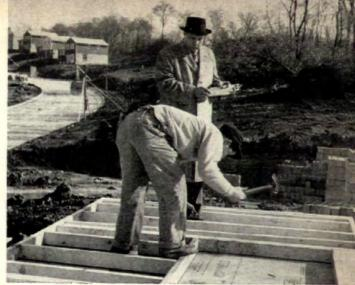
Smaller crews busy all the time! This is what Ryan's time studies showed Strutwall could do. Saved waiting for materials, too. To install Strutwall, cut two load-bearing side struts to fit header construction...nail to adjacent studs.
