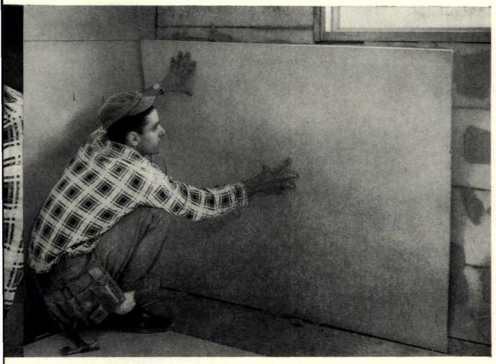
Workman fitting a section of dry wallboard in place against the Styrofoam insulation. Wallboard is then braced for 24 hours until cement dries.
