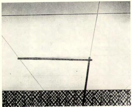
acoustical ceiling tile. "The new thing about this Owens-Corning Fiberglas product is that it comes in big pieces. We used both the new 2'x2' size (above), which is held in place by a metal spline
