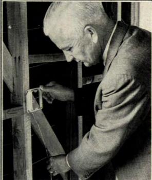
Telephone man Mason Layton checks concealed telephone wiring and position for outlet in a Gardiner "Mission Ranch" home at Fremont, Calif.
