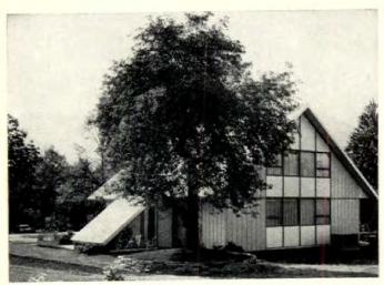
**SUN ROOF** slopes to ground at rear of house and opens mechanically to expose second floor sun deck and to light master bath.
