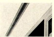
Maintenance-free soffit is made from perforated asbestos cement. Vent holes allow adequate air flow, will not admit insects. Gold Bond perforated soffit material comes in 2'x4' sheets with integral white finish. Panels are autoclaved, will not rot, burn, sag, buckle. No painting is needed except to change color.
