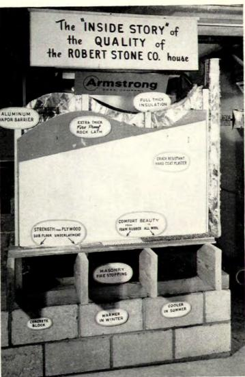
INTERIOR SIDE of the wall shows new "Hardcote" plaster finish. Note the "Eastern brace" construction required by the local code.
