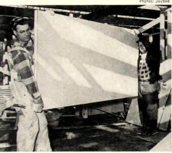
Light-weight, 4'x8' panels are easily handled by two men, so a crew of three can enclose house in two days. Panels can be load-bearing, but in this house, framing takes all loads.
