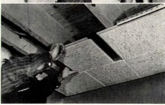
Ceiling tile clip-strip, nailed or stapled directly to ceiling joists, eliminates furring strips for wood fiber tile. Tile slides easily into channel, which is hidden by tile's t&g edges. No other fastening is needed. Installer works across room, row by row, puts up full ceiling in one pass. Clip-strip gives perfect alignment, cuts headroom less than 1" (vs 1½" or more with furring). Clip-strip comes in 4' lengths, 25 to a package.
