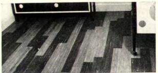
STRIP FLOORING. "By laying the vinyl strips in different directions, we can make a room seem longer or wider. We used Kentile."
