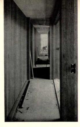
INTERIOR PANELING was left unfinished so that nothing would detract from the decorative grain patterns and subtle color tones of the saw-textured redwood. Exterior siding was treated with a clear water-repellent.
