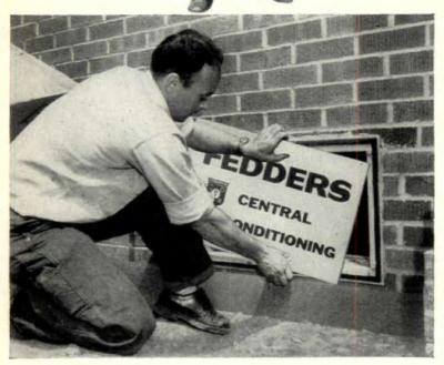
"This wall frame was set by the general contractor when he put in the concrete block foundation. It saves the cost and expense of setting forms and pouring a concrete slab. The rear cover plate seals the opening...lets buyers who don't want air conditioning right away add it inexpensively at a later date. Frees builders from FHA income restrictions, yet lets them promote whole-house air conditioning."
