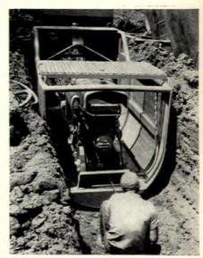
engine-powered winch reels in anchored cable to pull machine along the trench.
