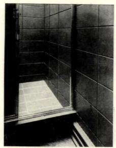
GLAZED-FINISH BLOCK. "In the lower level bath, we made the foundation wall do double duty by using a concrete block with a glazed finish on one side. The block has a plastic finish, called Spectra-Glaze, which is good looking and very easy to keep clean. The 12" blocks cost 80¢ each."
