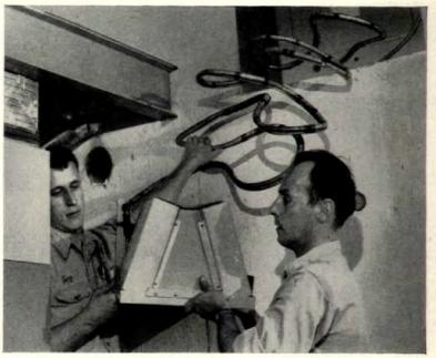
4 "My partner then carries the 'A' coil while I unfold as much of the flexible hermetic line as required. It permits 18 feet of travel, so there's no home too big. The flexible line is armored so there's no danger of kinking. This takes only minutes...instead of hours we used to spend bending and brazing hermetic lines and charging the system with refrigerant."
