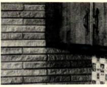
**Decorative masonry** that is also sound absorbent (noise reduction about 30%) and insulating (K = 1.7 to 2) is called Z-brick. Bricks  $12"x1\frac{1}{2}"x\%"$  are made of cement, pigments, and vermiculite. They can be glued to any flat flakeproof wall with a special waterproof adhesive. Bricks come red, tan, or green, 60 to a carton.
