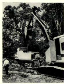
**MACHINE** is lowered by crane at head of trench to start casting pipe.
