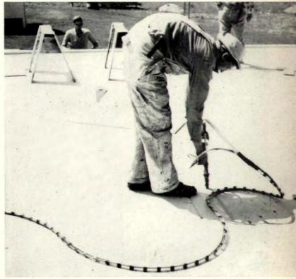
PLYWOOD SUBFLOOR is nailed in less than an hour as worker walks the chalkline. Walls are framed and sheathed flat, tilted up.
