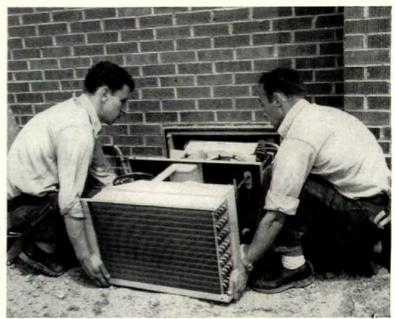
2"The entire FlexHermetic Air Conditioner—furnace-top 'A' coil ... outdoor compressor section... and interconnecting hermetic line, all factory charged and sealed—is slid through the wall frame just as it comes from the shipping carton. Then it's simply bolted onto the steel wall frame, which has a built-in rubber gasket to assure a good seal."
