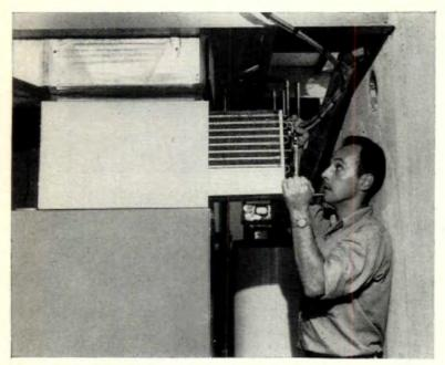
The 'A' coil slides right into the furnace-top plenum—and the whole hermetic job is done. You can see why any heating contractor can do the entire job without hiring refrigeration sub-contractors or high salaried mechanics. The furnace?—it's Fedders' FlexAire with a multi-speed blower that automatically delivers the right cfm needed for heating and for cooling."
