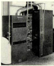
TWO-FURNACE ZONING. "We use one furnace to heat each level. We found almost no difference in cost-the two units cost a little more than one big one, but we saved on ductwork. And there are big advantages for the homeowner:
