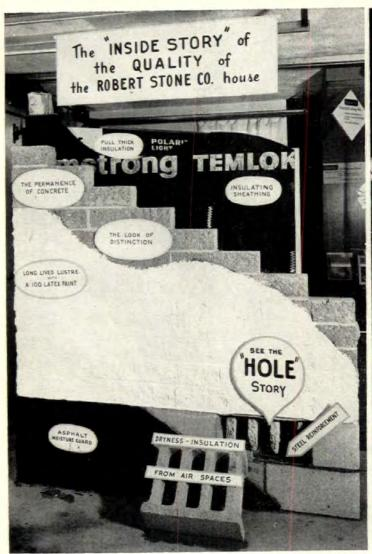
**EXTERIOR SIDE** of the wall is cut away to show veneer construction with split concrete block and features of the foundation wall.
