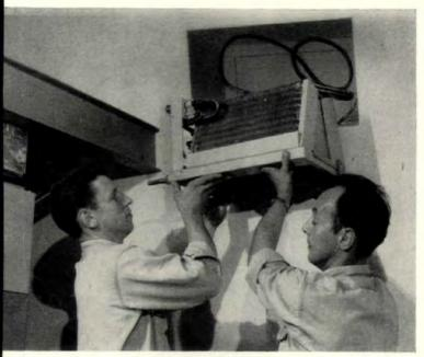
3 "The rest of this remote air conditioning installation is done indoors. In the basement, we remove the shipping braces in minutes to free the 'A' coil and the flexible hermetic line. In slab homes, this would be done in a utility room with the outdoor section and wall frame out of the way under the eaves—goes into any kind of wall—brick...studding...what have you."
