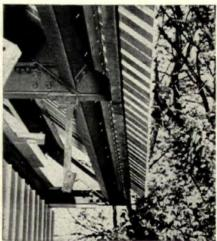
EAVE LINE shows how decking is fastened to Z-beams. Foreground hanger supports soffit.
