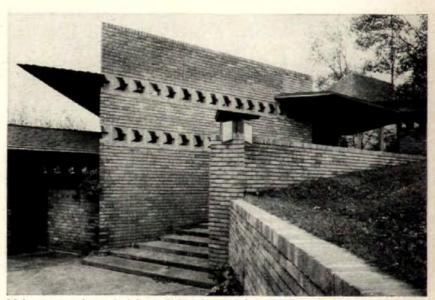
Main entrance is reached by a flight of steps of gentle proportions. The perforated bricks were specially cast with fixed, translucent glass embedded in their centers. Lantern on pedestal was designed by Wright.
