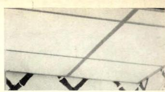
Panels' we chose give a soft light, and let us use a higher ceiling without the fixtures showing through. The panels sit in an aluminum T-strip. We find it takes less than a day for two men to do the ceilings in the three baths, the laundry, and the snack bar. The panels cost 85¢ a sq ft plus installation." (Pattern at bottom of photo is wallpaper.)
