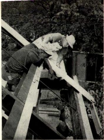
ROOF DECKING starts with workmen aligning lower edge of panel at exact eave line (determined by man with level). Screws fasten decking to Z-beam.
