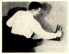
Wallboard adhesive from 3M is designed for installing hardboard, wallboard, and similar materials to existing plaster, drywall, wood, concrete, or other sound smooth surfaces. Rubber-base mastic gives high strength, is fast drying, water resistant. Adhesive may be floated or buttered, fills irregularities between surfaces.
