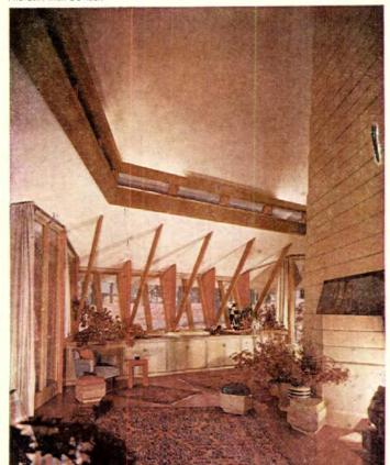
The tall, tapered roof over the living area of this house was one of Frank Lloyd Wright's favorite devices—especially when it could be contrasted with a low-slung roof over an adjoining bedroom wing. He called this tent-like roof his "pine tree type," and this example is the last one he built.
