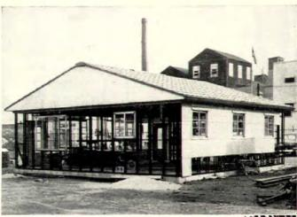
FOURTH STEP was to place big porcelain enameled steel roof shingles right on roof trusses. Ridge cap and gutters finished roof. Exterior wall panels, 2' square, were clipped to frame to complete close-in.
