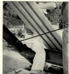
DECK STRENGTH comes from deep longitudinal corrugations. Deck easily spans 12'.
