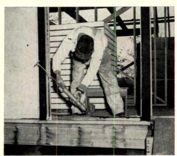
Inner stops (drawing opposite) are set, then bead around opening is laid with caulking gun. Sill flashing fits into kerf in bottom edge of panel's foam core. Posts are 4' oc.
