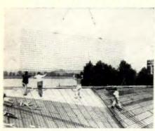
The easiest way to reinforce concrete slabs, apartment house floors or roof decks, roads, or retaining walls is to use a few sheets of welded wire mesh (photo, above). Reasons: 1) the cold drawn wire is stronger per sq in. than
