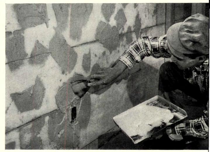
After the Styrofoam is cemented directly to the SCR brick exterior wall with mortar, drywall cement is applied in gobs to the surface of the Styrofoam.
