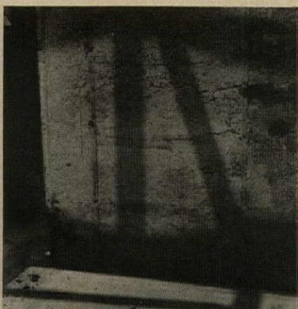
**CONCRETE SURFACE** has rough texture that provides a "tooth" for plastering.
