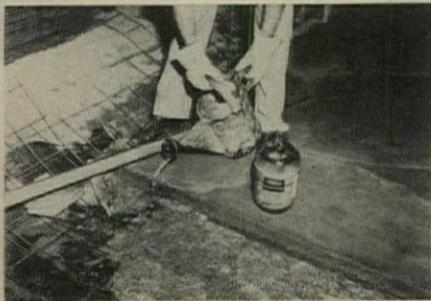
**TERMIBAR LIQUID** is poured into soil areas that are not covered by vapor barrier.
