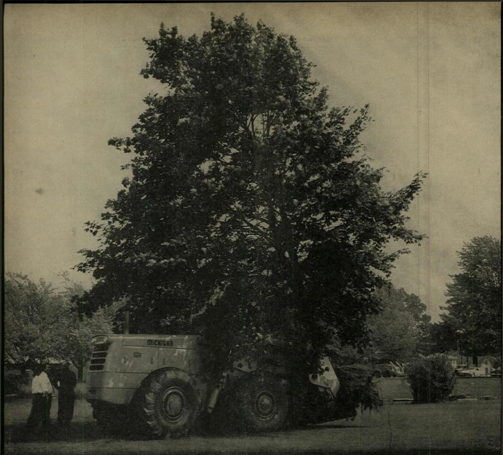
**TREE BEING TRANSPLANTED** was dug up, moved 150 yards, and replanted in 58 minutes by loader with special tree-moving attachment.
