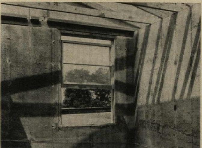
**PREGLAZED WINDOW** was set in form before walls were poured, giving a tight fit. Walls can be poured smooth, painted rather than plastered.
