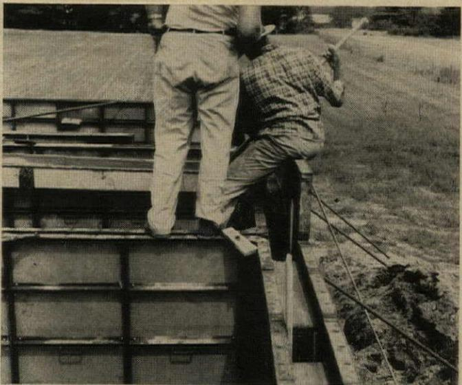
**CONCRETE FLOWS READILY** around prehung windows and doors set in forms (foreground). Diagonal rods are temporary form braces.
