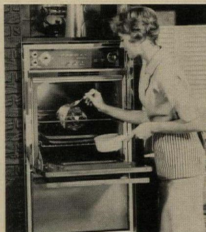
**Preway** Gold Star oven has automatic clock control, low temperature (140F) oven, built-in rotisserie, large broiler. Control panel is encased in heat-resistant glass, lighted by concealed tubes, holds thermostat, clock, timer, push-buttons.
