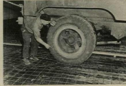
**BEFORE POUR**, vapor barrier and wire mesh will support weight of transit-mix truck.
