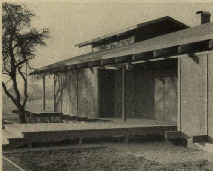
**2** **Panel-and-batten** wall on Eugene, Ore. home was simply built with standard  $\frac{3}{8}$ " Exterior fir plywood nailed to studs with battens at joints, and stained. With weathering, plywood checks and acquires a pleasantly textured surface. One-step wall method meant low cost: \$8.75 psf. For the smoothest siding, use overlaid fir plywood, painted.
