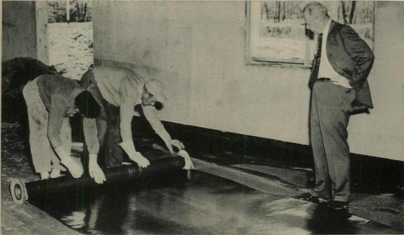
**TERMIBAR SHEET** is unrolled over a gravel base before slab is poured. Sealed 2" or unsealed 6" lap is required.
