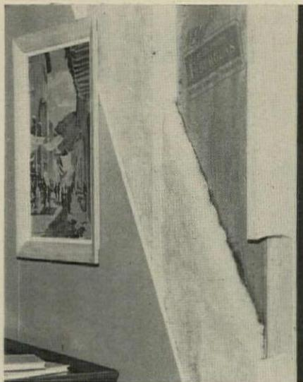
**Sound control blankets** installed back-to-back between saw-split studs are claimed to cut sound transmission 83% over conventional 2x4 framed wall, 20% over 6" block wall. Blankets are stapled only head and foot so they hang limp. An air space between the impervious backing sheets isolates the conductive surfaces. Split stud cuts direct transmission of sound.
