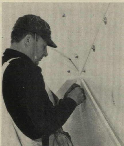
**PANELS ARE BOLTED** through preformed holes by inside and outside workmen.
