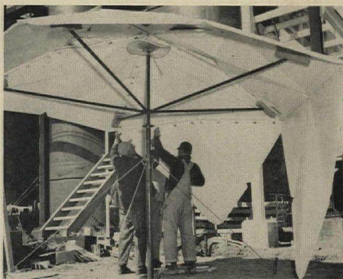
**TELESCOPING MAST** supports dome as panels are bolted to crown. It is raised about 4' for each ring. Dome can be rotated on mast.
