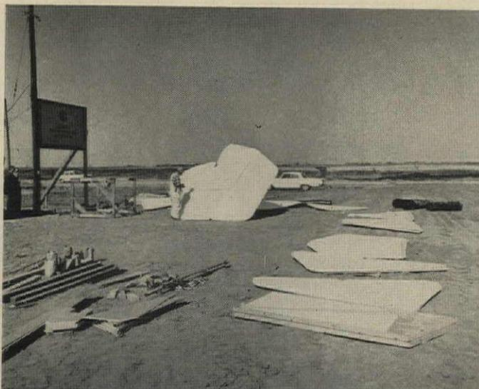
**ERECTION STARTS** with assembly of five crown panels. Panels, wood parts, and mast are laid out at site for ready accessibility.
