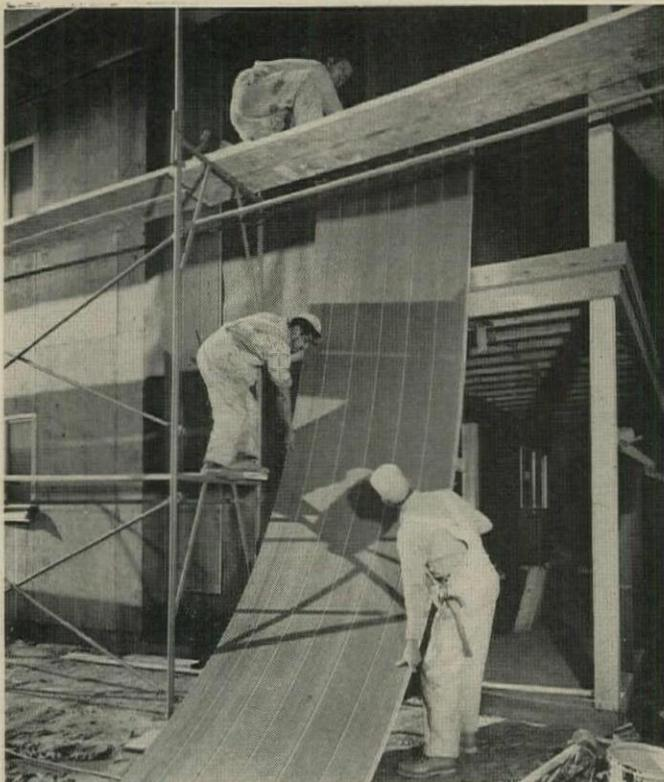
**Big 16' panels** of tempered hardboard speed the siding of two-story structures. The sheets come with smooth or striated surfaces, U-grooved in 4", 8", or random spacing, or factory primed light gray. A modified shiplap edge conceals joints and continues groove pattern; the edge is stair-stepped to provide a built-in guide stop in butting panels.
