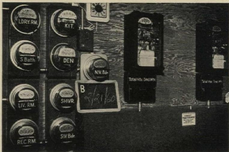
CLUSTER OF METERS records room-by-room heat consumption in two 1,100 sq ft test houses.
