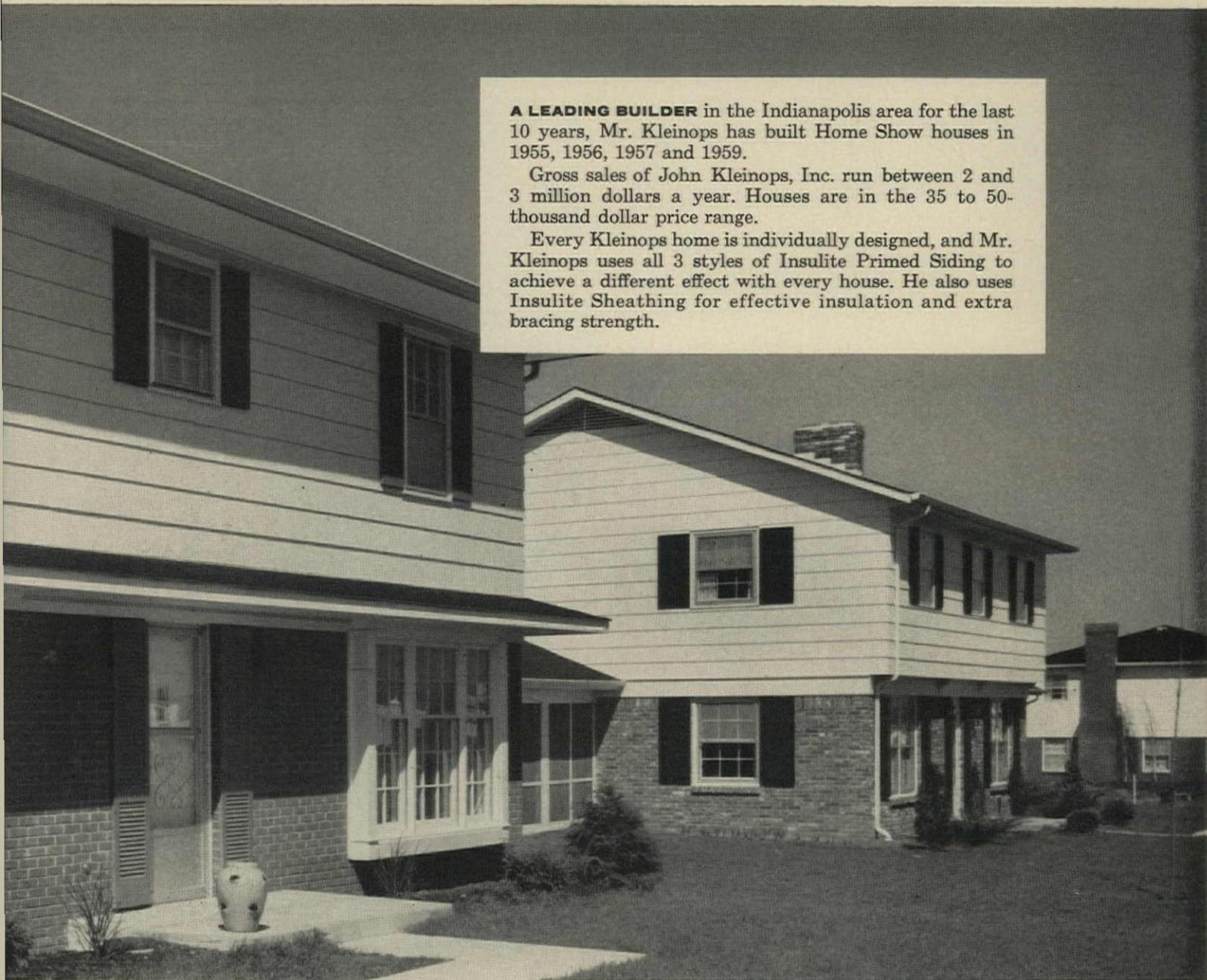
**HORIZONTAL (LAP) SIDING.** This application was made in 1957—and the butt is as tight now as it was 4 years ago. Also seen is the attractive deep-shadow line. Now available in 16' lengths and in 8", 10" and 12" widths for maximum design and construction flexibility.
