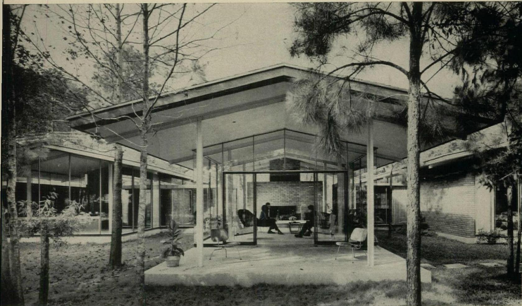
In living pavilion, center, transition between outdoors and indoors is scarcely noticeable. Roof is floated on 4" WF rigid frames, 12' oc and spanning 11'.
