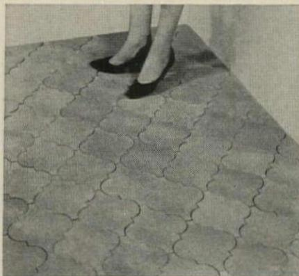
**Shaped quarry tile** are used to give a new floor texture. New thin unglazed tile, called Contour, are 7" x 8" but only a nominal ¼" thick. Tile come in two earth colors—cimarron red and cork finish. They can be set in conventional or thin-set mortars.
