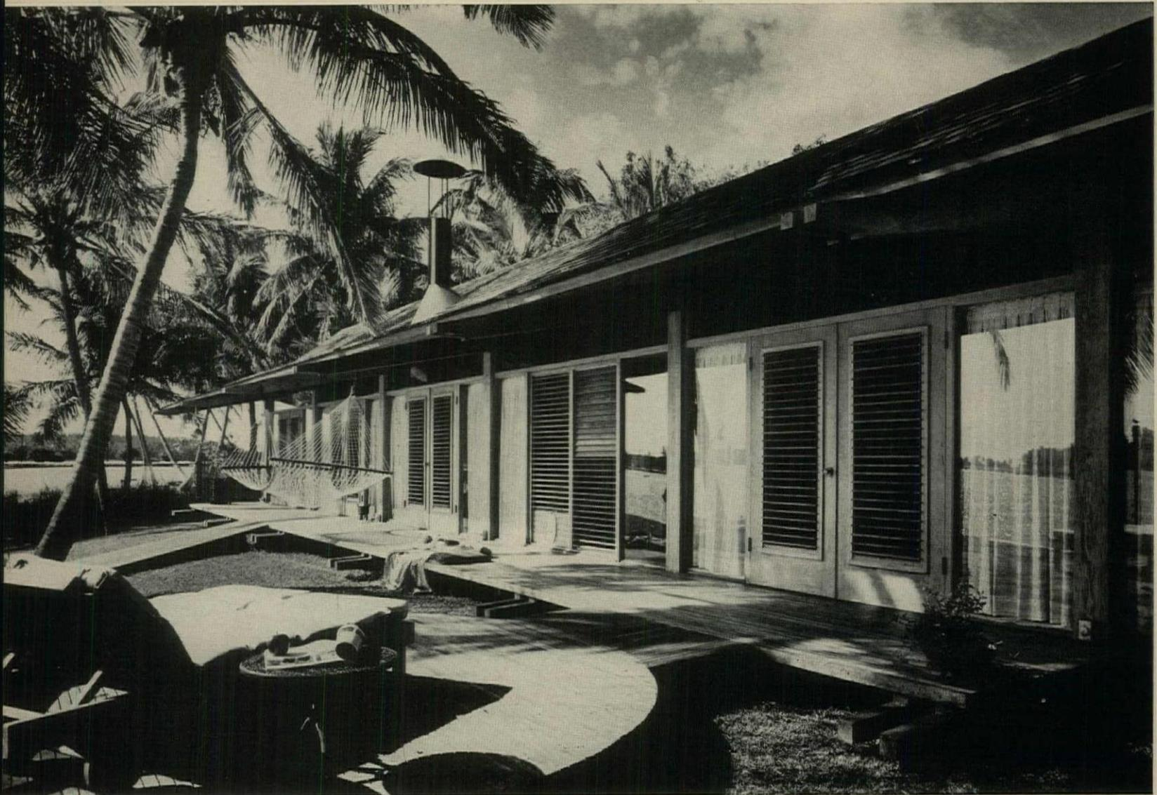
House floats just above grade, supported on 12 piers. It seems wider than its 17' because of the 5½' cantilevered deck and 8½' overhang.
