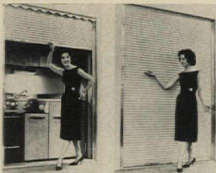
**Roller kitchen door** separates cooking from living areas in small apartments. Jamb-to-jamb panels are aluminum, coated in a variety of colored enamels. Nylon bearings and insulated tracking eliminate metal-to-metal contact. Roll-up spring at the head gives fingertip operation. Sizes from 12'x10', prices from \$49.95.
