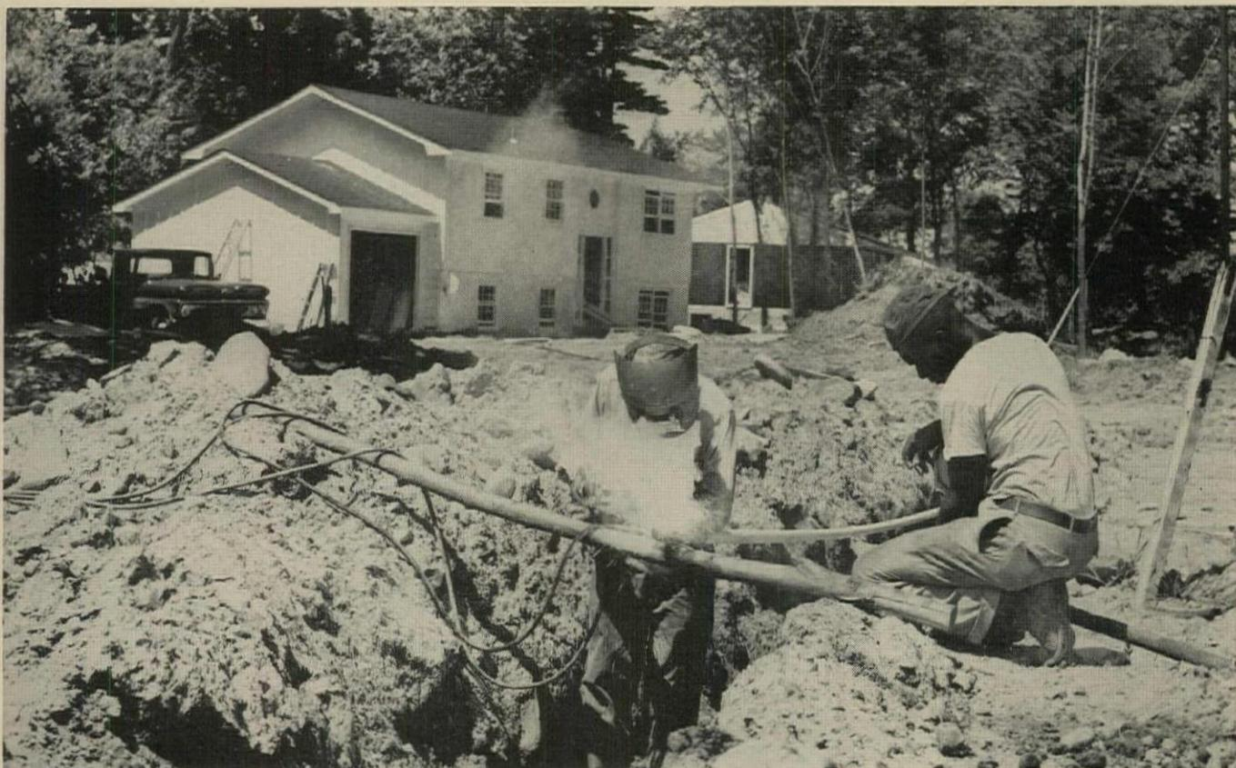
PLASTIC-COATED STEEL PIPE leading from nearby storage tank will carry fuel oil to a group of 47 new houses in Poughkeepsie, N.Y.
