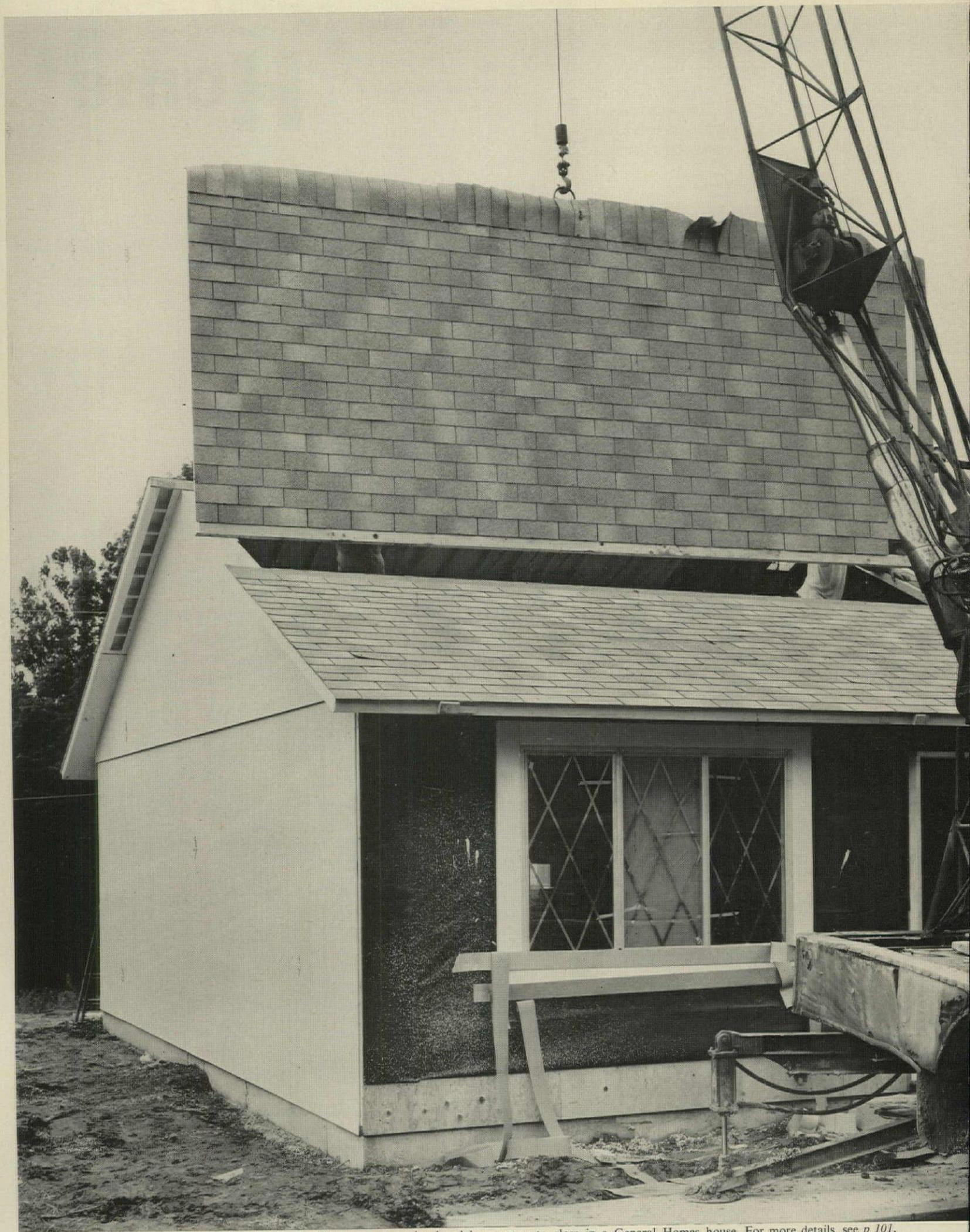
**FACTORY-ASSEMBLED ROOF SECTION** is placed by a crane to close in a General Homes house. For more details, see *p 101*.
