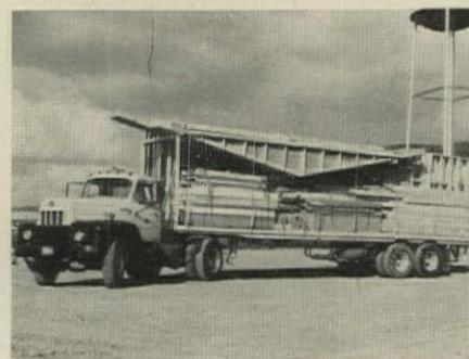
The smaller photos at the right show both sides of a loaded truck without its tarpaulin. This load arrangement allows parts to be taken off in sequence and moved directly into position—nothing is stacked on the ground. Final finish materials—the last items off the truck—are stored inside the house shell when it is locked up at the end of the first day. /END
