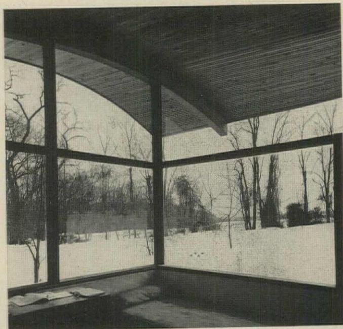
Structure is post-beam, with no bearing walls. Roof deck of fir 2x3s spans from outside, curving beams to a straight center beam (see right).
