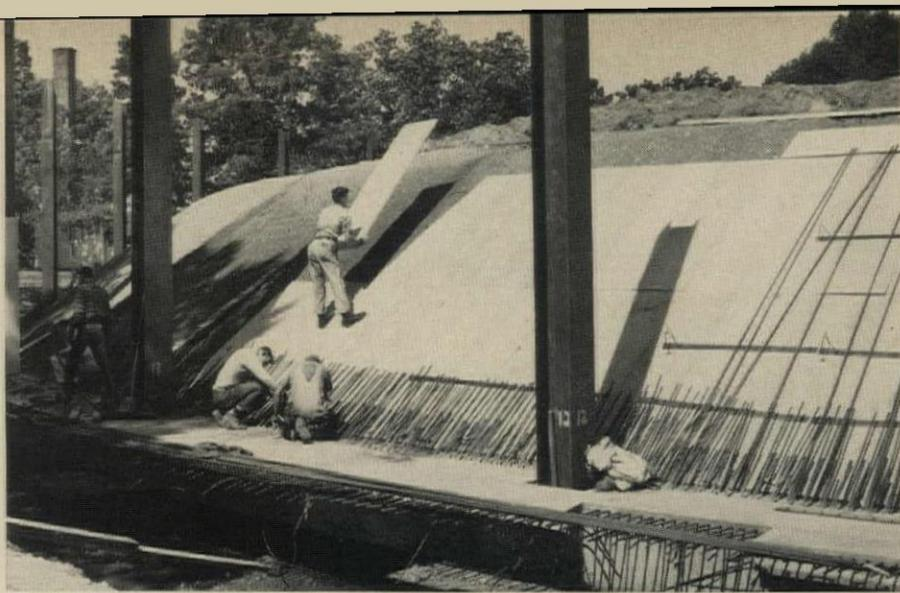
**POLYSTYRENE FOAM SLABS** are laid on gravel, are followed by reinforcing.
