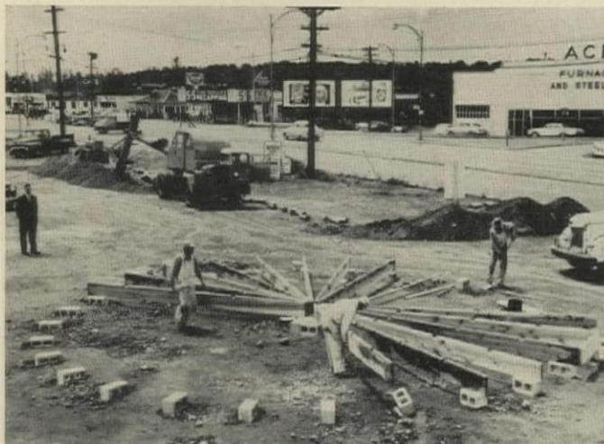
**FLOOR JOISTS** are laid out on block foundation. Floor panels will fit into notches and rabbets on top of the 2x12s.
