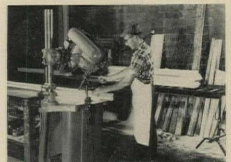
**Radial drill press** is low-cost, medium-duty tool for construction and building trades. Maker claims three special virtues: 1) the tool moves, not the work, 2, it has large capacity, 3) it is portable. Drill moves up and down, in and out, swivels 360°, tilts 45° left or right. Price: less than \$350.
