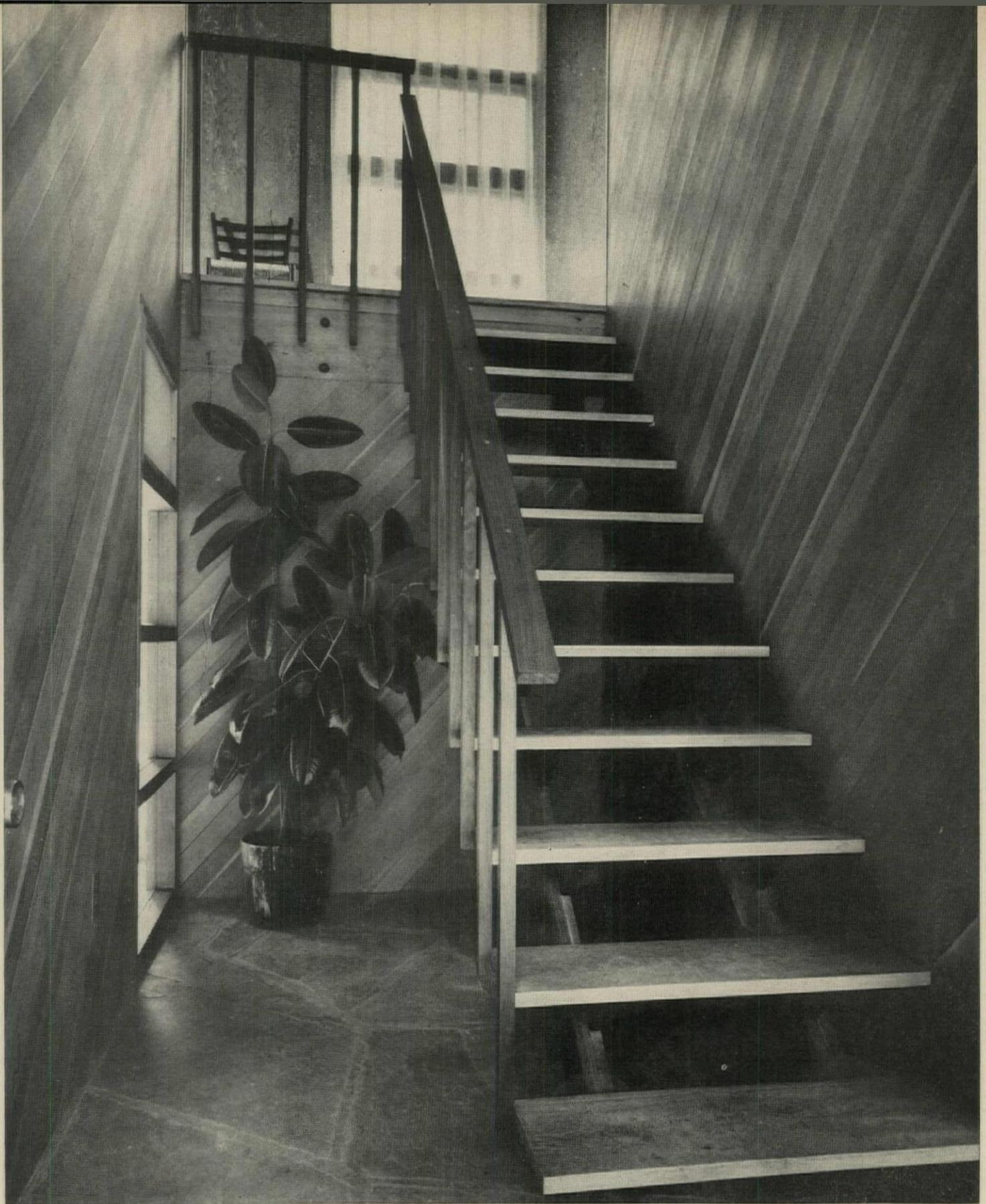
In entry core, gracefully detailed staircase leads up to living area. Diagonal siding is fir. Utilities are beyond wall at right.
