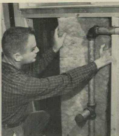
Slips easily behind pipes or wiring. No vapor barrier to catch and tear.
