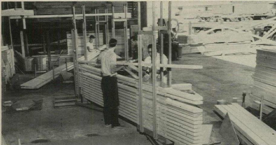
**PLYWOOD GUSSETS**—in pairs with unglued sides back to back—are laid in jig between truss framing members. Parts are simply stacked up until jig is full.
