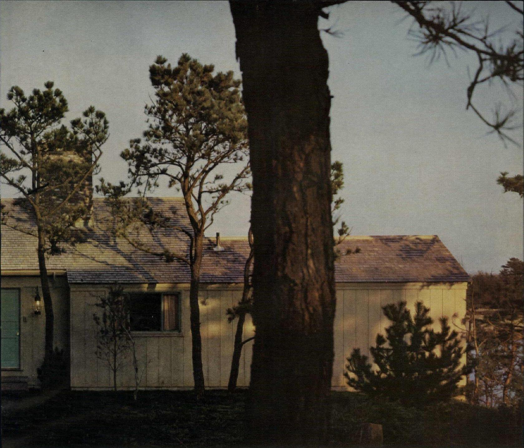
**FRONT ELEVATION** has the familiar silhouette of a Cape Cod cottage but the siding is unpainted rough-sawn cedar with reverse battens.
