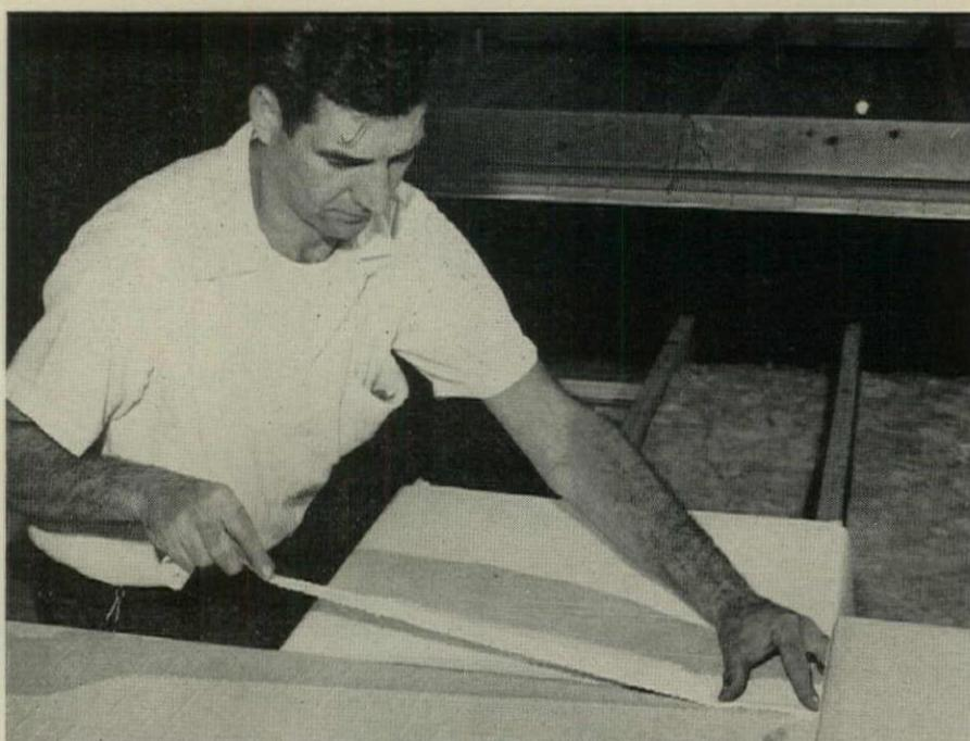
**JOINTS** between duct sections are coated with adhesive, held together with tape.
