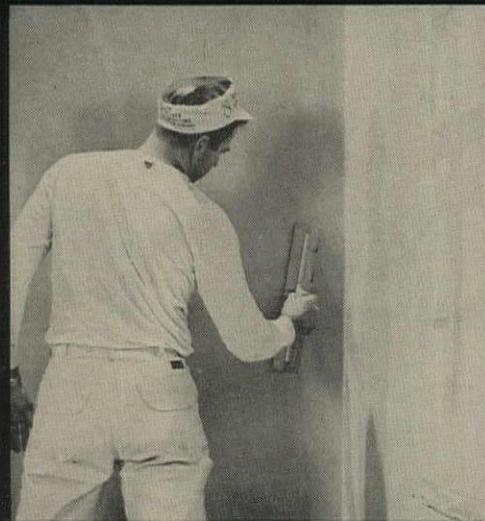
Troweling can be done right after spraying. In less than a day, the job is done.
