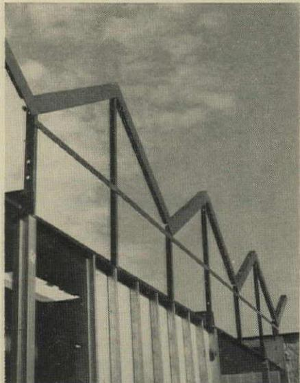
5 Roof frames to carry folded-plate roof are bolted to side of center core.
