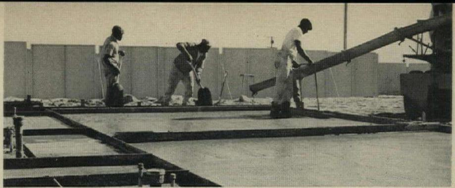
2 Slab is poured with template in place; template will be removed when concrete sets up. Area at left, with rough plumbing, will be under the center core.
