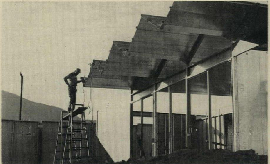
6 Folded-plate roof is assembled over living area. Insulation will be laid in channels between folded panel edges. Steel skin goes over insulation, gets spray finish.
