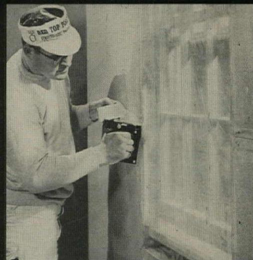
Specially formulated glass fiber tape is quickly stapled in place over joints.
