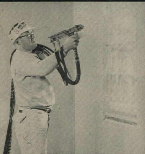
Thin coat of TUFCON Finish is sprayed over tape and wall, ceiling surfaces.
