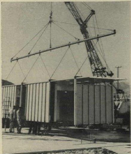
3 Pre-assembled center core is dropped onto slab by crane with special yoke.
