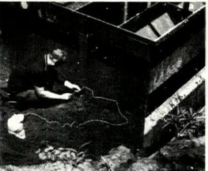
Magnesium anodes and epoxy coating protect the plant from corrosion...
