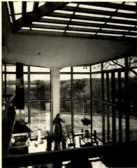
**LIVING ROOM** interior shows convex ceiling, post encased in plaster, center skylight roof.
