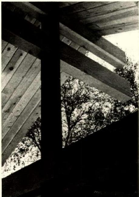
**DETAIL** shows framing at point where pitch roof over living area intersects flat walkway roof. Top 4x8 is roof ridge; bottom 4x8 was added for additional design interest.
