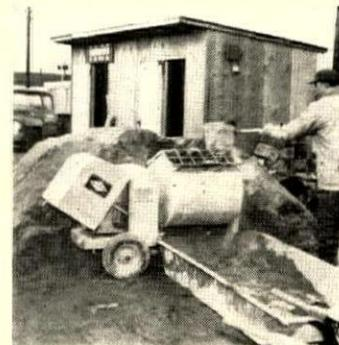
**Utility mixer** has 6 to 8 cu. ft. capacity for contractors who occasionally do big-volume work but do not need a heavy-duty mixer of this capacity. It is available with gas or optional electric drive. \$495 f.o.b. manufacturer's plant. Muller Machinery Co., Metchen, N.J.
