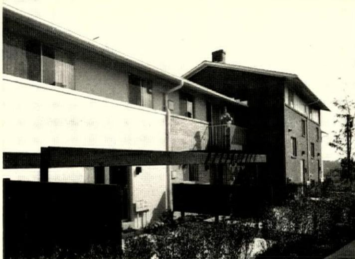
**SETBACKS** break up what otherwise might have been monotonous façades. Top floor exterior panels (above brick) are pebble-grained aluminum laminated to plywood, topped by perforated aluminum soffits.
