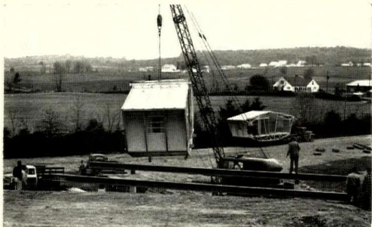
**SPACE FRAME HOUSE** by Building Components Research, Newark, Ohio is made of transverse sections that rest on steel rails (see H&H, Sept).
