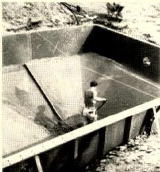
WALL PANELS bolt together, pool bottom is lined with sand.
