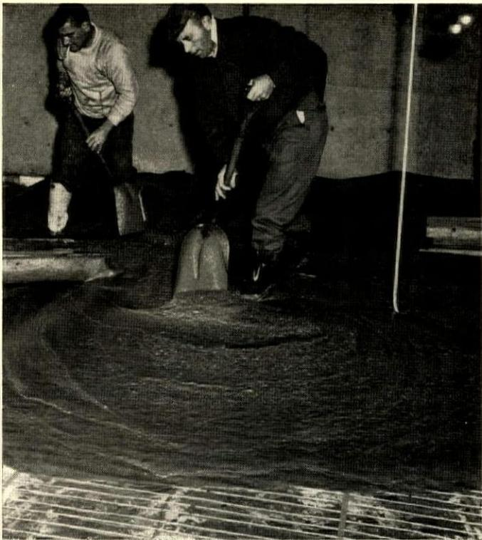
SLAB is poured over heating cables. Test lights, right, warn of breaks.
