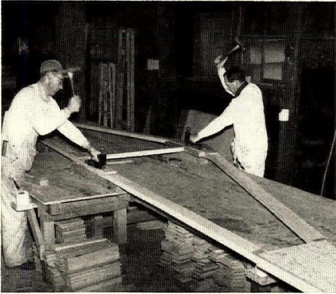
▲ **King post trusses** may have nail-glued or staple-glued plywood gusset plates (as above); or gussets may be pressure-glued; or simply nailed. They're economical because they require only half as many connections as other truss designs. Many component fabricators and lumber dealers supply king post trusses as part of a complete prefabricated house package. Some builders who have used them report savings up to \$300 a house due to use of the prefabbed components.
