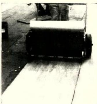
**One-ply roofing**, called "Last-O-Roof," is made of polyisobutylene welded to an elastomer-bonded asbestos support. It is applied with cold adhesive, can stand up to any climate. Johns-Manville, New York City.
