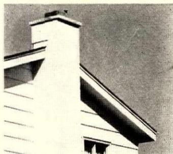
**Hardboard siding** comes as lap siding (above) 12" or 9" wide, or as V-grooved or panel siding. Called "X-ninety", it is face-primed and backsealed in the factory. Masonite Corp., Chicago.
