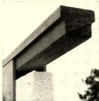
**TOP PLATE**—continuous, rabbeted, and glued snugly between skins—ties panels together structurally.
