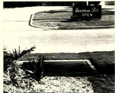
TRANSFORMER VAULTS of reinforced concrete are located at the front of property lines but are not conspicuous—and are also easy to service—because steel covers (photo above) are flush with the ground.
