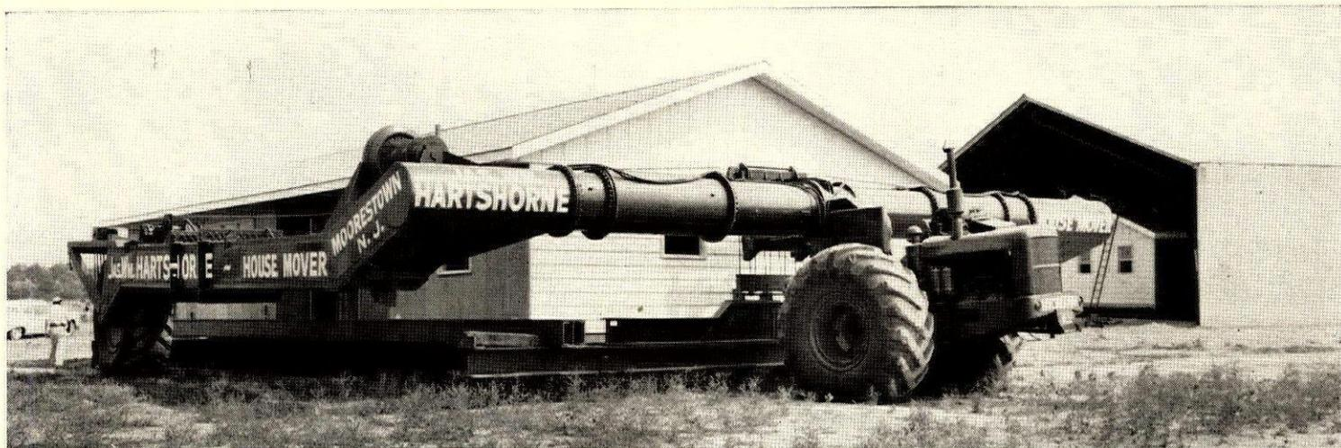
**HOUSEMOVER** is 100-ton yoke and tractor with 8' wheels. It carries house on steel cross beams at front and back. This 1,100 sq ft house sells for \$14,000.
