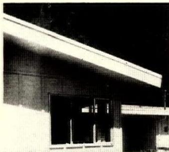
**Board-and-batten siding** is made of  $\frac{3}{8}$ " overlaid exterior plywood with two prime paint coats. Battens are available in 8', 9' and 10' lengths to match plywood sheets. Evans Products Co., Portland, Ore.
