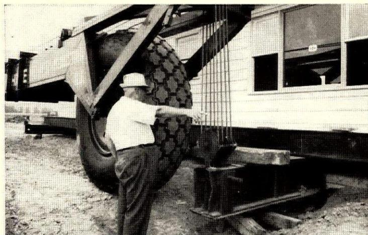
**3. LIFTING BEAM** at rear of housemover raises house, which still rests on steel channels, off I-beam dollies. Space between end-to-end dollies gives beam clearance. Housemover can lift load 4' off ground.
