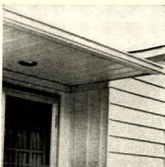
**V-groove aluminum siding** can also be used as a soffit system, as shown above, is supplied in plain and ventilated panels. It is available in white and four pastel colors. Mastic Corp., South Bend, Ind.
