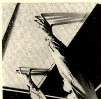
**Embossed lay-in panels** fit into a simple metal grid system. Flame-resistant panels come in 2' x 4' and 2' x 2' sizes. Luminous and acoustical panels are also available. Celotex Corp., Chicago.
