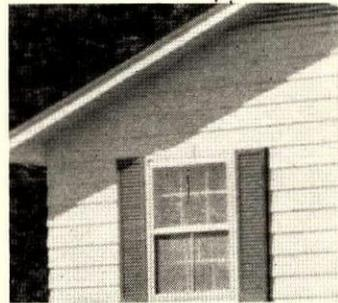
**Aluminum siding** is available with or without  $\frac{3}{8}$ " foam insulating backing. Factory finish is acrylic enamel. Snap lock joint holds bottom edge of each strip. Kaiser Aluminum & Chemical Corp., Oakland, Calif.
