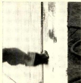
**TONGUE** of t&g panel gets coat of phenol resorcinol glue in field before adjoining panel is erected.
