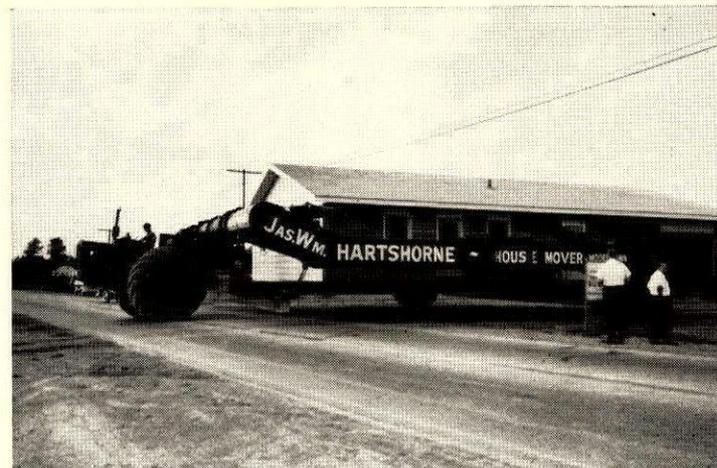
**4. LIMITED ROUTE** of housemover is across highway where phone and power lines have been raised (traffic is stopped for three minutes). Mover makes up to 20 mph, but cannot travel roads because of its width.
