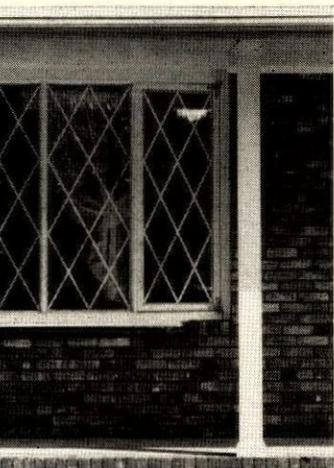
**Windor** aluminum "Bow Wall" windows can be adjusted for depth and angle during installation, have snap-on vinyl glazing beads. Sizes range from 5'10" x 4'9" to 6'3" x 13 1/4". Windor Industries, Inc., Dallas, Tex.
