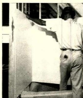
**One-piece waterproof wall** for tub-and-shower enclosure has Micarta surface, foam core, and Micarta backing. It can be installed over studs by one man in an hour. Micarta Div., Westinghouse, Hampton, S. C.
