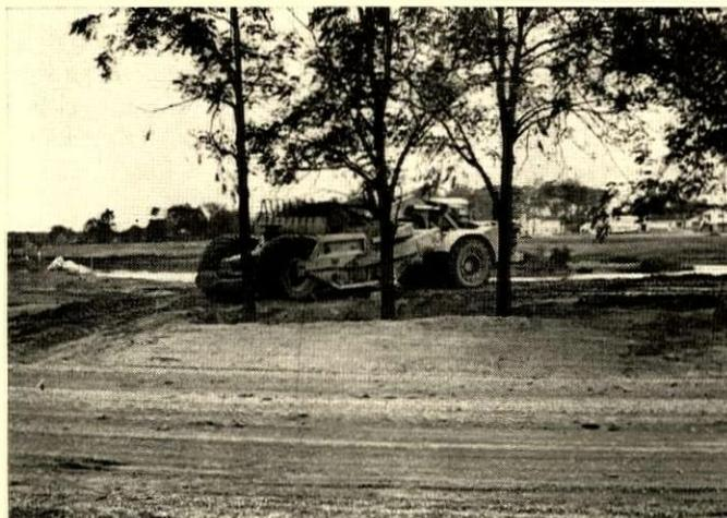
**HUGE SCRAPER**, carrying fill to a low spot, carefully avoids trees that will later be welled. Water in the background forms an artificial lake created to overcome the problem of low, wet ground and to add an important attraction for houses in the \$30,000 range.
