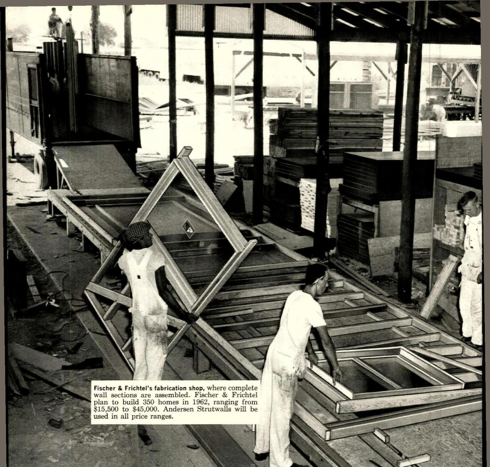
Fischer & Frichtel's fabrication shop, where complete wall sections are assembled. Fischer & Frichtel plan to build 350 homes in 1962, ranging from \$15,500 to \$45,000. Andersen Strutwalls will be used in all price ranges.
