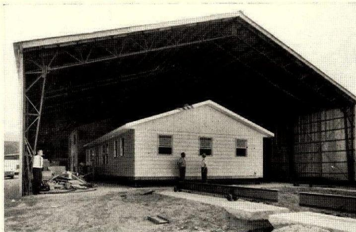
**2. FINISHED HOUSE**, still on dollies, is moved out to loading area. Space between end-to-end dollies will be directly above trench, in foreground, where lifting beam (below, left) will be placed. Factory holds four houses.
