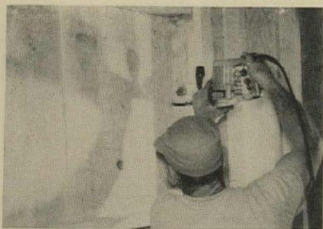
*Item:* Stanley makes an all-purpose, heavy-duty reciprocating saw (above). TAMAP engineers found it could be used to make window cutouts from the inside (through the sheathing) using the framing as a guide. This proved cheaper than using a portable builder's saw, which must be used from the outside and requires careful measuring to locate the openings under the sheathing correctly. During the study, the plumbing crew spotted the saw
