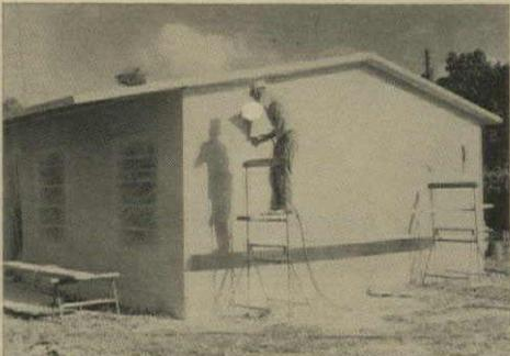
**PERMANENT FINISH** is sprayed on exterior of house after roof panels have been glued to walls.
