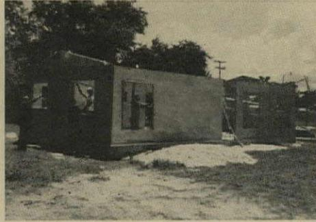
**WINDOW OPENINGS** are cut in 3"-thick wall with router and split-jamb frames installed.
