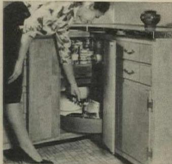
**Revolving corner shelves** are 32" in diameter, occupy 36" x36" corner area. Super Susan shelves revolve independently on bearing races, are supported by a steel frame (left) and can be used with any cabinet fronts. Murray Equipment, York, Pa. For details, check No. 7 on p. 182
