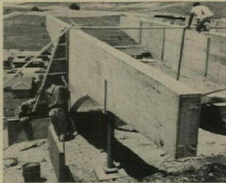
Triangular lateral braces, over wall, and pipe columns, foreground, carry no load. They resist horizontal forces, unequal loading, and rotation.
