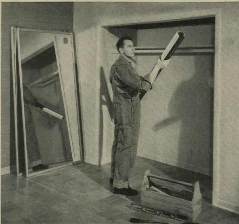
2. Install track. Track is simply screwed to head. Track and finished fascia (in anodized finish to match door) are a one-piece extrusion.
