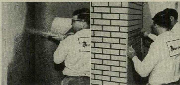
Brickstone compound is applied to the prepared wall with a Dyno-blast gun—first the mortar joint layer, and then the Brickstone finish layer of the desired color.
