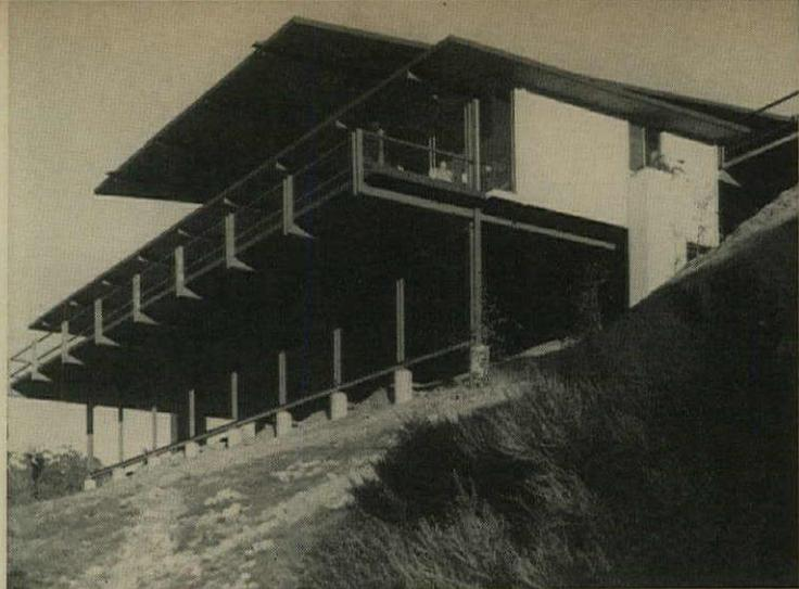
Uphill view shows simplicity of steel framing and foundation piers and deep (10') cantilevering of the 80' deck. Lower level can be converted to living space or finished as a sheltered patio.
