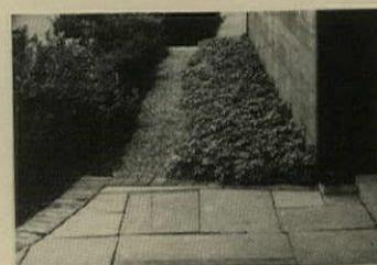
**GRAVEL STRIP** below roof drip line prevents washout of plants.
