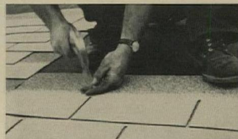
smoother. Roofers hold the nail between two fingers (above) and complain that the rougher American nails scratch their skin painfully in the course of a day, and are harder to drive (because of uneven length) without occasionally banging a finger.
