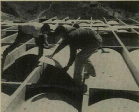
Plywood soffits are sprung between 2x6 blocking to produce a vault effect, and create a space for utility lines and insulation.
