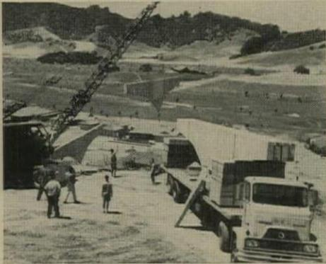
Crane placed seven foundation beams in less than two hours, at a cost of \$67.50. Glue-nailed in the factory, beams were trucked to the site.
