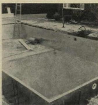
**Swimming pool** of 2"-thick aluminum sandwich panels is assembled in an excavation. Package includes steel channel, vinyl liner, aluminum coping, plumbing and filter system. A 16' x 32' pool costs \$995 as a kit, \$1,995 installed. Trojan Pools, Troy, N.Y.
