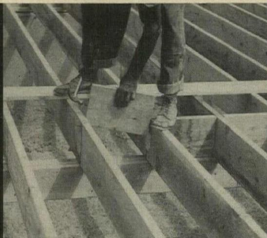
Block bridging placed between joists directly over the center beam is the only bridging needed with UNICOM to assure strong, straight floors in your house.
