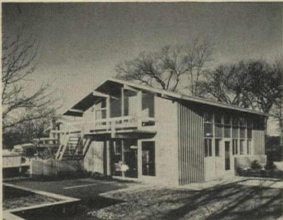
**ORIGINAL 1953 TECHBUILT** was a split-entry with 1,800 sq. ft. which could be arranged in a variety of plans.
