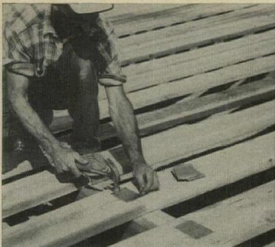
End-to-end joists join over the supporting beam's center to eliminate wasteful overlap, provide uniform spacing for UNICOM's modular subflooring or decking.
