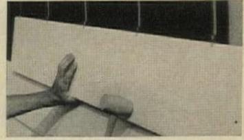
Metal fastener strips are nailed to sheathing (left), siding is slipped under tabs (center) and driven against anchors.
