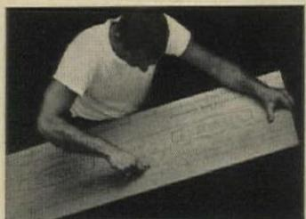
**Gypsum lath** has a nonfading printed surface with guide lines for accurate scoring and nailing. "Pinolath," insulating, and perforated types are reinforced with glass fiber, have absorbent face paper for rapid plaster takeup. Bestwall Gypsum, Ardmore, Pa.
