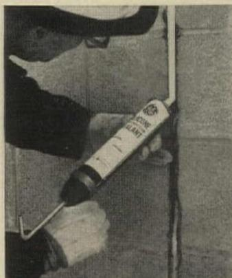
**Silicone sealant** for curtain-walls, precast concrete, expansion joints, and window glazing is applied from a caulking gun without mixing. It resists temperatures to 250F, can be applied in below-zero weather. \$26 a gal. in bulk. G. E. Waterford, N.Y.
