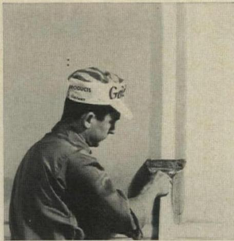
**TAPE BEDDING** is done with hand knife: fast drying material may clog automatic equipment.
