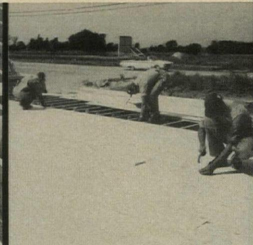
UNICOM board subflooring, delivered pre-cut to standard uniform modular length, is quickly and accurately laid down to provide you with a sturdy, lasting deck.
