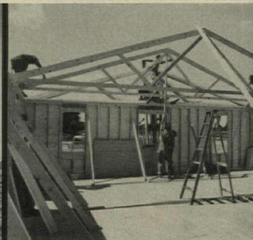
A notched gin pole moves a truss into position for the UNICOM house. W trusses provide free-span area below, obviate load-bearing interior partitions.
