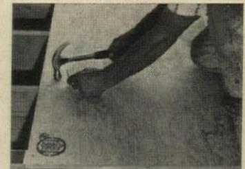
**Floor underlayment**, a sheathing-grade plywood, has a solid veneer sheet under the face veneer. Since there are no voids under the face veneer, damage from spike heels and heavy furniture is eliminated. Vancouver Plywood, Vancouver, Wash.
