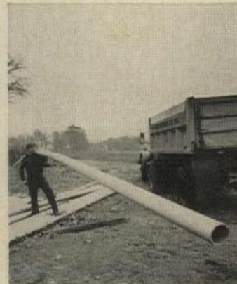
**Rigid PVC pipe** combines high strength, impact, and chemical resistance. Used for electrical conduit, oil, gas, water, and chemical lines, the pipe and fittings come from 1/4" tubing to 12" diameter pipe. Barrett Div., Allied Chemical, New York City.
