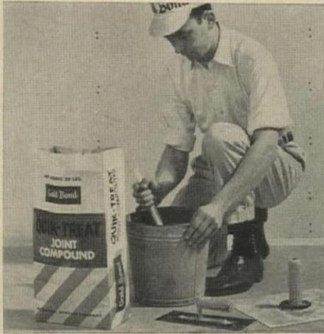
**MIXING** is done in clean, drinkable water. Water cannot be added if material starts to thicken.
