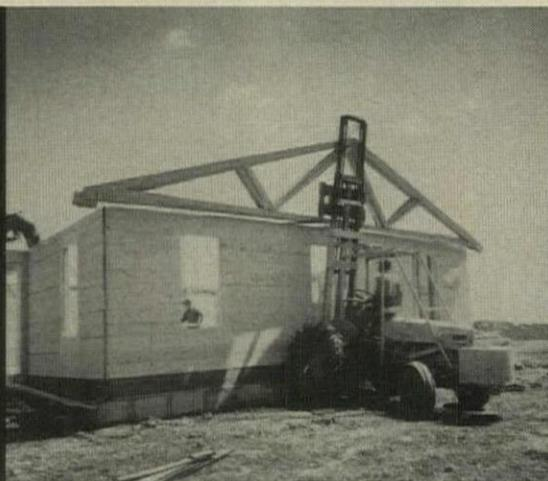
Trusses are raised to position as needed with a fork lift. UNICOM-coded trusses are keyed to working drawings for speedy placement. Wall elements are coded, too.
