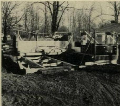
**BACKFILL** is graded around foundation so core can be rolled right up to wall.
