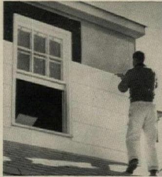
**Vinyl siding** has a ten-year, maintenance-free guarantee. IVBS is applied without special tools (package includes all accessories). Styles: horizontal lap 12" wide and 16" long, vertical panels 4'x8' and 4'x9'. Four colors. Insulite, Minneapolis.
