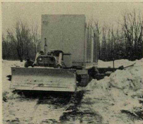
**INSTALLATION** starts when dozer or truck tractor backs core up to the foundation.
