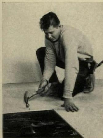
**Flakeboard underlayment** is available in 3/8", 1/2", 5/8" and 3/4" thicknesses, can be used under tile, sheet goods and carpets. It complies with FHA UM-28 floor underlayment specs and with CS236-61. Collins Pine Co., Chester, Calif.
