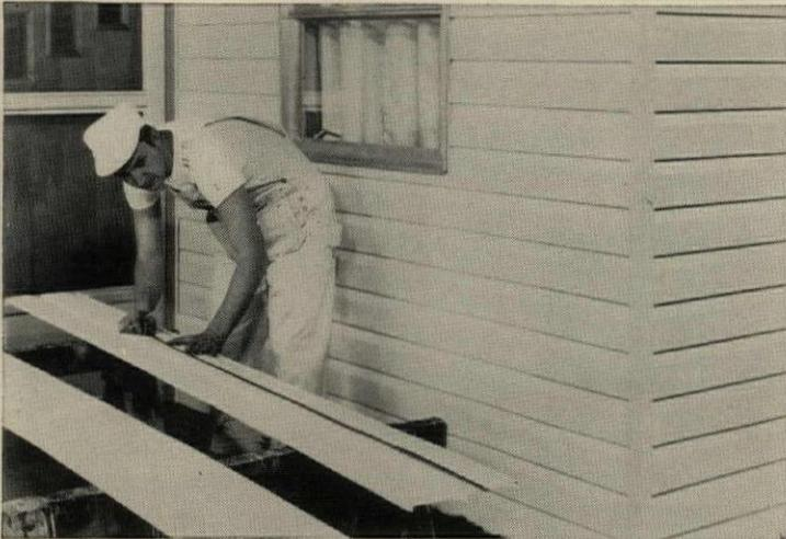
**Aluminum lap siding** is shaped so its surface is parallel to the wall rather than slanted, cutting dirt accumulation and still giving a shadow line. Double Five has two 5" clapboards to each 10"x12' piece. Alcoa, Pittsburgh. (For details, check coupon No. 20 on p. 198)
