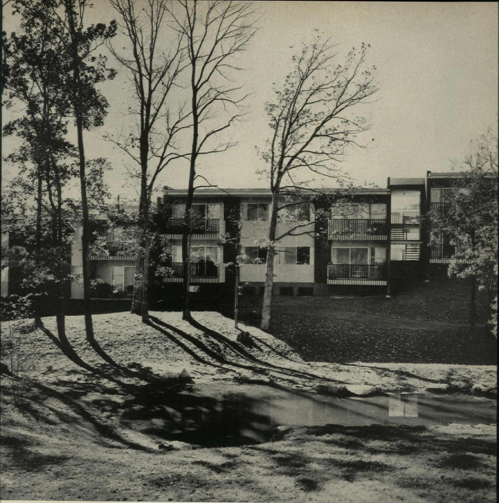
**STEPPED-DOWN ELEVATIONS** matched buildings to grades, kept earthmoving to a minimum. Pool is part of a watercourse in the middle of the site.
