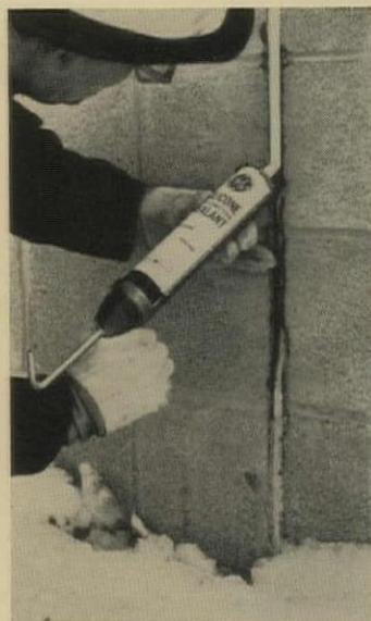
**Silicone sealant** for expansion joints, glazing and caulking costs about two thirds as much as similar industrial products. It can be used at sub-zero temperatures, cures to form a durable seal that remains flexible. G. E., Waterford, N. Y. (For details, check No. 22 on p. 203)
