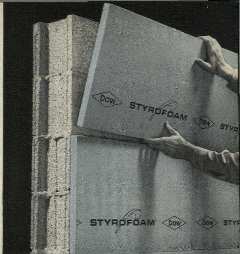
**4. Press Styrofoam FR into place. It installs fast, resists heat transfer, stays dry for year-round comfort.**
