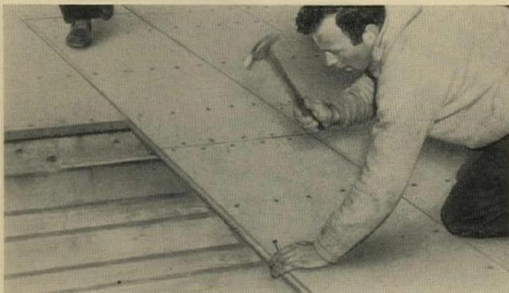
**Double-thick decking** combines sub-floor and underlayment in a single 1 11/32"-thick panel. Four-way nails directly to joists, serves as base for tile or carpet. T&G panels measure 2' x 8'. Homasote Co., Trenton, N. J. (For details, check No. 19 on p. 203)
