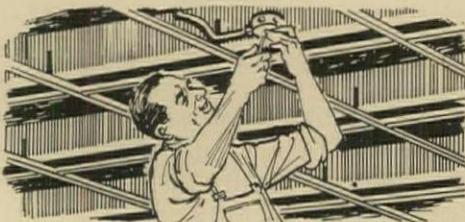
Easy leveling hanger system requires no support between 4' centers, snaps into grid in a second. Interlocking connections require no tools or time consuming fitting, just a twist of the wrist and they are securely fastened.
