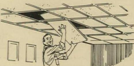
The inherent flexibility of the Simpson grid system allows use of a wide variety of inexpensive lighting fixtures or diffusion panels, heating or air-conditioning systems and provides easy access for maintenance.
