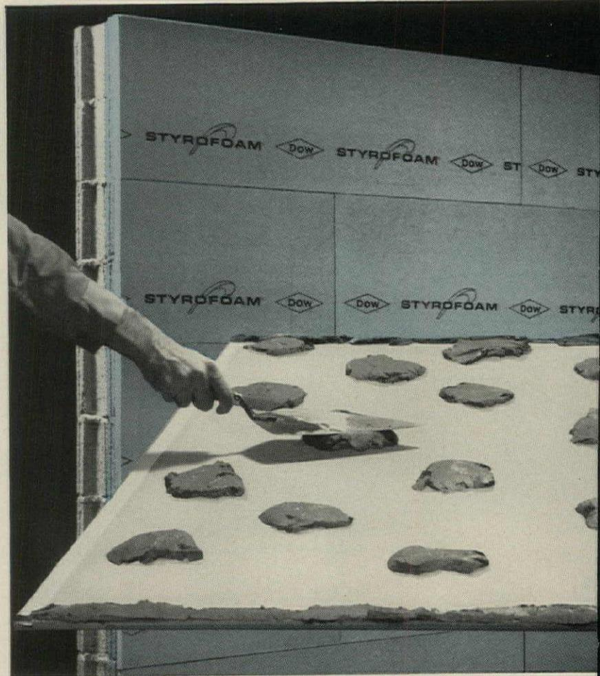
**6. Apply Styrotac—no nails to “pop,” no holes to fill.**
