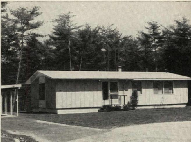
**4. ROOF PANELS** (4' x 15'), stored in attic during transport, are set in place by hand. Shingles or roll roofing finish the job.
