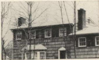
The chimneys on the house above are better than most but they still miss the mark on three counts: 1) they are too narrow, 2) the top two brick courses project and 3) the flue liners stick up above the top. "You can use full-sized chimney pots," says Thompson, "but keep flue liners flush."
