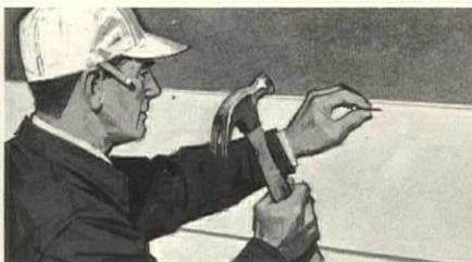
**NAIL ALONG TOP EDGE.** Siding won't split; vinyl color-coat won't chip. Nails easily, firmly. When complete siding job is done, nails won't show.
