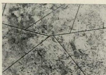
**Concrete floor-finish** is pre-packaged with graded aggregates that simulate color and texture of natural keystone. Keystone is dusted on concrete before troweling. It can be used indoors or out. Lambert Corp., Orlando, Fla.
