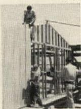
May be used for board and batten, flat panel or lapped siding. Ideal for accent paneling under windows, etc. Use panels  $\frac{3}{8}$ " thick for direct application to studs,  $\frac{5}{16}$ " over sheathing. Smooth surface requires only primer plus finish coat of any good quality house paint. Special architectural enamels may also be used. Prime back and edges where possible.
