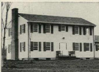
The under-6" pitch on the roof of the house above lacks mass, and the roof overhang is both non-authentic and too small to offer any protection. The 9"-pitch on the Thompson-designed house at the right is in scale and the gutter cornice is both more colonial and less expensive.
