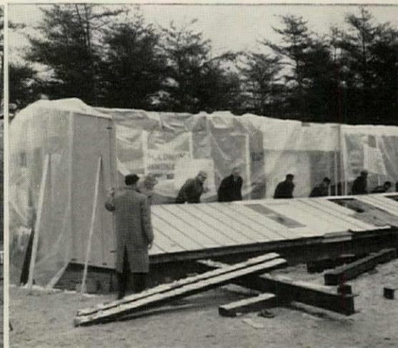
3. **SIDE WALL**, hinged to floor, is raised by workers after they have first swung out end-wall sections and then unfolded floor sections.
