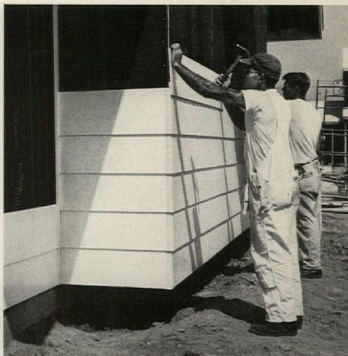
**TEDLAR\* PVF film** is a tough new film-finish—not a liquid or a spray. TEDLAR is factory-bonded with special Du Pont adhesives to wood or metal, actually becoming part of the material it protects.
