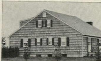
Shingles can be exposed more than clapboards, but the exposure on the house above—about 14"—is too much. The shingles at right are 6½" to the weather, midway in the permissible range—5½" to 7½".
