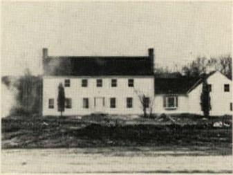
The facade above is unbalanced, Thompson notes, because 1) the upstairs windows are not aligned with the windows directly below them, 2) there are no upstairs windows above the downstairs windows at the ends of the house and 3) the windows flanking the entrance are poorly spaced. The house at right shows the result when windows are placed correctly.
