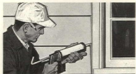
**APPLY CAULKING.** Special long-life butyl caulking in matching colors applies like ordinary caulking. That's it. Complete exterior wall is up fast!
