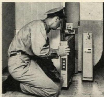
**Only 7 inches deep,** the Honeywell Electronic Air Cleaner fits easily into the duct work of any forced-air heating or cooling system. While ordinary fiber furnace filters are only 5 to 8% efficient, the Honeywell unit has been rated at up to 95% efficiency. \*(As rated by National Bureau of Standards Dust Spot Method.)
