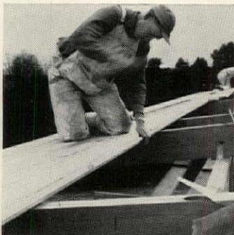
**Roof framing system** includes laminated beams and laminated roof decking. Beams are 4' x 10', 6' x 10' or 6' x 12' and from 12' to 60' long. Deck planks are 6" wide and 3", 3 1/2" or 4" thick. Edges are beveled. Weyerhaeuser, Tacoma, Wash.
