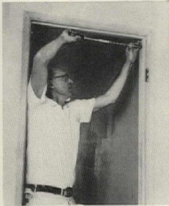
**Presto door frames** can be installed by one man in ten minutes. Presto frames have one-piece T&G construction with interlocking mitered joints. Casings, stop and hinges are factory-installed. Dexter Inds., Grand Rapids, Mich.
