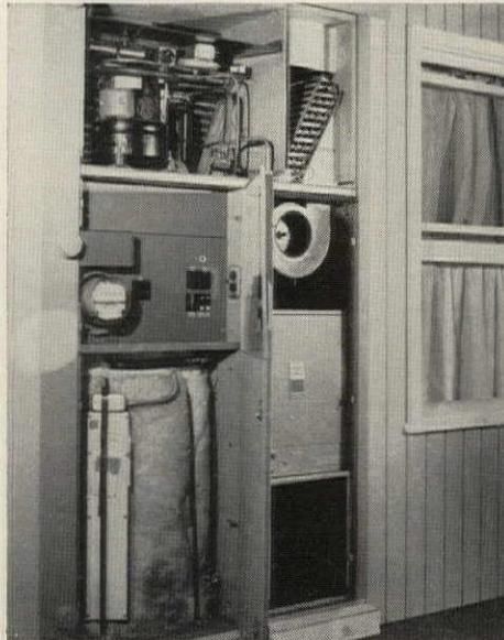
**COMPARTMENTED CABINET** houses heat pump and coils, circuit box, water heater, fan, filter.
