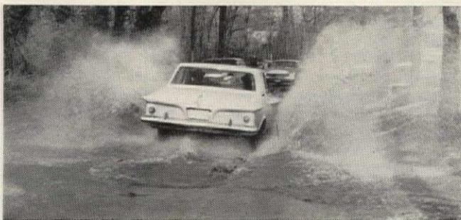
**FLOODING** results from clay soil, poor grading and paucity of storm sewers.
