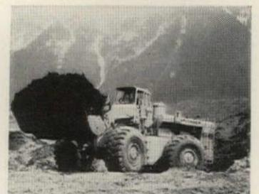
**Tractor-shovel** handles up to 30,000 lbs. with buckets ranging in size from 8 to 20 cu. yds. Model H-400 is the world's largest production model loader. It weighs 120,000 lbs. has a 180" wheel base and a 106" tread. Frank G. Hough, Libertyville, Ill. Circle 82 on Reader Service card
