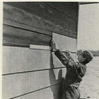
**Mineral-fiber siding** looks like wood, resists fire, warping, blistering, peeling and termites. Dura-shakes have a plastic finish that comes in five colors. They can be applied over existing siding as well as on new construction. Ruberoid, New York City.
