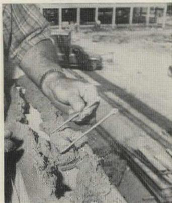
**Adjustable wall ties** permit mason contractors to erect cavity walls in two steps: 1) female ties are installed in interior wythe with eyelets protruding 2"; 2) exterior wythe is tied in with male ties. Dur-O-Wal, Cedar Rapids, Iowa.
