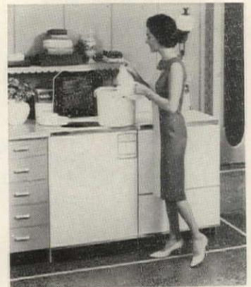
**Washer** has small Mini-basket for washing lingerie or small loads. It uses only 11 gals. of water per load. Custom V-114 washers and dryers have 14 lb. capacity, come in colors and have lighted control panels. G.E., Louisville, Ky. Circle 68 on Reader Service card
