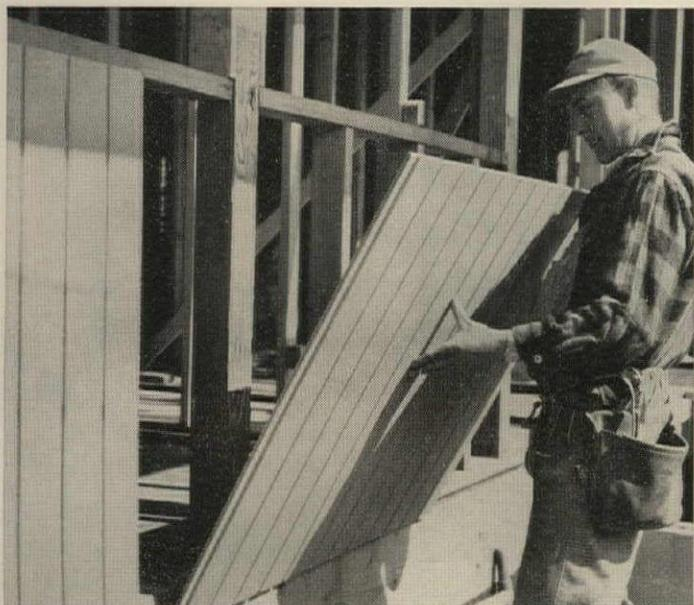
Bill Kay, White Plains, N. Y., developer, can build apartments for \$8.40 per sq. ft. because he uses low-cost, simple plywood building systems like Sturd-i-wall.
