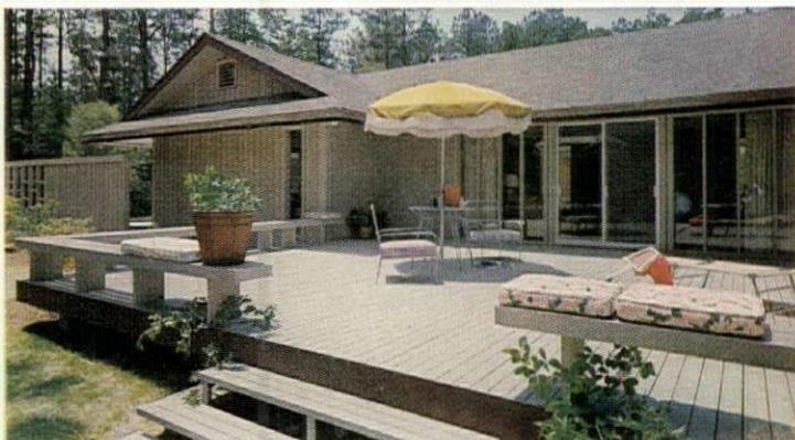
For the raised sun deck, pressure-treated Southern Pine provides lasting protection against all conditions of constant exposure.
