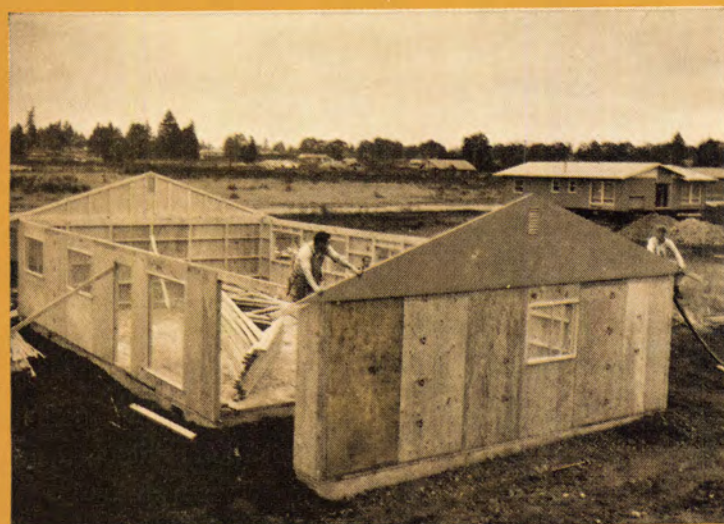
4. By 10:30 (2½ hours after the start of work) the crew is ready to lift prefabbed gable ends into position. Almost at the same time, they begin installing trusses which are waiting inside on the floor.
