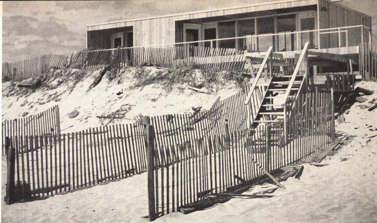
RECESSED GLASS WALLS permit sheltered outdoor living space on ocean side of house. Doors at ends of walls let sea breezes sweep through rooms (see plan below).
