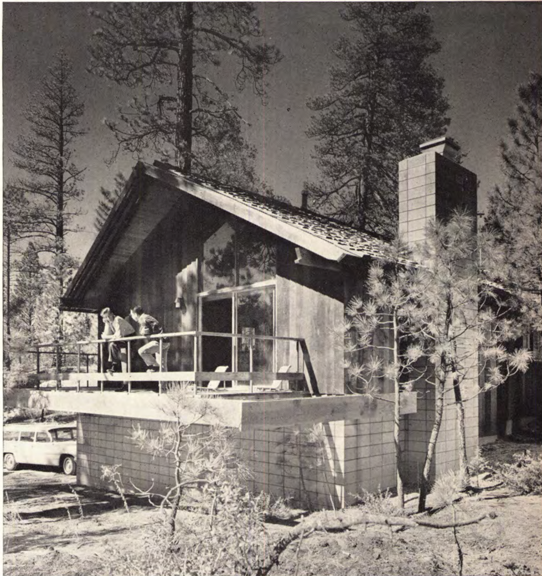
GABLE ELEVATION has deep roof overhang and deck supported by cantilevered 4x6 girders.
