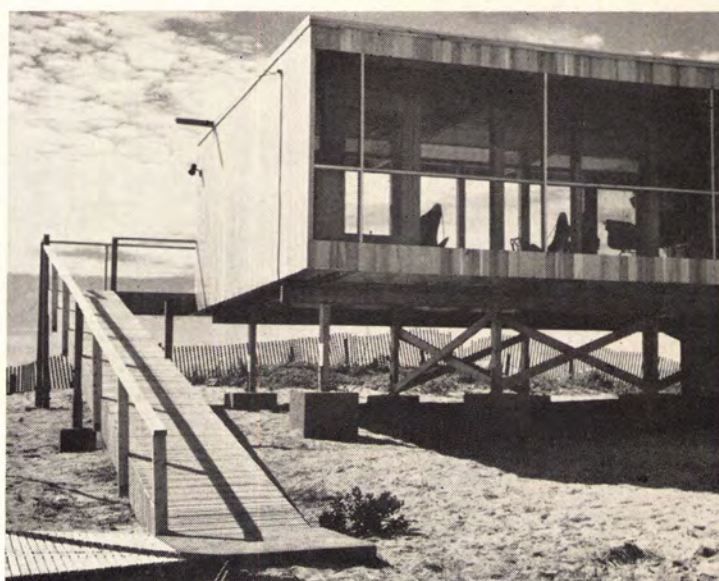
SIMPLE FOUNDATION consists of piers and posts. Cross-bracing resists racking stress.
