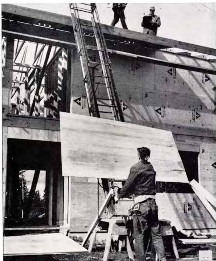
MATERIALS CONVEYOR is one of several ideas studied by APA-NAHB roof analysts in program aimed at reducing sheathing labor costs one-third.
