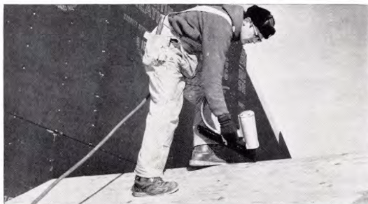
POWER FASTENER , used after all panels were positioned and tacked, saved one hour of labor on 2,000-sq.-ft. roof compared with hand nailing.
