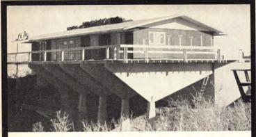
HILLSIDE LOTS — This home has a substructure of five inverted wood girders, each composed of three Sanford trusses boxed in plywood, mounted on concrete piers. Savings in labor, materials and site grading enabled the builder to use this steeply-sloped lot efficiently.
