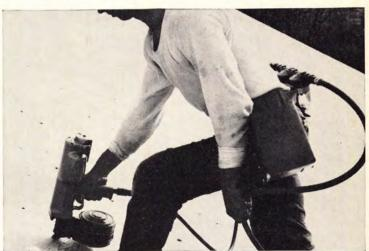
Pneumatic nailer drives 300 6d or 250 8d full-head, standard common nails without reloading. Nails are fed from a compact coil. The new nailer is called the Bostitch N2 coil-feed nailer. Bostitch, East Greenwich, R.I. (Circle 237 on Reader Service card)
